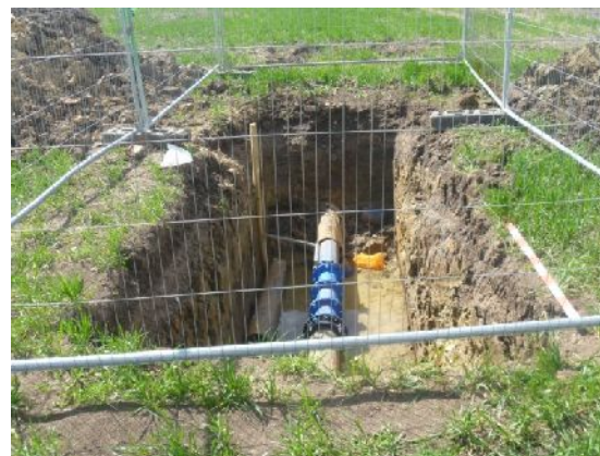
Plate 2. Test pit showing existing pipe
