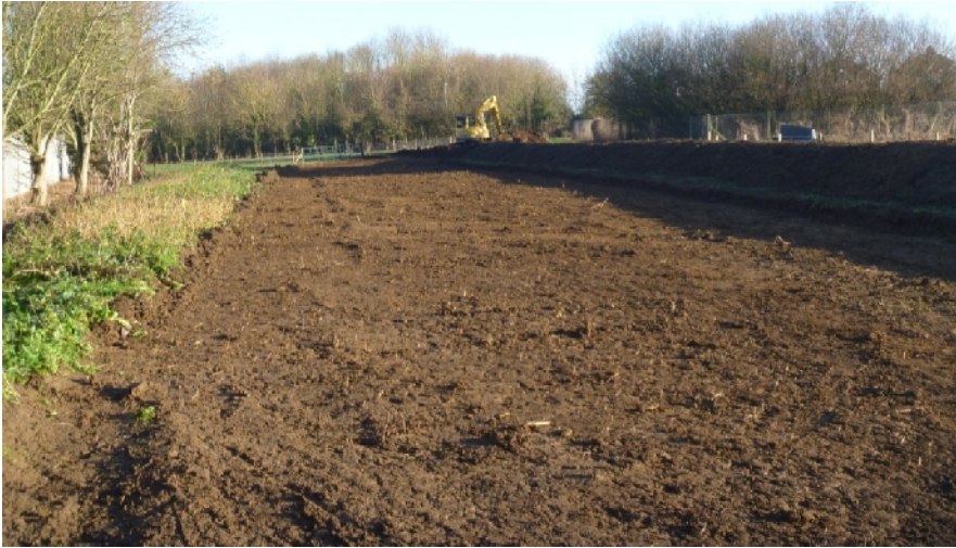
Plate 1. Field 1, after stripping of the topsoil (from ENE; no scale)
