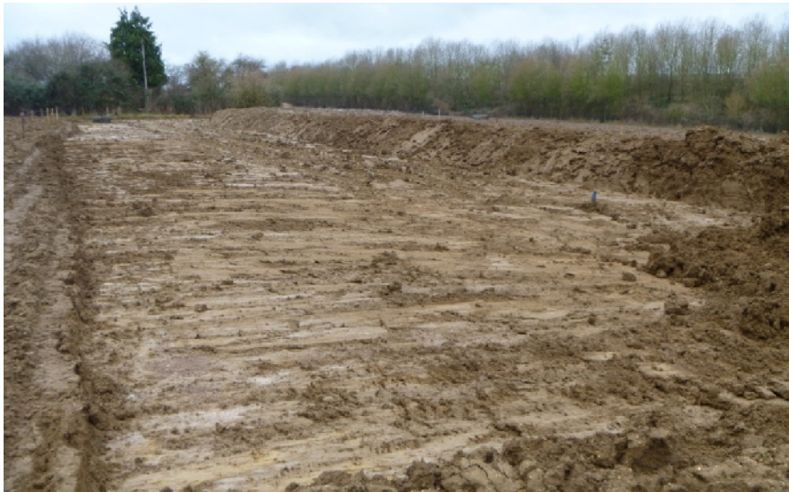
Plate 2. Field 4, after stripping of the topsoil (from E; no scale)
