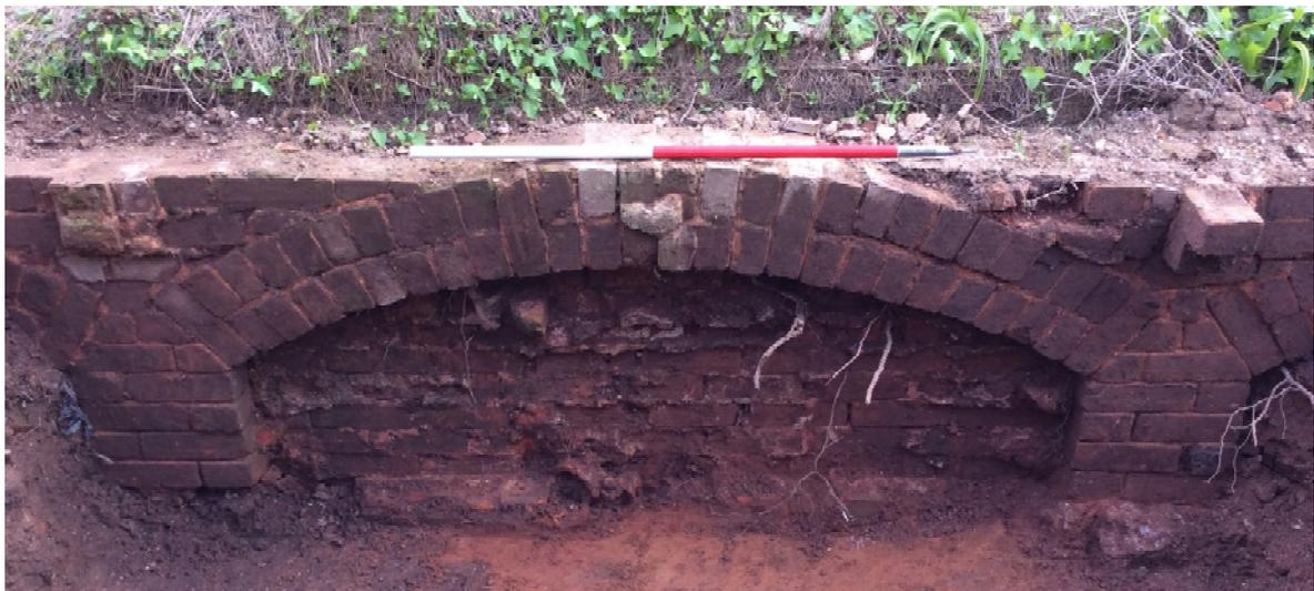
Plate 25. Vine arch in glasshouse A (inner side) showing broken central pier & corbels (1 x 1m scales; looking S)
