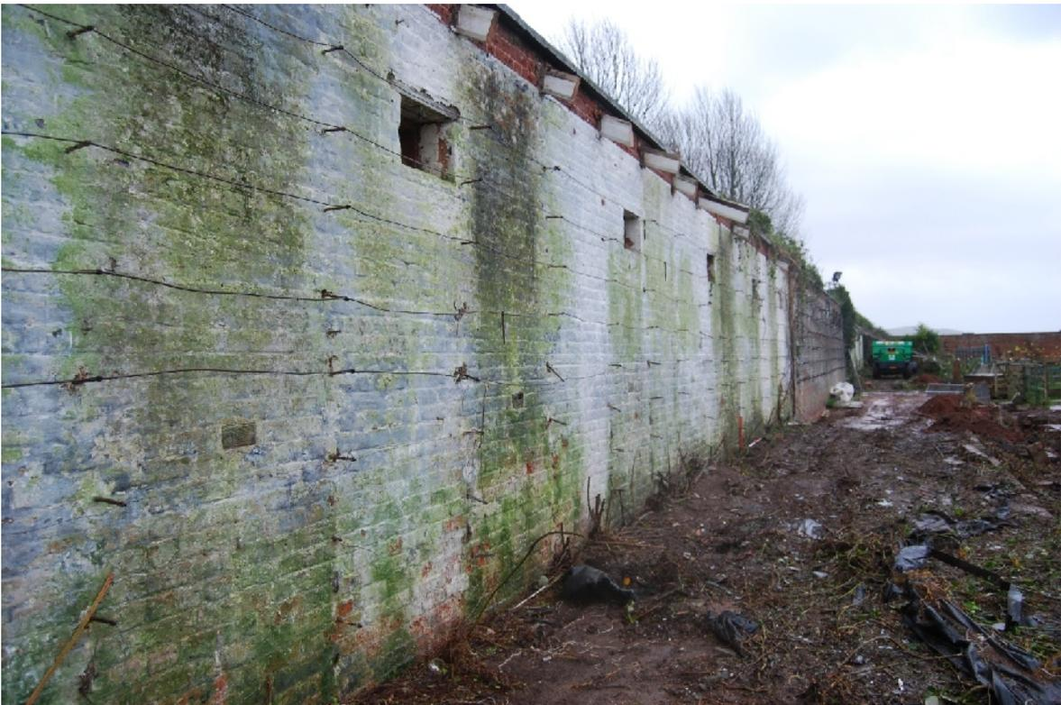
Plate 11. Vine ladders along back wall of Glasshouse A (2 x 2m scales; looking ENE)
