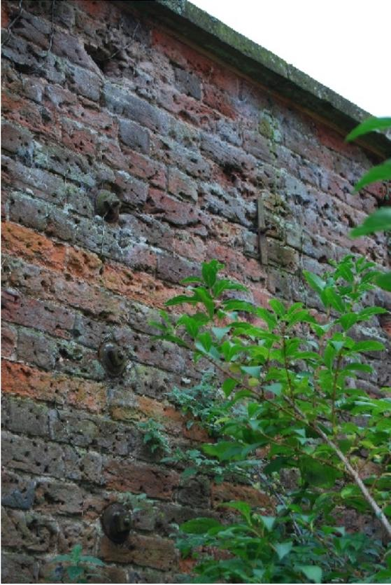
Plate 17. Vine ladder fixings in rear wall behind central glasshouse (looking SW)
