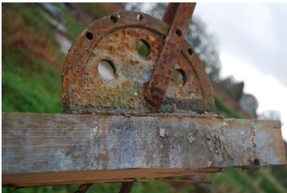
Plate 7. Close-up of gear for roof opening mechanism with stamp 'Harding' 'Torquay'
