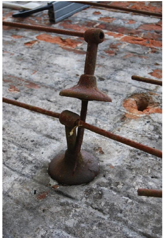
Plate 16. Fixings for vine ladders along back wall of central glasshouse
