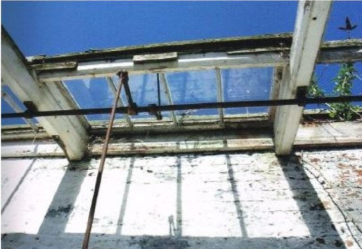
Plate 4. Window opening mechanism in roof of glasshouse B (looking N) (from Thompson 2009)
