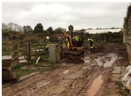
Plate 2. Excavation of exploratory trench along front wall of central glasshouse (from ENE)
