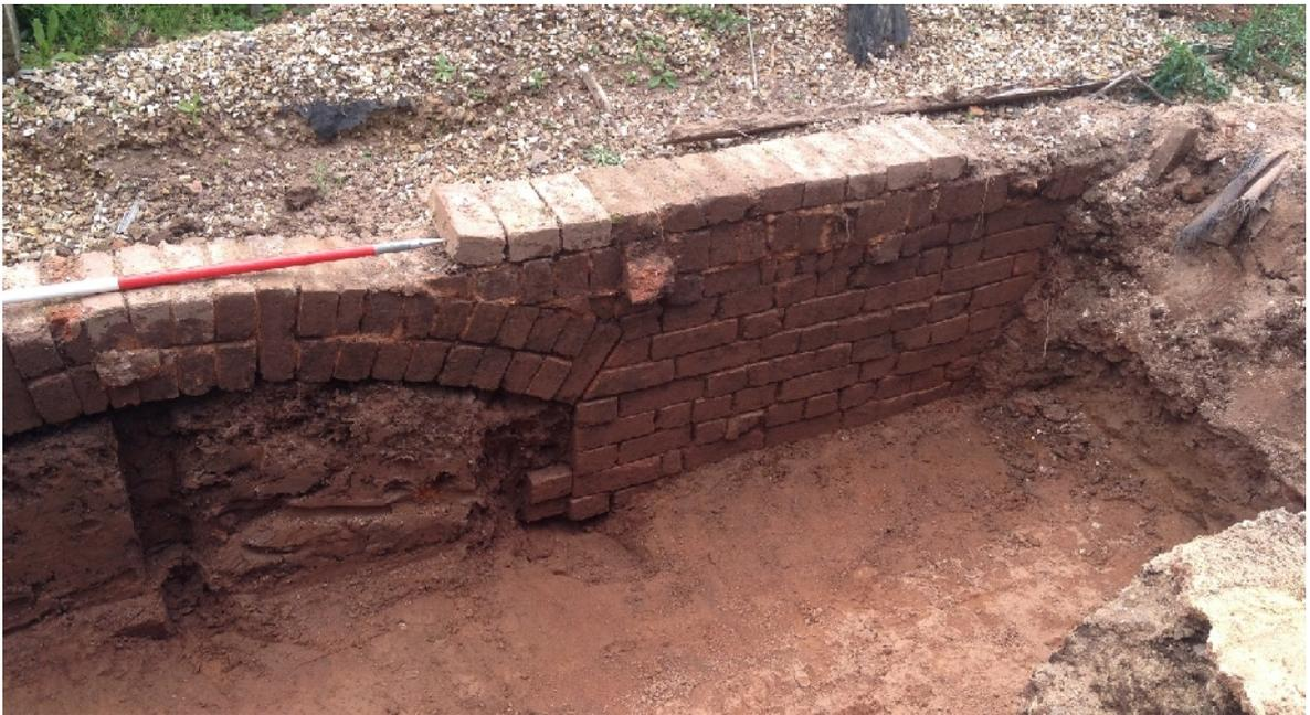
Plate 27. Solid walling between arches in central glasshouse (1 x 1m scales; looking SSW)
