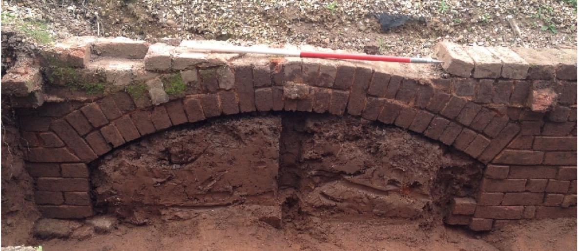
Plate 26. Vine arch in central glasshouse (inner side) showing broken central pier & corbels (1 x 1m scales; looking S)
