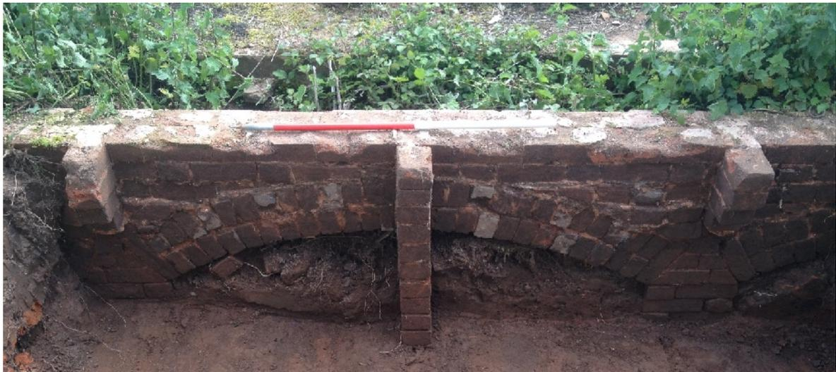
Plate 24. Vine arch in glasshouse B (inner side) showing central pier & corbels (1 x 1m scales; looking S)
