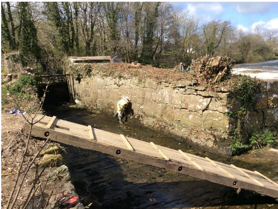
Plate 6. Pre-demolition recording of sluice north wall (from SE)
