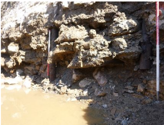
Plate 3. Timbers (103), marked by scales, within sluice stonework (104) (2 x 1m scales; from N)
