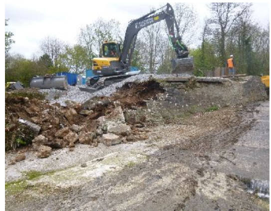
Plate 4. Removal of concrete and stonework from weir (from N)
