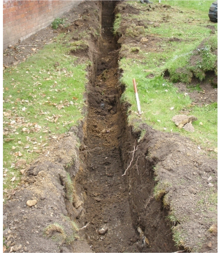
Plate 12. Area 3, service trench (from SE; 1m scale)
