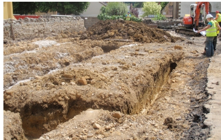
Plate 4. Area 1, general view (from NW)
