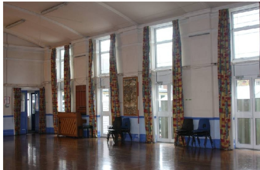
Plate 21. View across Assembly Hall full length windows (scale 2m, from NE)
