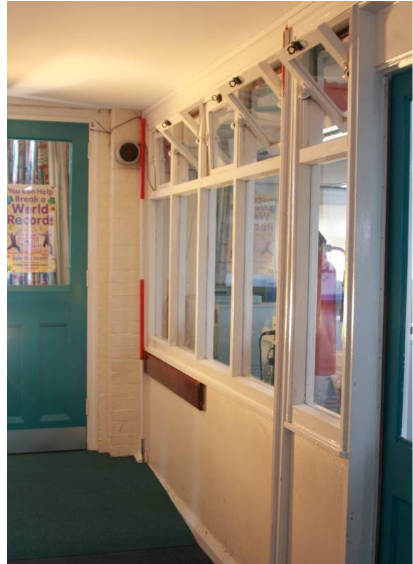
Plate 31. Original wooden window, hall approach (scale 2m; from WNW)
