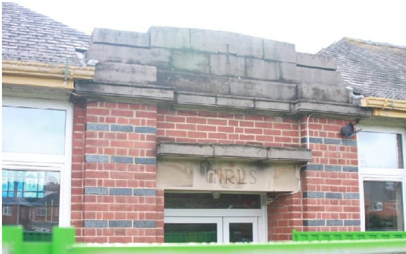
Plate 3. Western Entrance, Looking E
