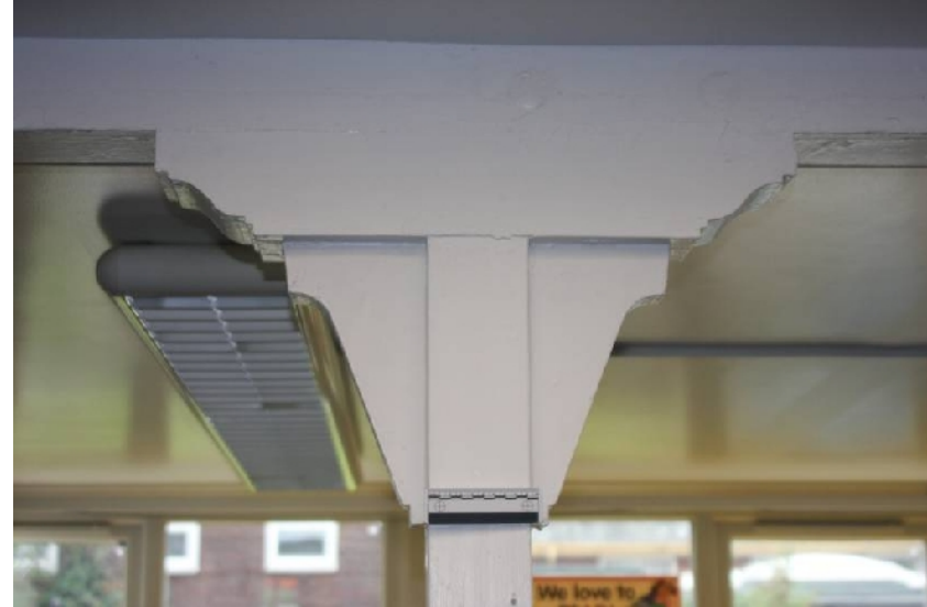
Plate 27. Detail of roof support, east corridor (no scale; from W)
