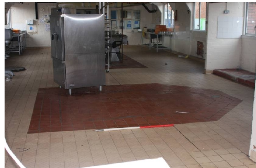
Plate 44. Kitchen Area within MOWP Hut detailing floor (scale 1m; from SW)
