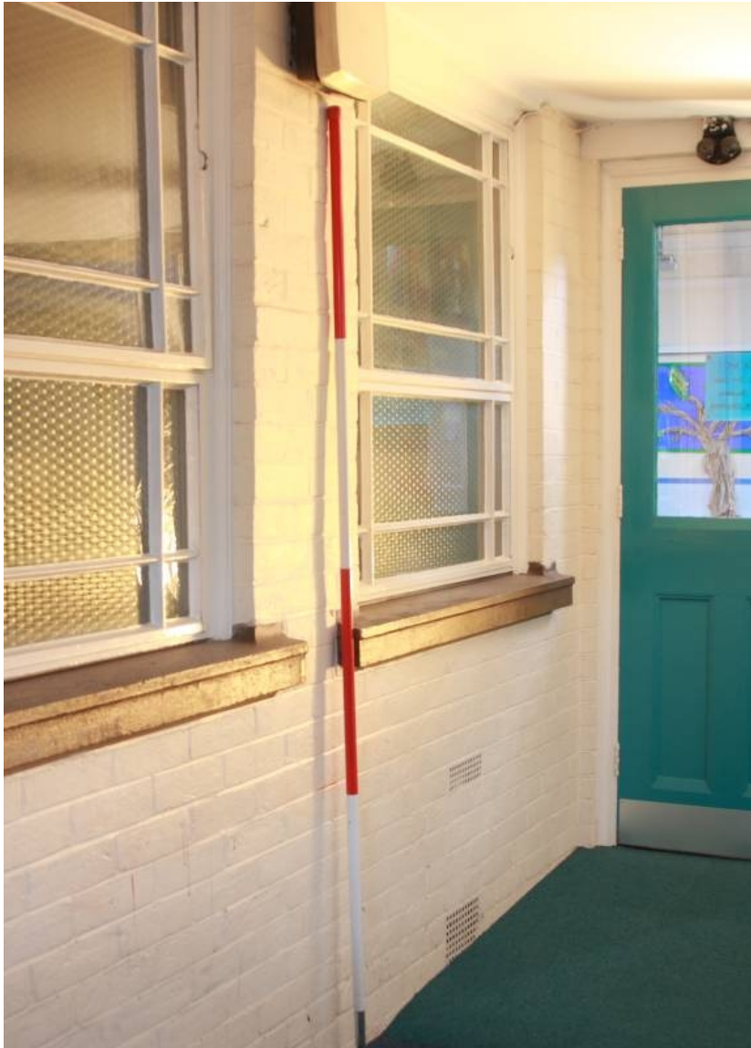
Plate 30. Original metal window, hall approach (scale 2m; from WSW)
