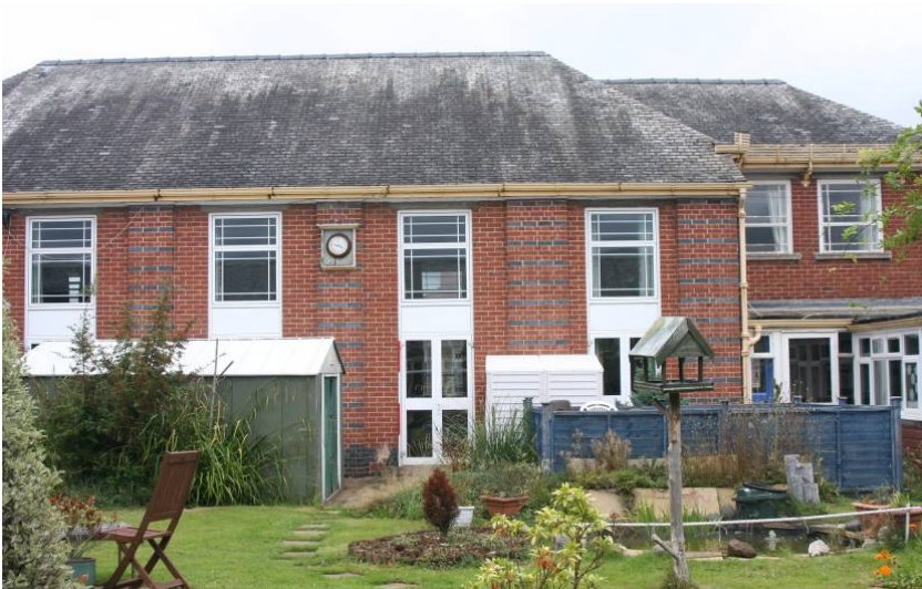
Plate 14. West courtyard interior, across 'cloister' garden (scale 2m; from E)
