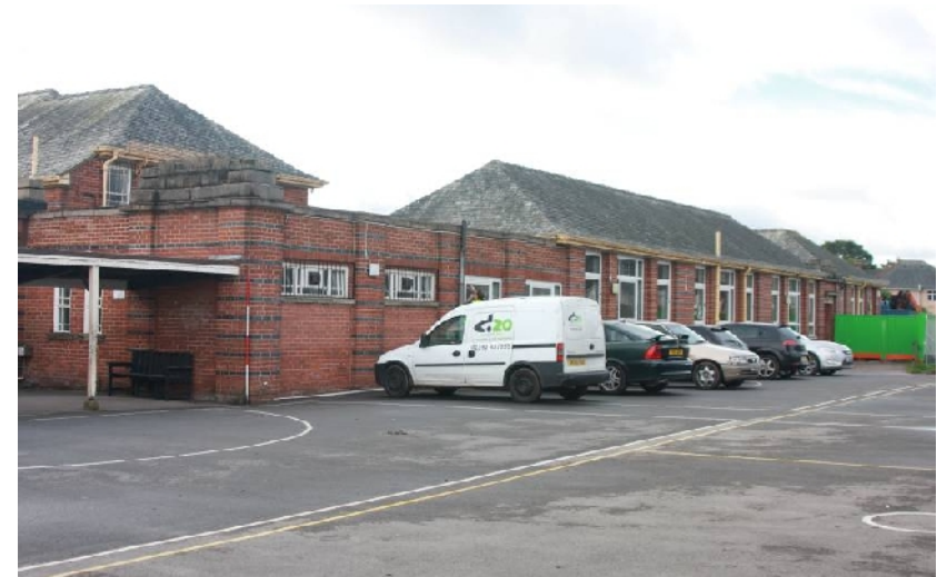
Plate 4. Main School, north west corner and west range exterior (scale 2m; from NNW)
