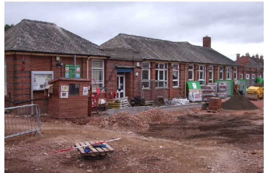
Plate 11. East range exterior (scale 2m; from SE)
