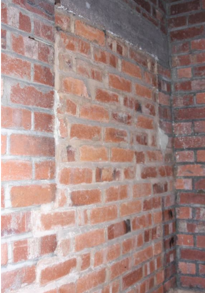
Plate 48. Detail of MOWP Hut (D) brickwork (from SE)
