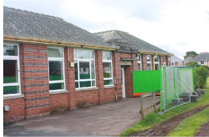
Plate 2. Overview of brickwork and western entrance, Scale 2m, Looking SE
