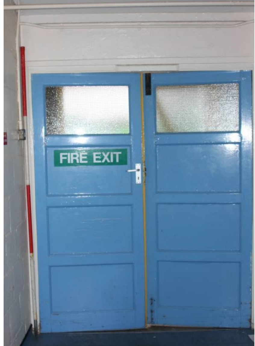
Plate 49. East exit from MOWP Hut (D) (scale 2m; from W)
