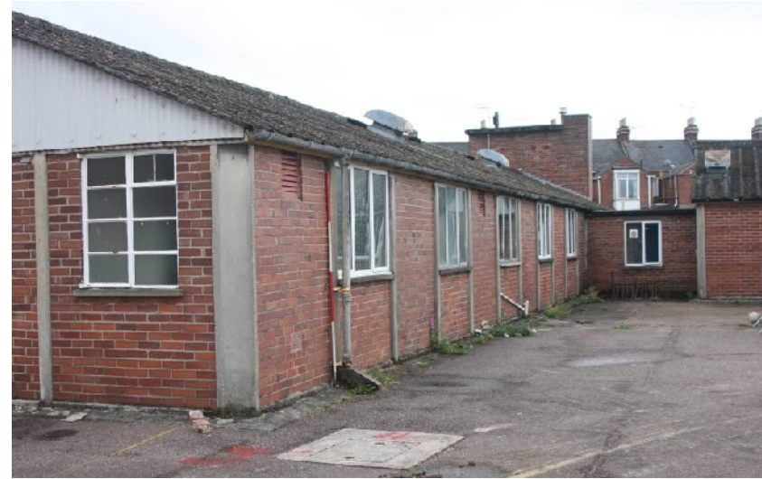
Plate 36. MOWP Hut (D), west exterior (scale 2m; from NNW)
