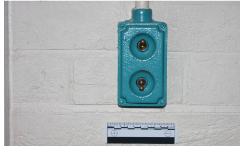
Plate 33. West corridor, light switch (scale 0.1m, from E)
