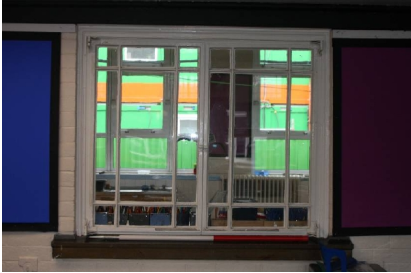
Plate 26. Original east range metal casement window (scale 1m; from W)
