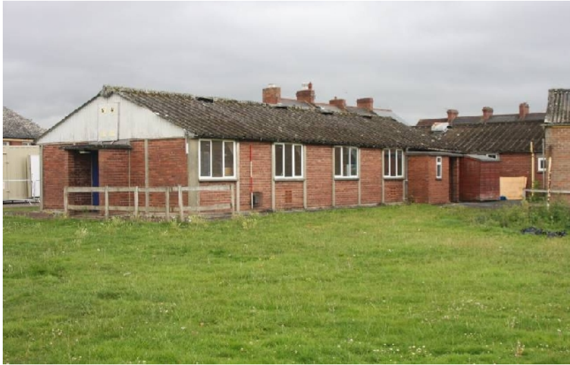
Plate 35. MOWP Hut (E) showing roof structure (scale 2m; from SW)
