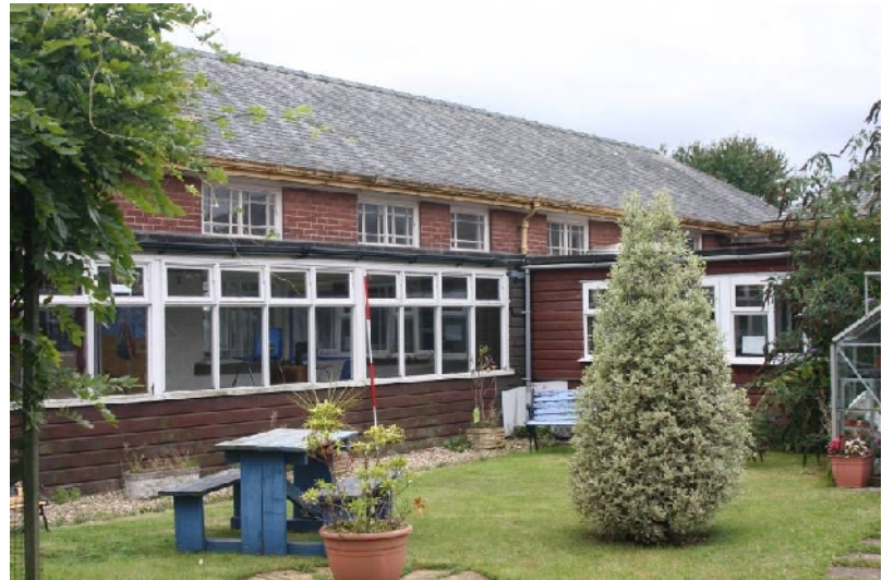
Plate 15. Junction of north and east ranges courtyard interior (scale 2m; from SW)
