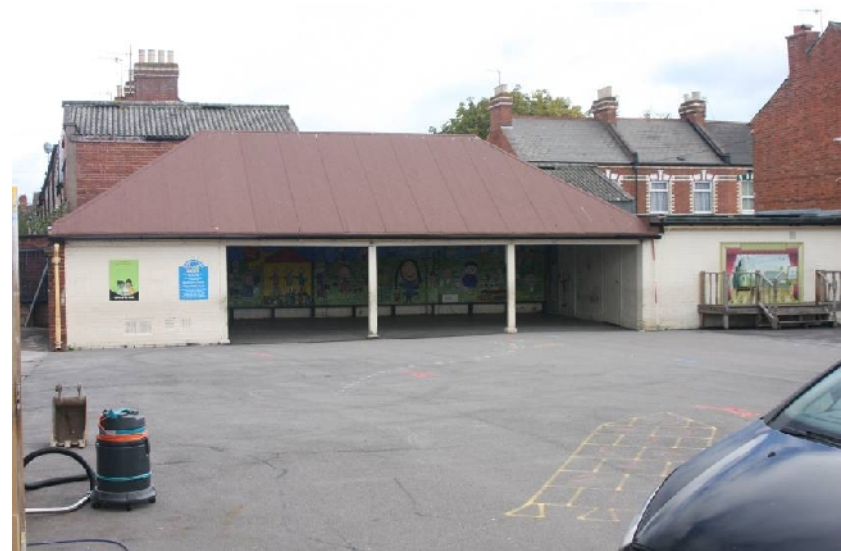
Plate 9. Covered play area (C) (scale 2m; from SSW)
