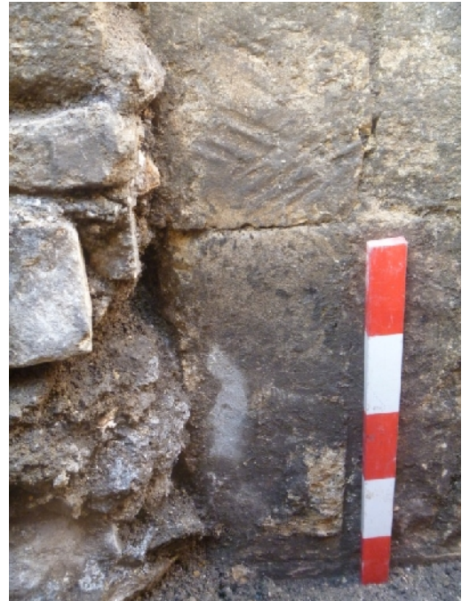
Plate 4. Close-up of diagonal tool marks on wall (106) (from E; 0.5m scale)
