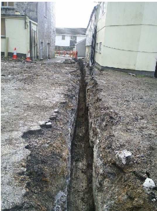
Plate 1. Service trench along NW side of Former Corn Mill (from NE)
