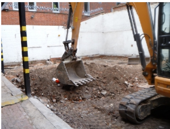
Plate 1. Demolition of outbuildings (from W)
