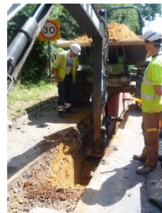
Plate 2. Open cut trenching along Bere Road (from N)
