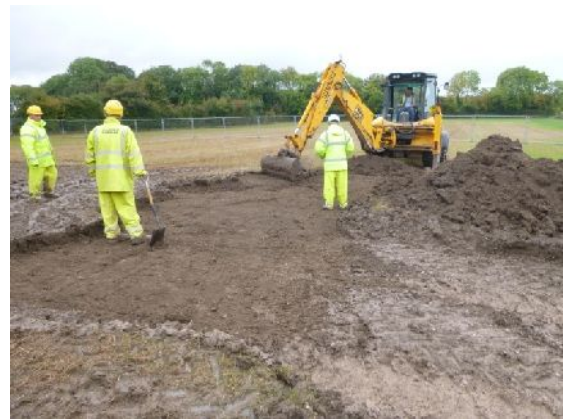
Plate 2. Compound strip (from E)
