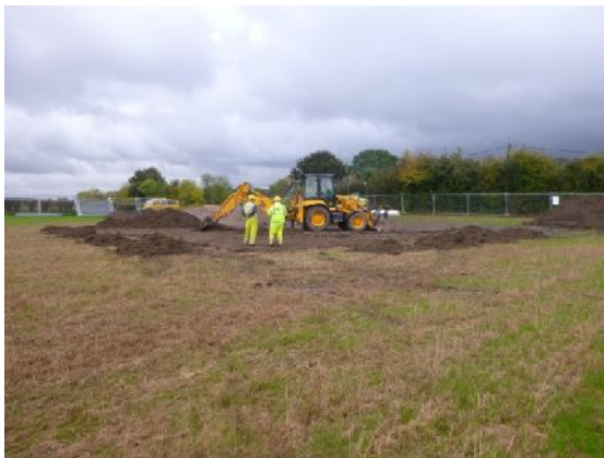
Plate 1. Compound strip (from W)
