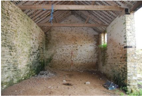
Plate 27. B5 interior west elevation (from E)
