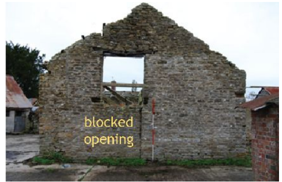
Plate 10. B2 exterior south elevation (from S)
