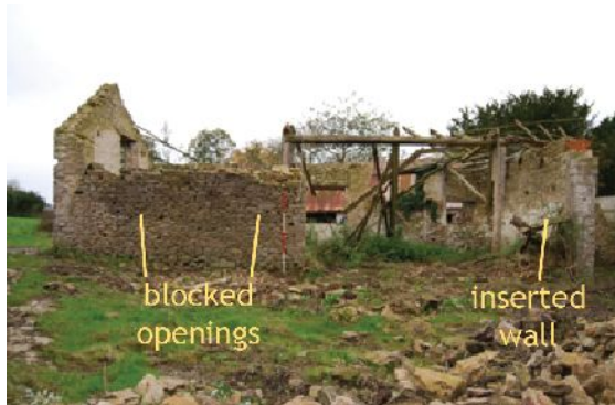
Plate 9. B2 exterior east elevation (from E)
