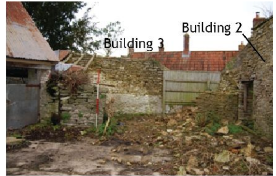
Plate 16. B3 exterior south elevation (from S)
