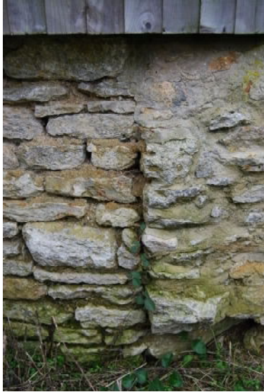
Plate 7. B1 interior north elevation showing junction in masonry (from S)
