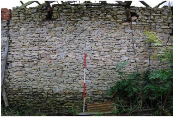
Plate 13. B2 north elevation forming interior south elevation of B1 (from N)
