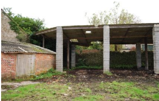
Plate 33. B7 exterior east elevation, south end (from NNW)
