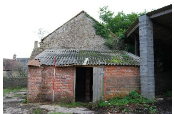
Plate 32. B6 exterior west elevation (from W)
