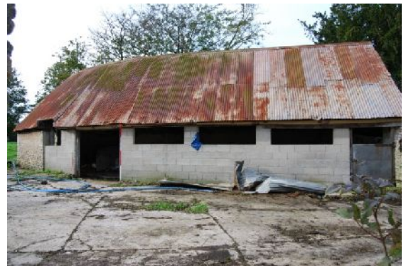
Plate 20. B4 exterior east elevation (from E)
