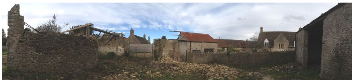
Plate 37. Panorama of eastern farmyard: from left - B2, B1, converted part of B1, listed barn, Court Farm House and B5
