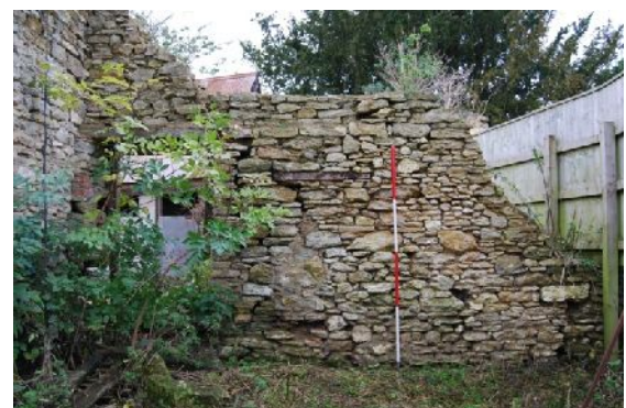
Plate 6. B1 interior west elevation (from E)
