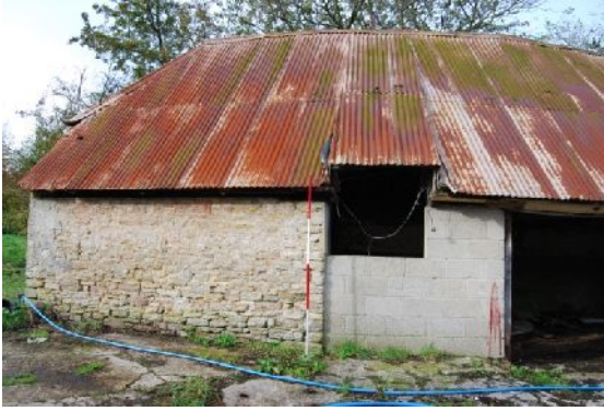
Plate 21. B4 exterior east elevation, south end (from SE)
