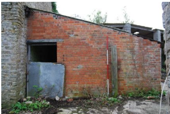
Plate 31. B6 exterior north elevation (from E)
