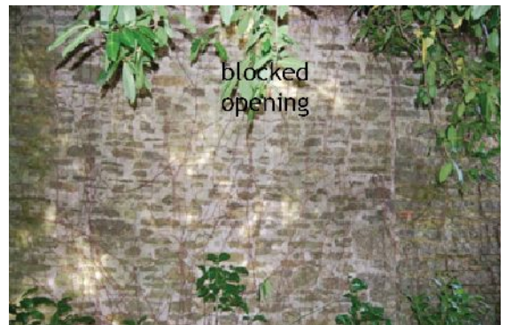
Plate 30. B5 exterior south elevation, blocked doorway (from S)
