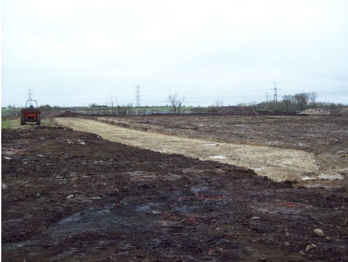
Plate 1. Phase 1 - road strip
