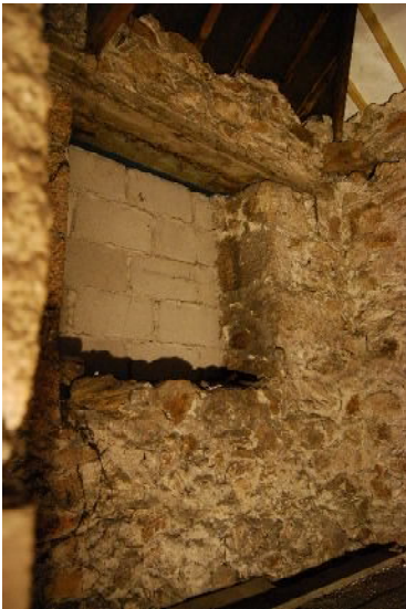
Blocked window in first floor of building I (from SW)
