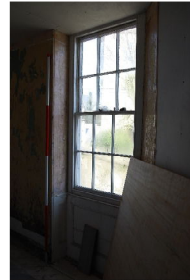
Exemplar window in first floor bedroom of building F with wooden surround (from SW; 2m scale)
