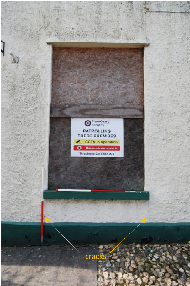
Plate 6. Window re-modelled from former doorway at S end of east flank (from E; 2m scale)
