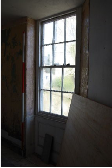
Plate 10. Exemplar 1 st floor window in building F (from SW; 2m scale)
