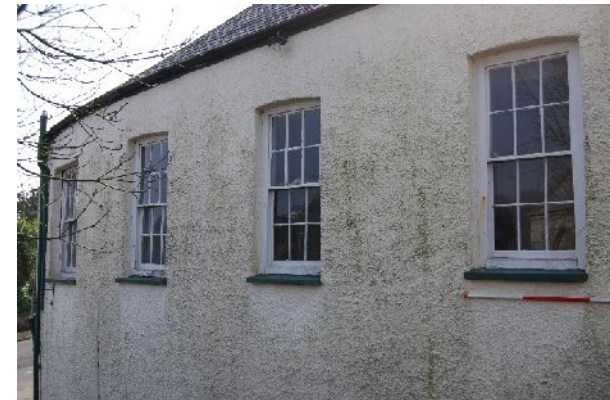
Building F (from NW; 1m scale)
