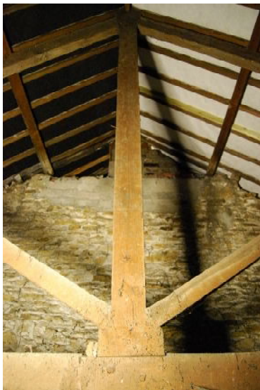
Roof at southern end of building A (from N)
