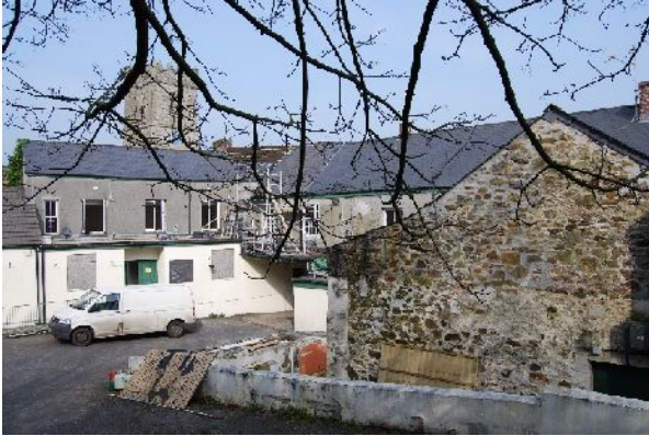
West side of complex following removal of modern extension (from SW)
