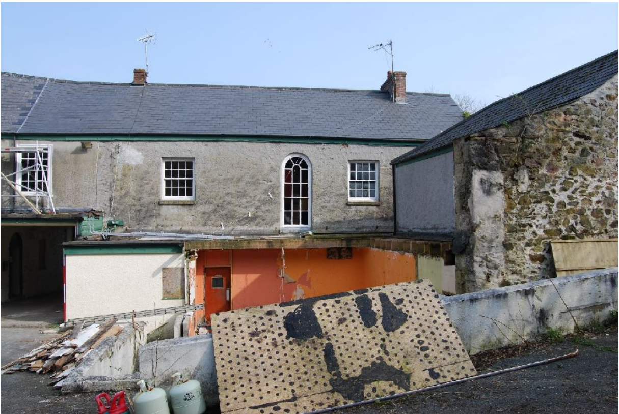
Plate 11. West elevation of building A (from W; 2m scale)
