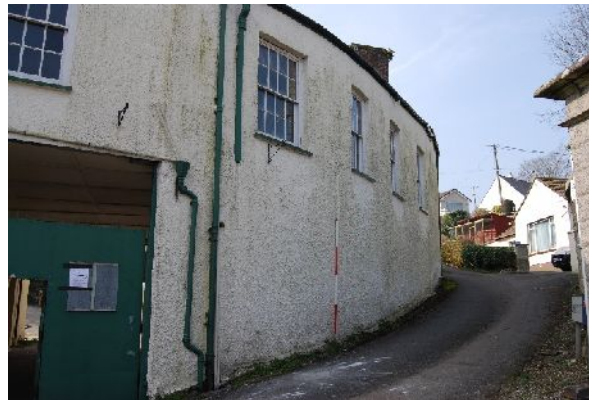
Coaching entrance E & building F (from E; 2m scale)
