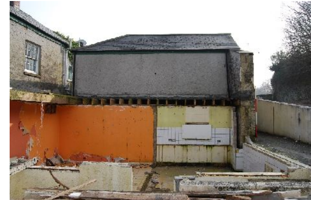
Building I following removal of modern extension (from N; 2m scale)
