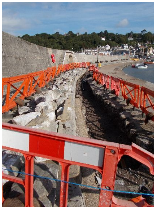
Plate 2. Duct trench in Area 4 (from SSW)
