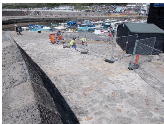
Plate 31. Repairs adjacent to aquarium (from SW)
