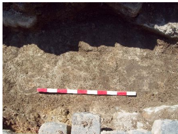
Plate 25. Earlier surface of large Lias blocks in duct trench, from 26.50m northwards (from E; 1m scale)
