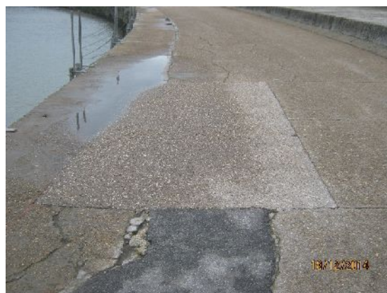
Plate 10. Concrete repair in Area 2 (from the NNW; photo by David Wilson)
