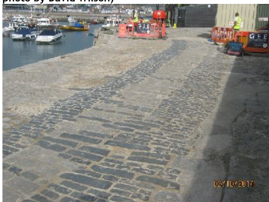
Plate 11. Repointing of Areas 8 & 9 (from the SW; photo by David Wilson)
