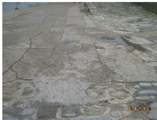
Plate 6. Duct trench concrete reinstatement (from the N; photo by David Wilson)
