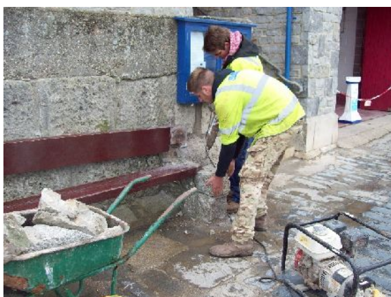
Plate 30. Removal of benches south of RNLI shop (from SE)
