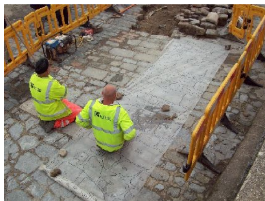
Plate 4. Removal of cobbles to tracing on side of trench (from N)
