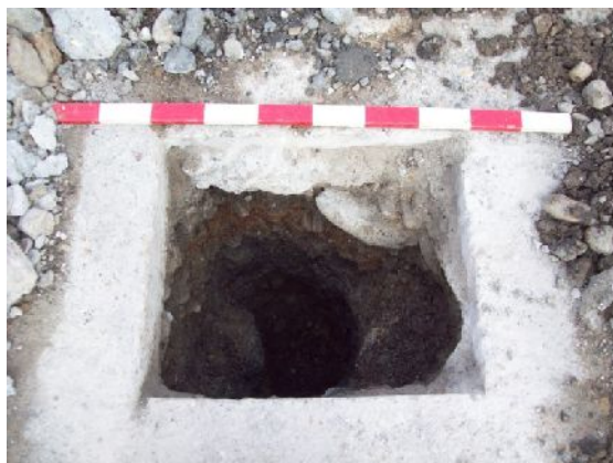
Plate 14. Trial Hole 1 excavated (1m scale)
