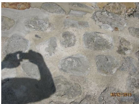
Plate 32. Re-pointing in NHL5 in Area 10 (photo from David Wilson)
