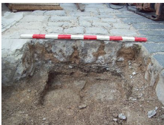
Plate 26. Profile of earlier surface of Lias blocks below present cobbled surface, N end of duct trench (from E; 1m scale)
