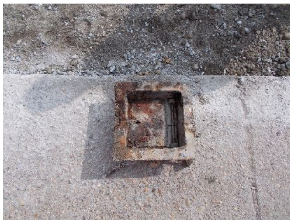
Plate 29. Cast iron surround recovered from make-up in Area 2 (1m scale)
