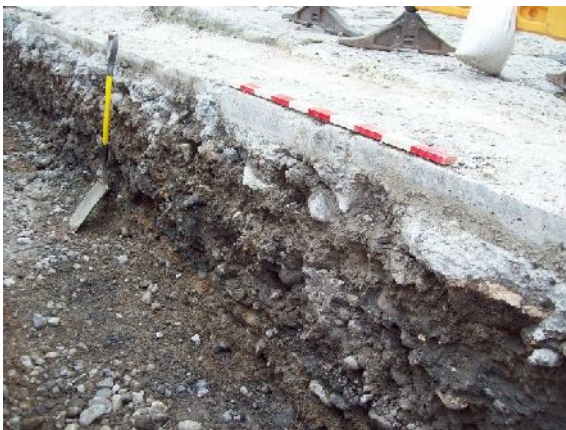
Plate 22. Southern end of duct trench (from SW; 1m scale)
