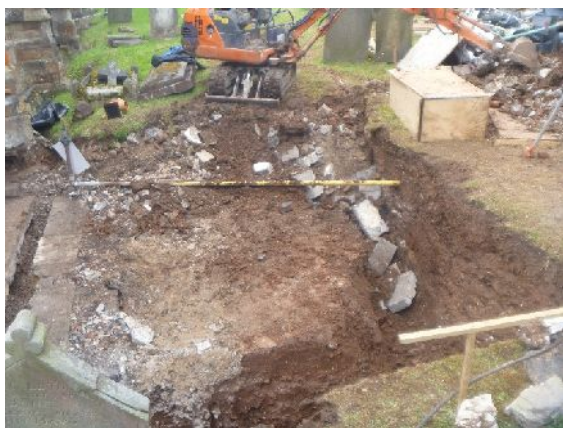
Plate 1. Footing trenches during excavation (from NE)
