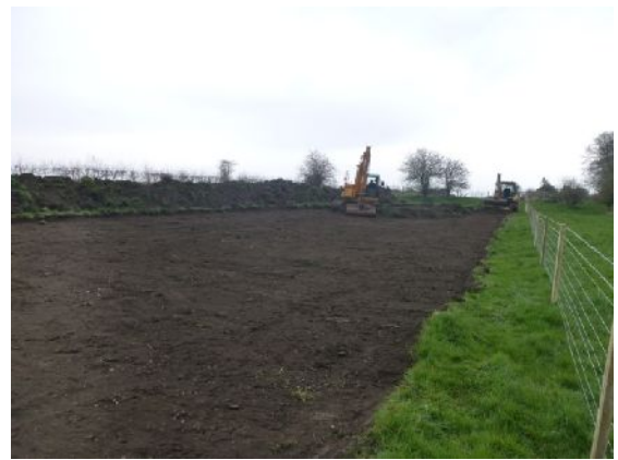
Plate 2. View along easement (from W)
