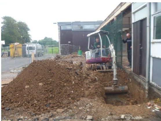
Plate 1. General shot showing excavation of Tr1 (from N)
