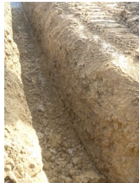
Plate 4. Profile 3 and sewer trench (from NW; no scale)
