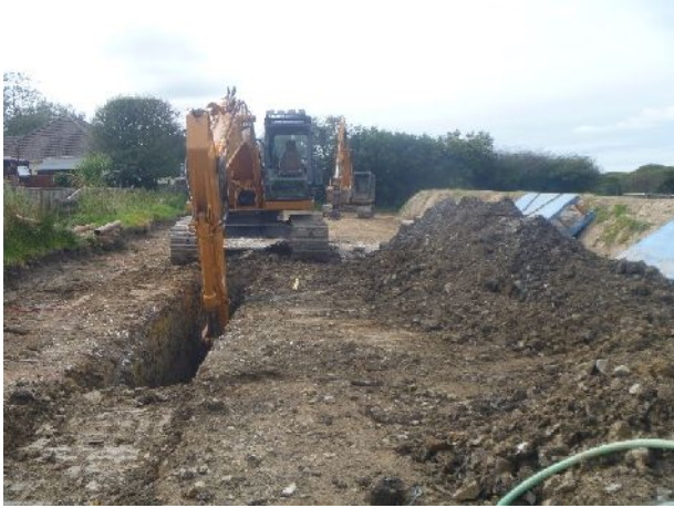
Plate 1. Stripping and excavation along pipeline route (from NW)
