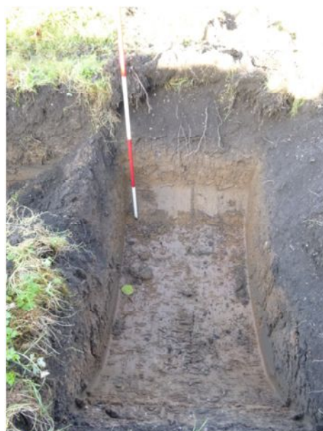
Plate 4. Trench 3, Sondage at east end for builders reference showing depth of geology (from W; 2m scale)
