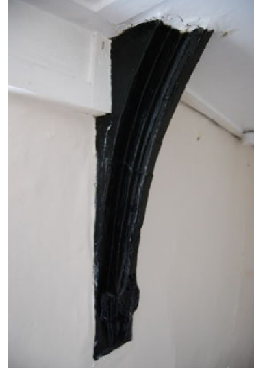
Plate 14. Cruck blade in first-floor room (from WSW)
