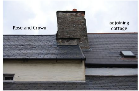
Plate 8. Chimney at SE end of Rose & Crown, showing slate drip course & original roof level (from SW)
