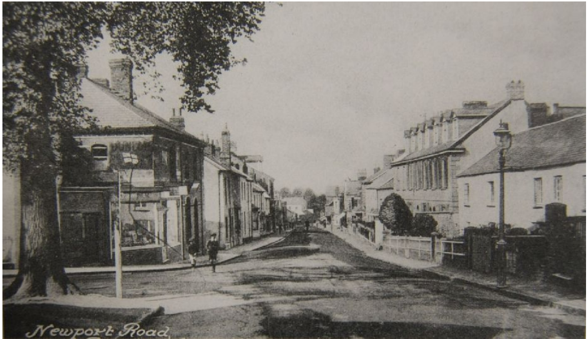
Plate 4. Junction outside Rose & Crown showing hollow tree on left and 17 th century cottages on right, c. 1911 (Stone 2002)
