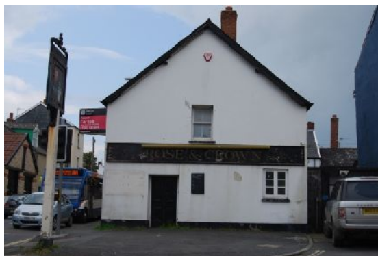
Plate 5. North-west elevation overlooking South Street (from NW)
