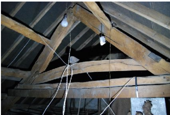
Plate 11. Roof showing jointed cruck truss towards E end (from WNW)
