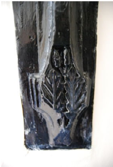
Plate 15. Carved foliage on cruck blade in first-floor room (from SSW)
