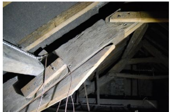
Plate 12. Joint of central cruck truss (from E)
