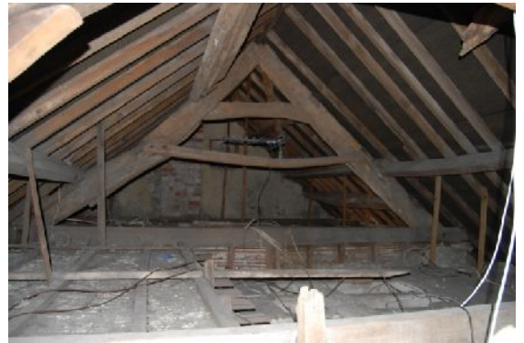
Plate 10. Roof showing jointed cruck truss towards W end (from SE)
