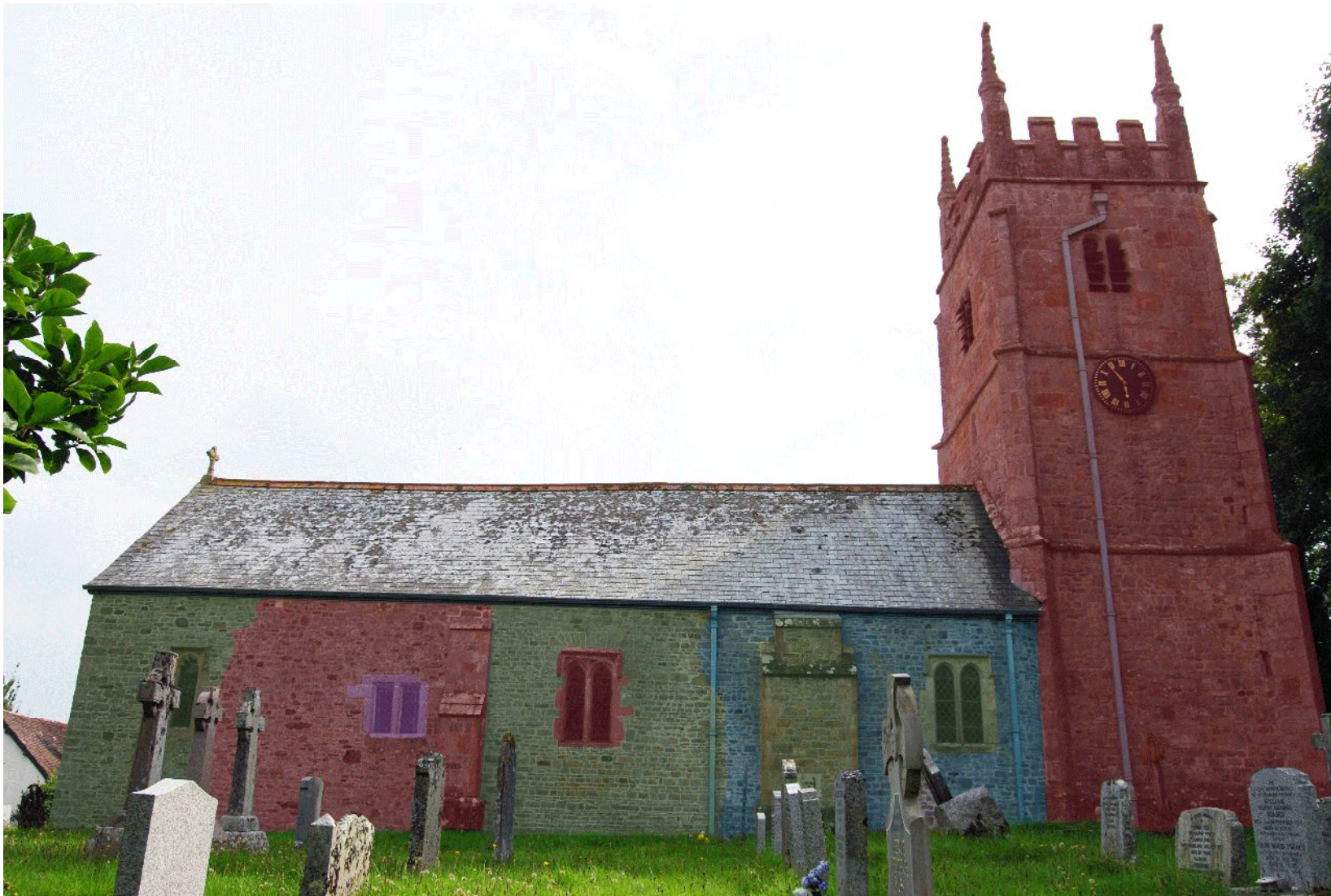
Plate 44. North elevation with approximate phasing, exterior (from N)
