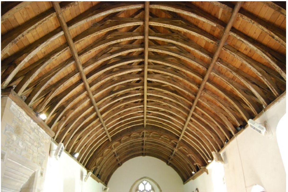
Plate 39. Wooden wagon roof with decoratively carved chancel arch (from W)
