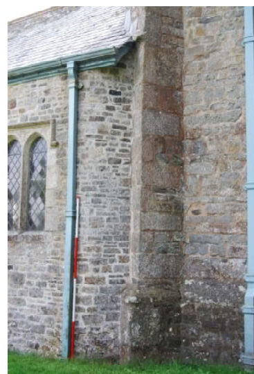
Plate 22. North-east corner of nave showing curved nave walling adjacent to scales abutted by tower to right (from NW; 1 x 2m scales)
