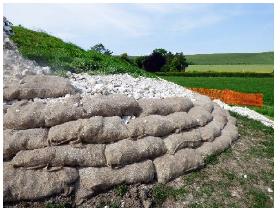
Plate 15. Bunding of Dairy Farm barrow and chalk in-filling complete
