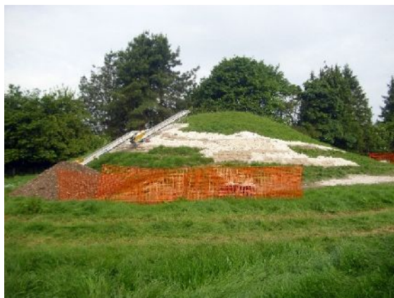
Plate 20. Dairy Farm barrow erosion scar repair work in progress from E
