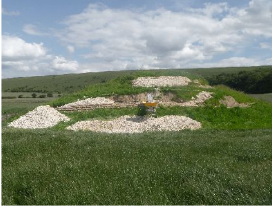
Plate 25. Truncombe Wood barrow erosion scar repair work in progress from NW
