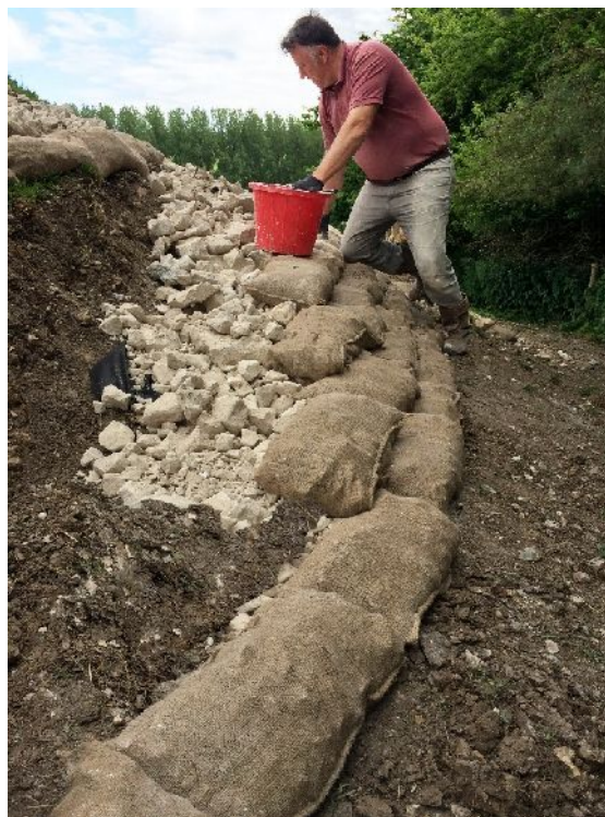
Plate 14. Bunding the larger erosion scars in progress
