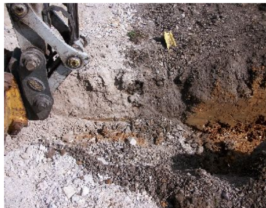
Plate 4. Chalk used in the demolished barn (from E)
