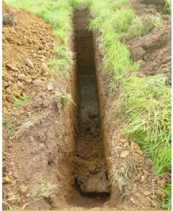
Plate 2. General inspection pit GI-01 (from NW)
