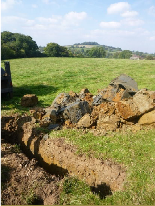
Plate 1. General view across GI-02 (from E)
