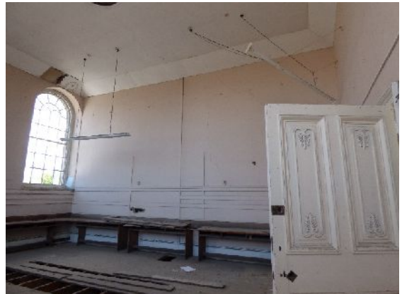
Plate 18. Desks in south side of first floor Lecture Room (from SE)
