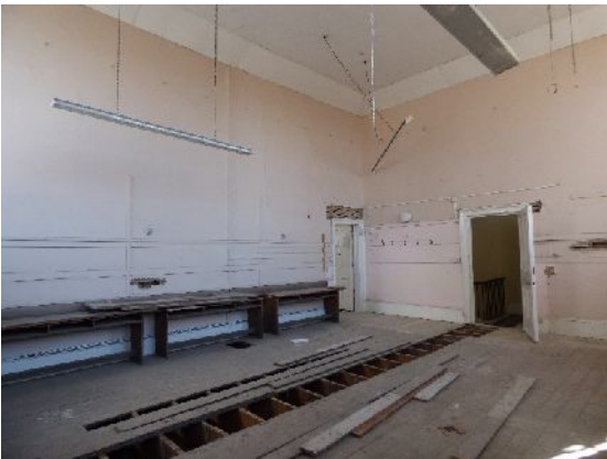
Plate 19. Desks in south side of first floor Lecture Room (from SW)
