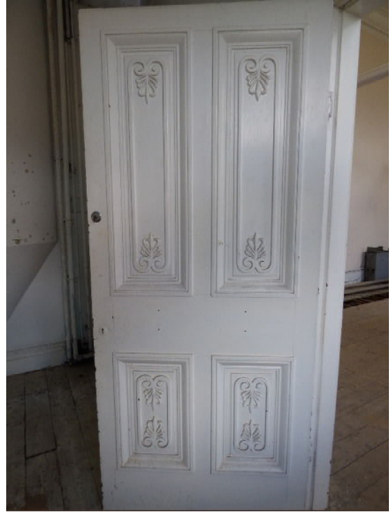
Plate 22. Panelled door between Lecture Room & adjacent office (from NNE)
