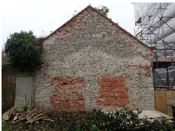
Plate 34. External west elevation of North Building (from W; 2m scale)
