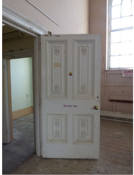
Plate 16. Panelled door between first floor landing & Lecture Room (from N)
