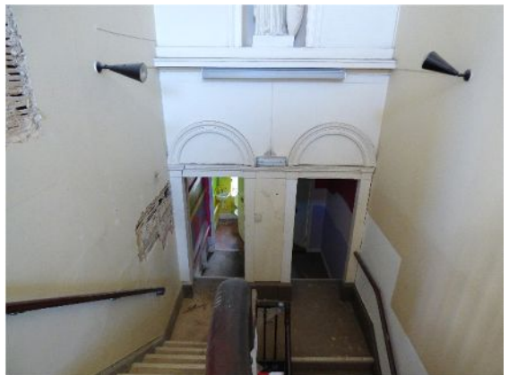
Plate 10. Half-landing from first floor landing (from S)
