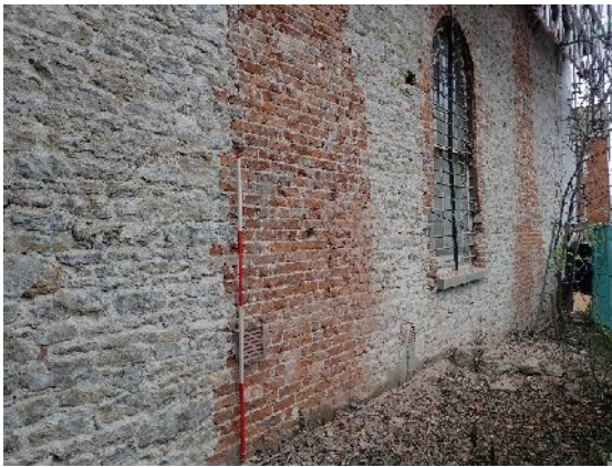
Plate 7. External west elevation showing brick chimney flues (from NW; 2m scale)
