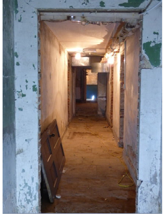
Plate 26. Basement hallway (from S)
