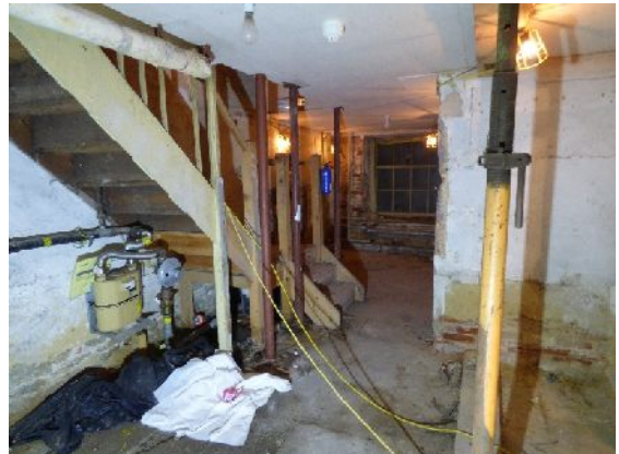
Plate 24. West side of basement showing internal stairs (from N)
