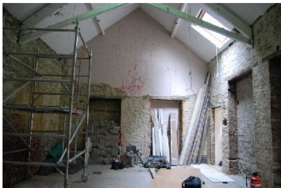
Plate 30. Ground floor of North Building showing brick arch above blocked door (from W; 1m scale)
