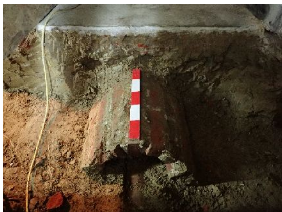
Plate 41. Modern brick culvert beneath basement hallway (from S; 1m scale)
