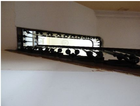
Plate 13. Staircase from ground floor with ceiling rose above
