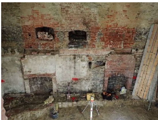
Plate 35. Internal north elevation of North Building showing fireplaces (from S)
