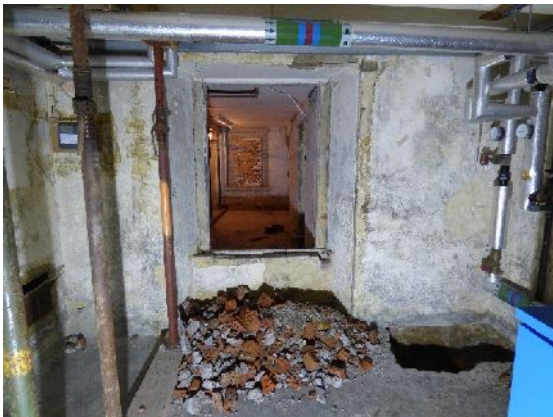
Plate 29. Window of north elevation from basement room (from S)
