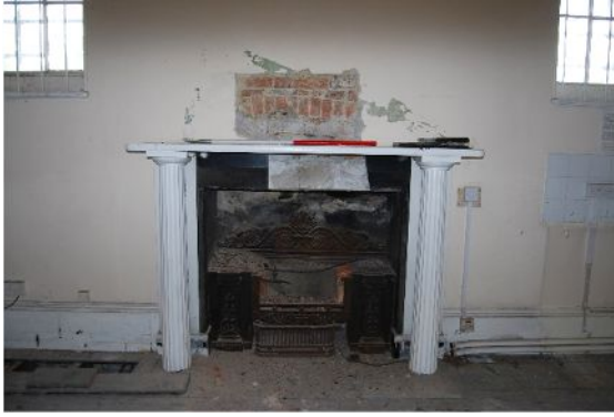
Plate 21. Later fireplace in first floor Lecture Room (from S)
