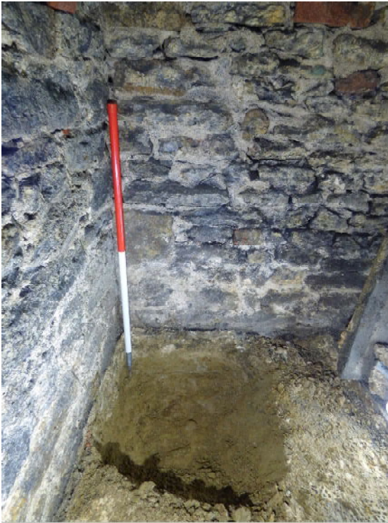
Plate 37. Test-pit in NE corner of North Building basement (from W; 1m scale)
