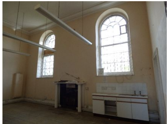
Plate 20. First floor Lecture Room, north side (from SE)
