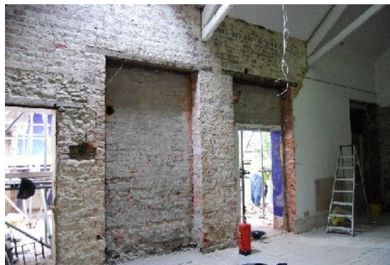
Plate 31. Ground floor of North Building (from NE)
