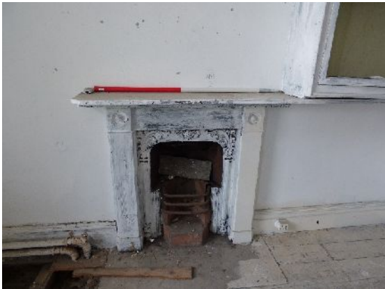
Plate 23. Fireplace in first floor office (from W)
