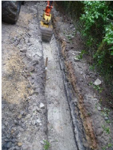
Plate 3. Working shot of pipe trench excavation (from N)
