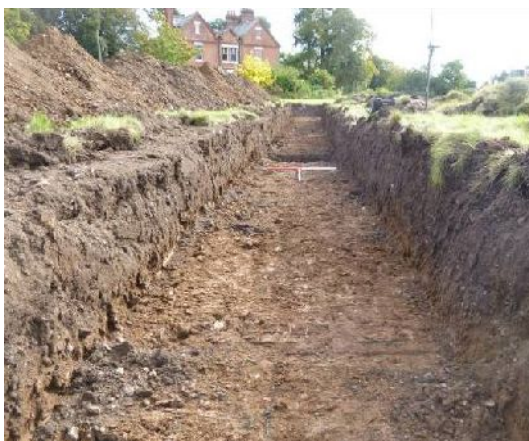
Plate 1. Trench 1 (from NW; 2 x 1m scales)
