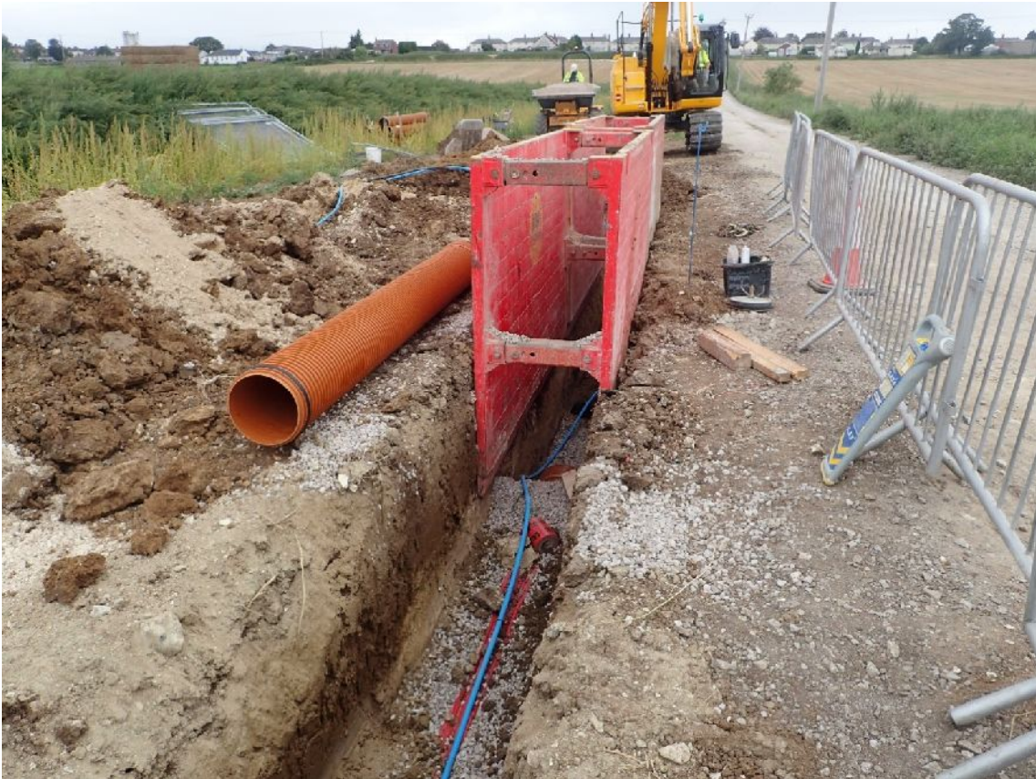
Plate 5. Pipe trench Profile 7 (facing N)
