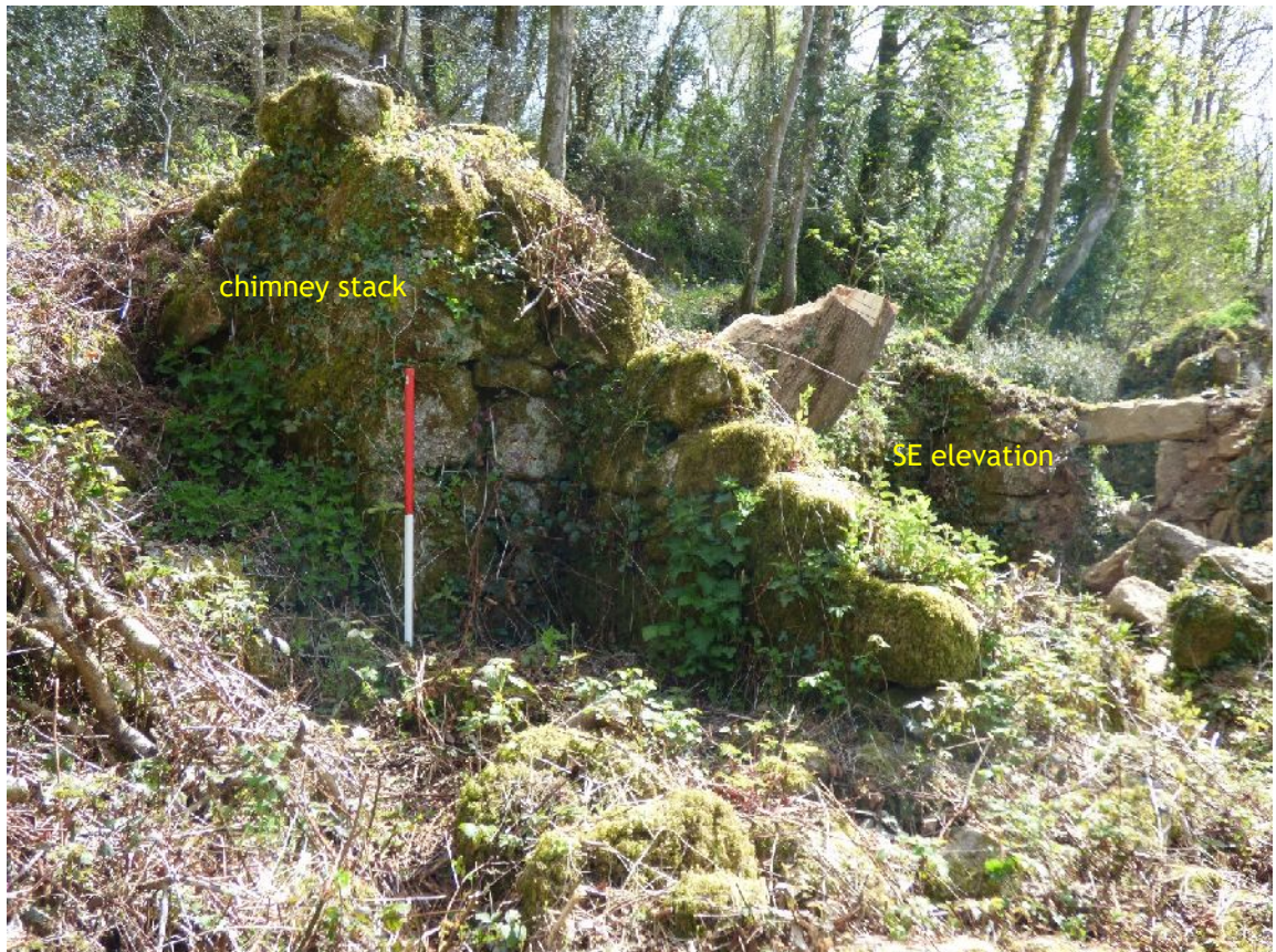
Plate 3. Building A - exterior NW elevation (from WNW; 1m scales)
