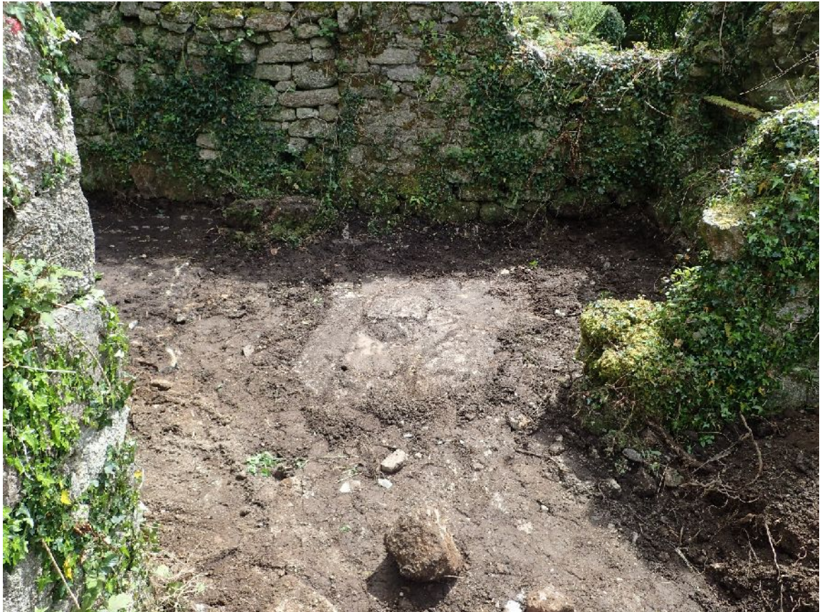
Plate 20. Building B - location of granite floor (7-200) & concrete slab (from NW)
