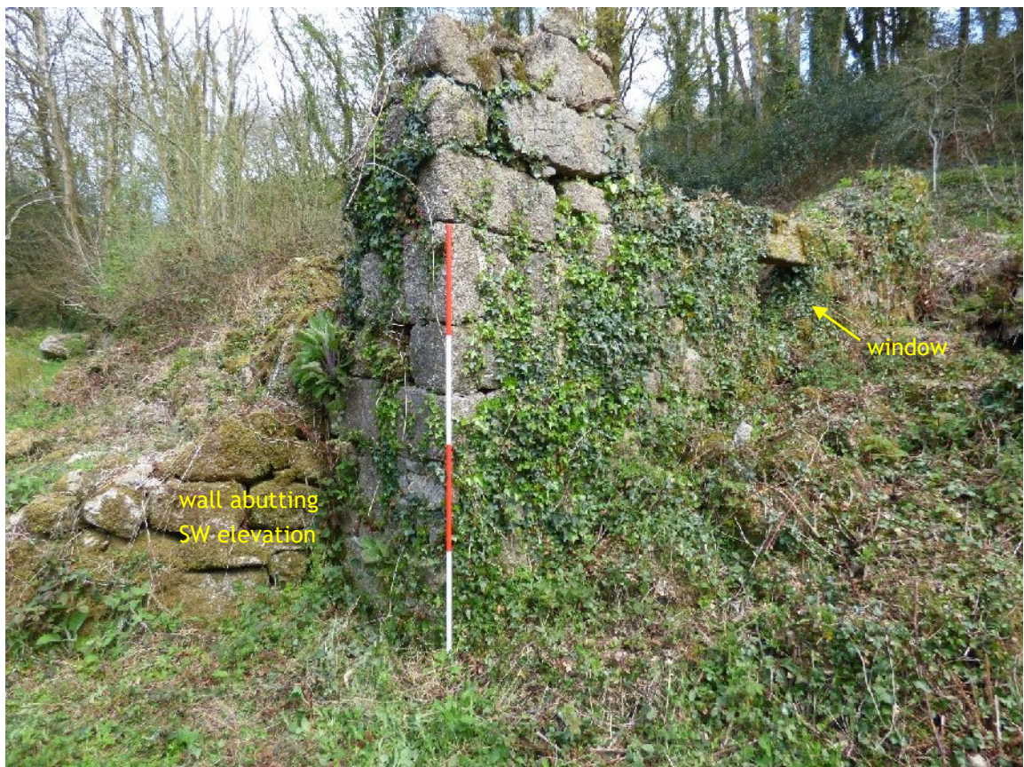
Plate 2. Building A - exterior SE elevation (from S; 2m scales)
