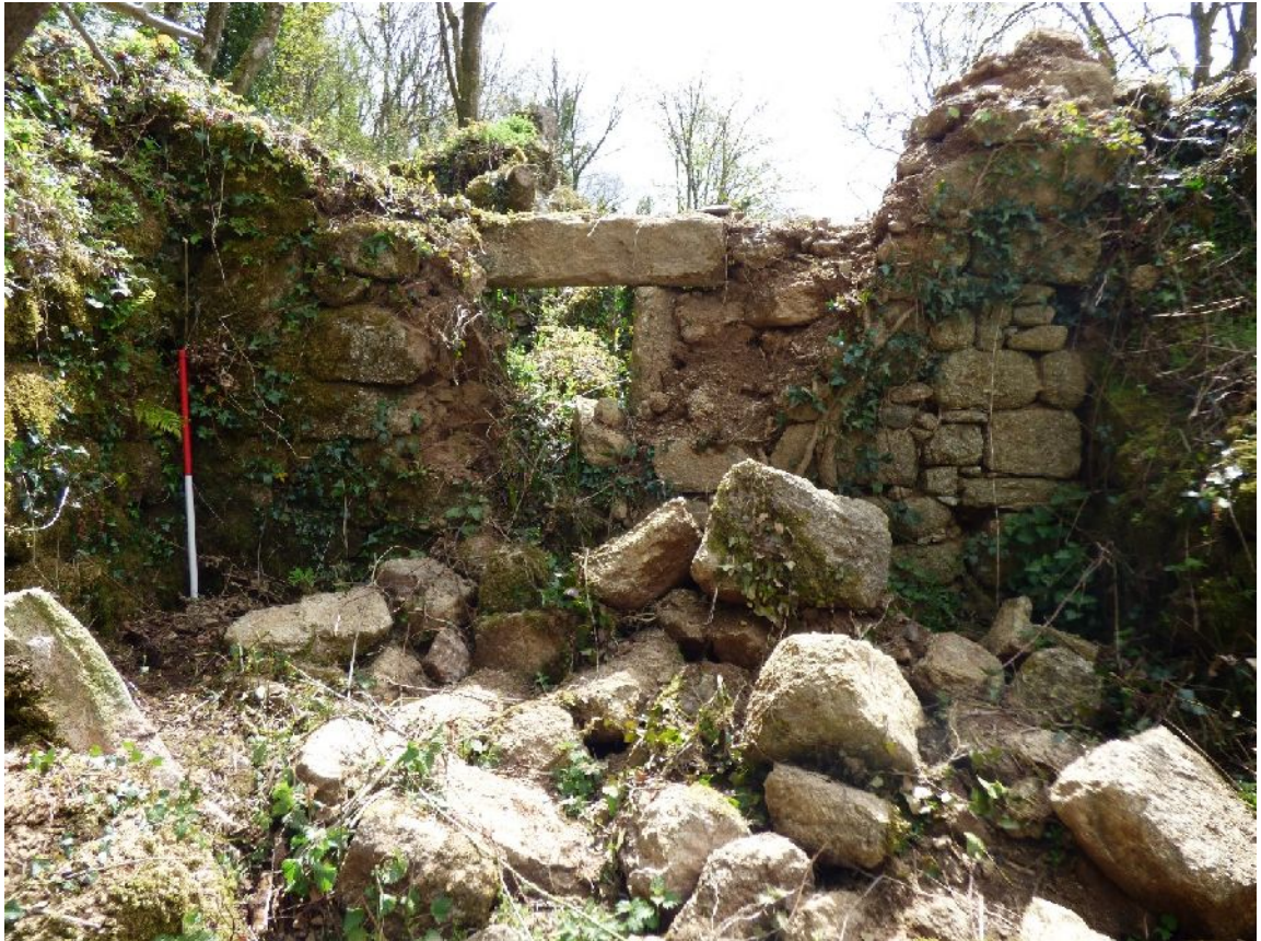
Plate 5. Building A - interior SE elevation with window (from NW; 1m scales)
