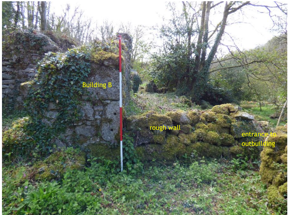
Plate 13. Building B - exterior NW quoin with two holes & outbuilding to SW (from NW; 2m scales)
