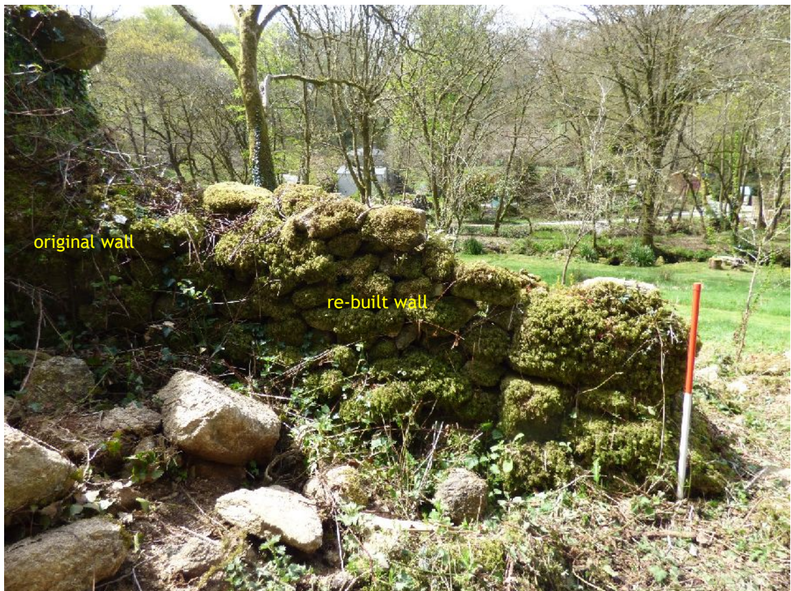
Plate 4. Building A - interior SW elevation (from NE; 1m scales)
