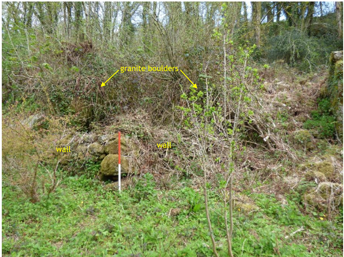
Plate 7. Outbuilding to NW of Building A (from S; 1m scales)
