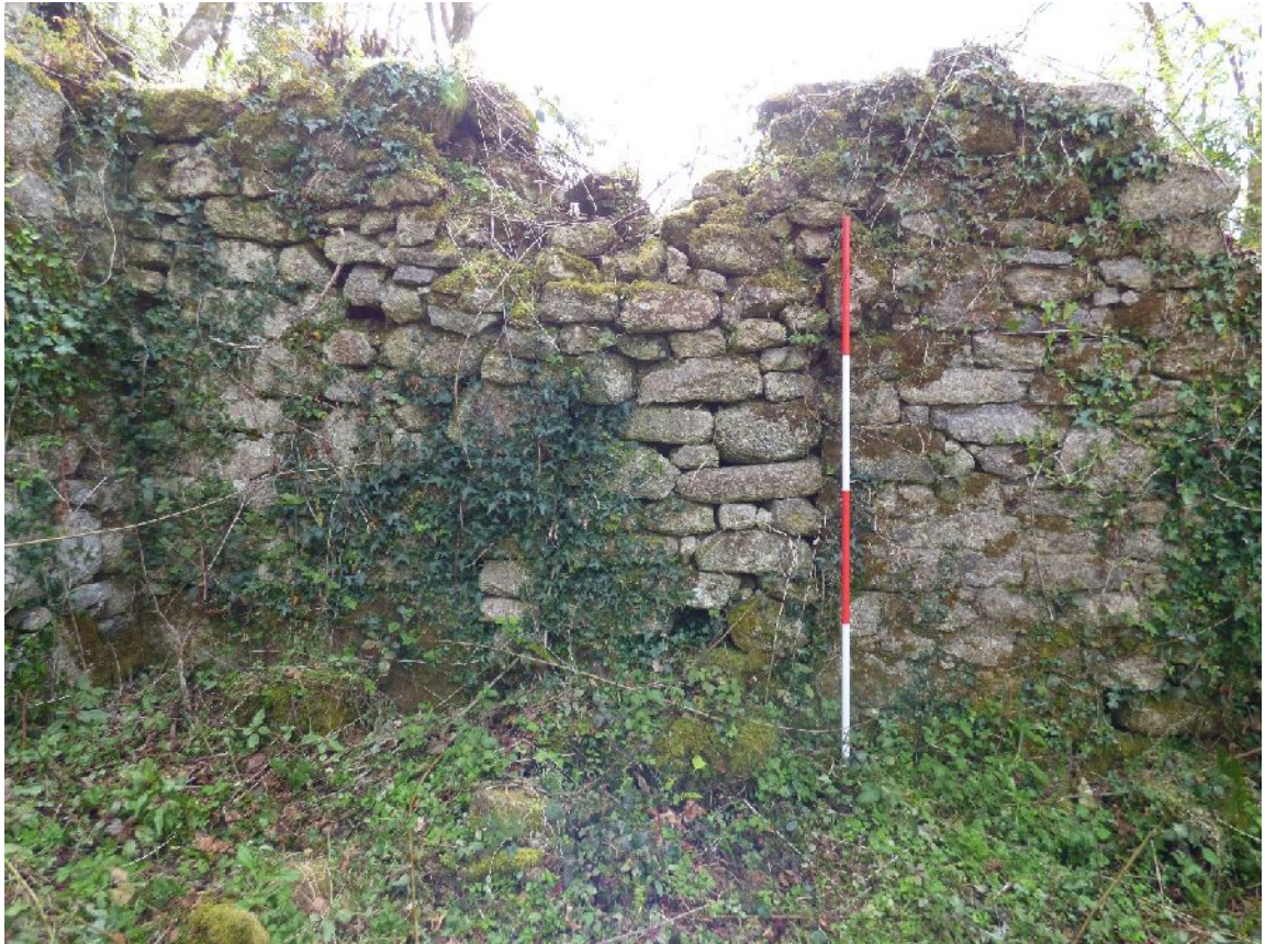
Plate 9. Building B - blocked doorway into southern cottage (from NW; 2m scales)
