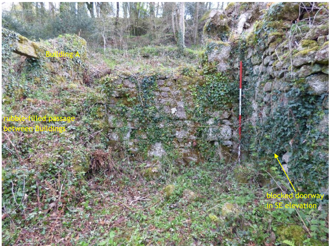
Plate 12. Building B - interior NE elevation (from SW; 2m scales)
