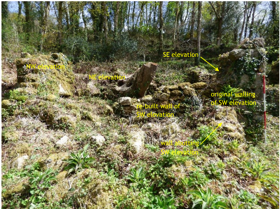
Plate 1. Building A (from SW; 2m scales)
