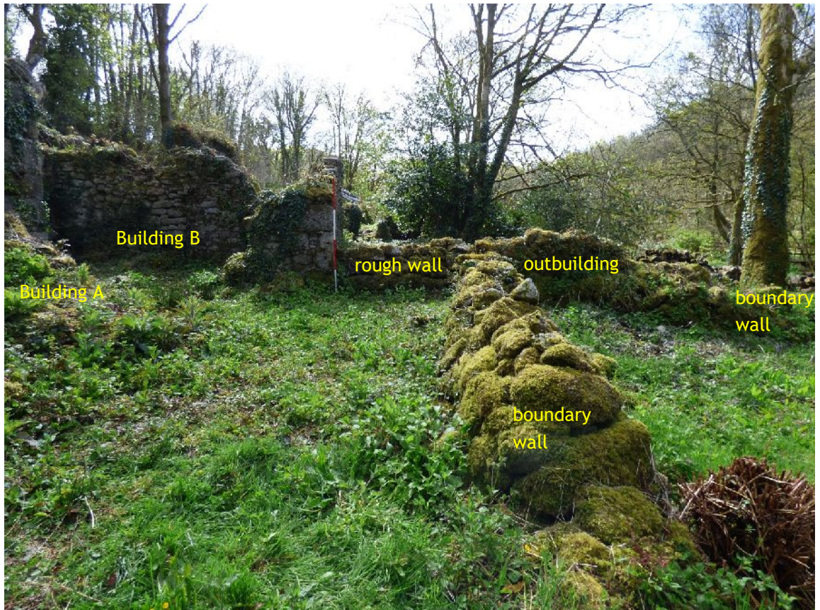
Plate 15. Boundary wall & outbuilding in front of cottages (from NW; 2m scales)
