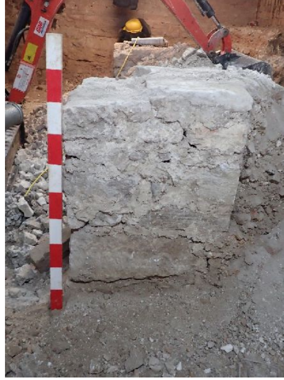
Plate 2. Foundation pier S2 (facing N; 1m scale)
