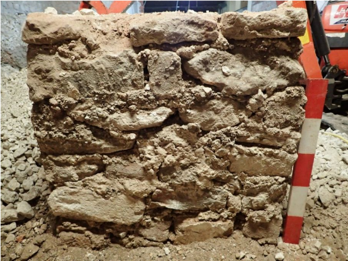
Plate 3. Foundation pier S3 (facing S; 1m scale)
