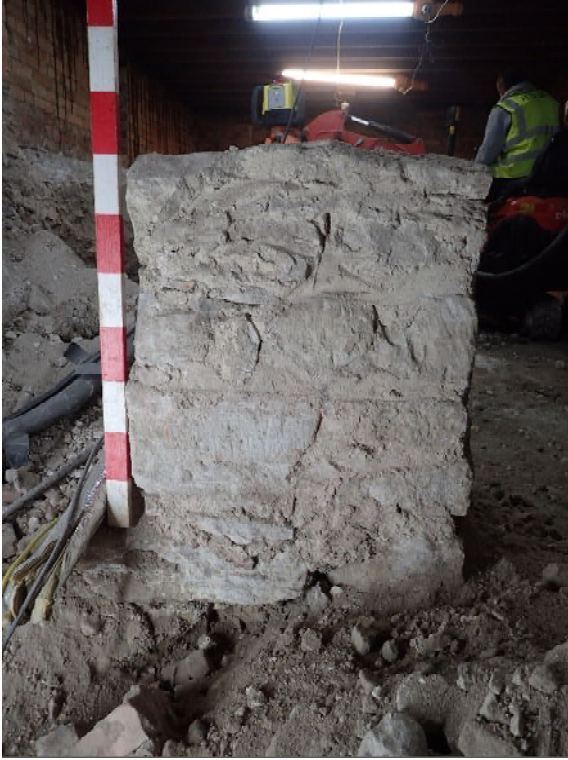
Plate 1. Foundation pier S1 (facing N; 1m scale)
