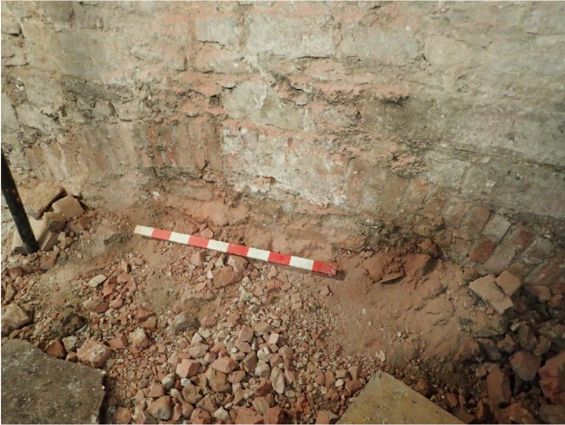
Plate 6. Foundation arch F7 (facing NW; 1m scale)
