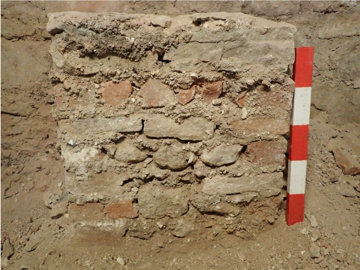
Plate 4. Foundation pier S4 (facing S; 1m scale)
