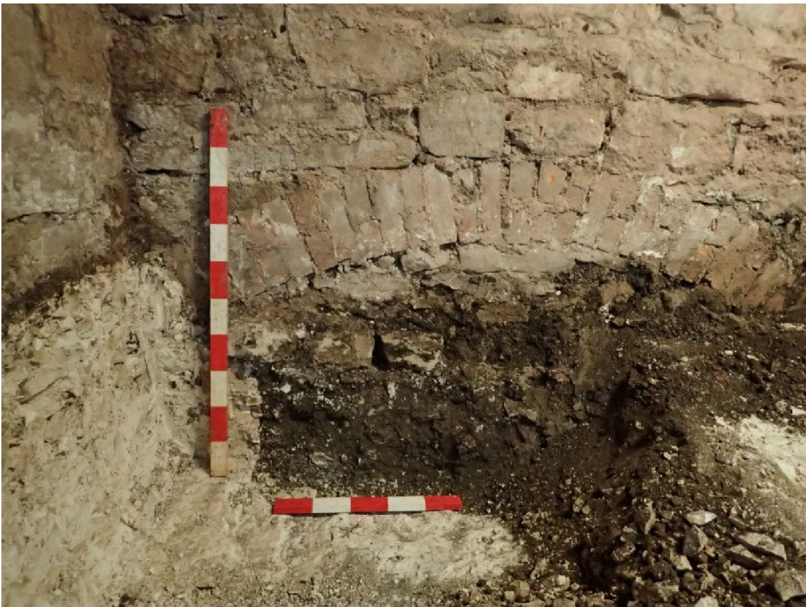
Plate 5. Foundation arch F5 (facing N; 1m and 0.50m scales)
