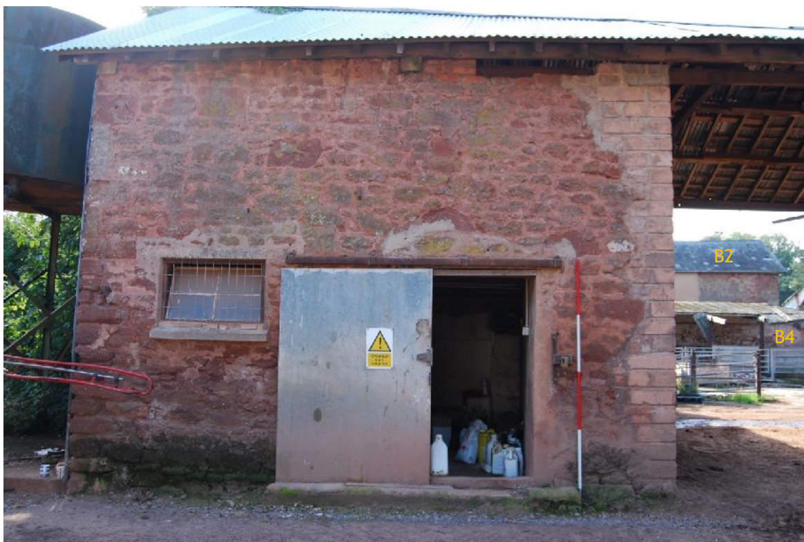
Plate 44. North-east exterior elevation of B6, S end (from NE; 2m scales)
