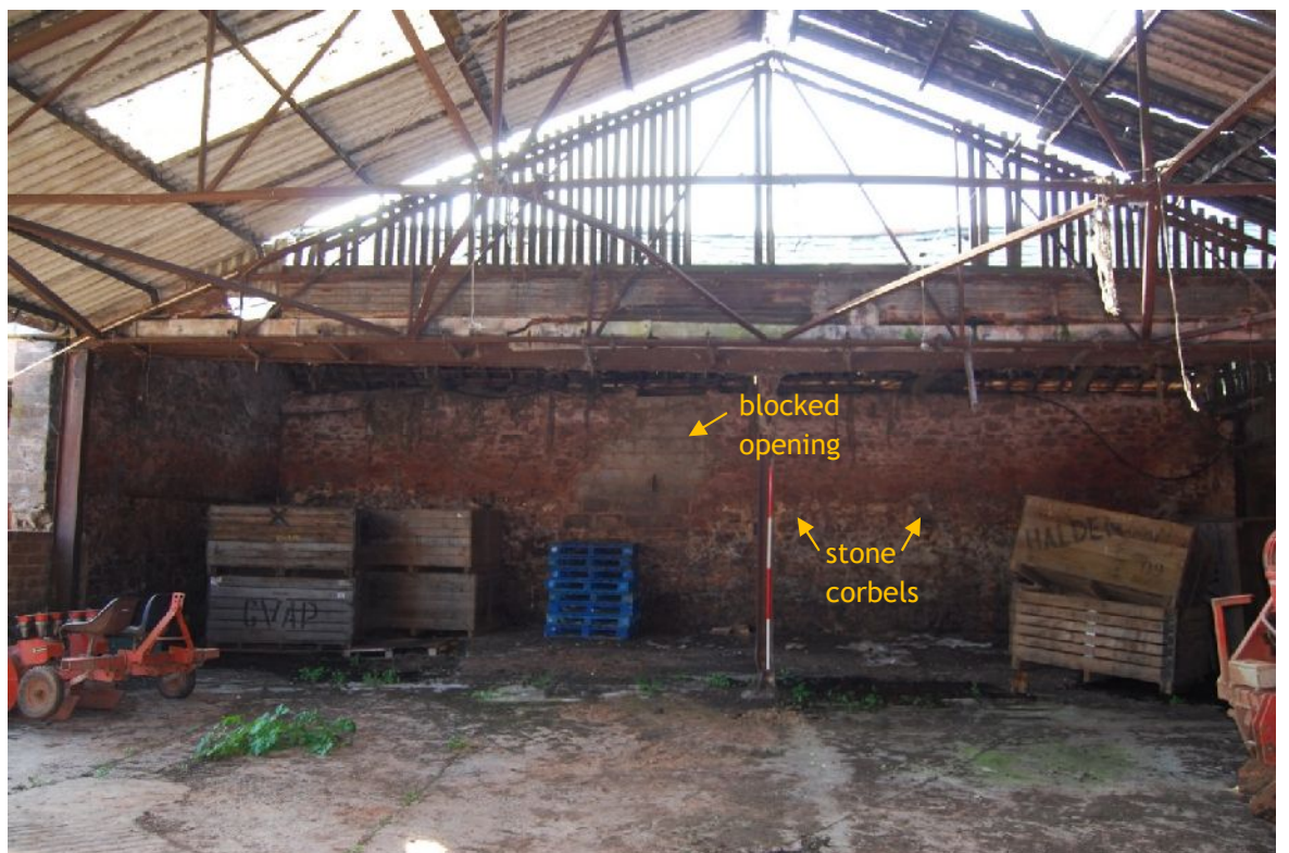
Plate 40. South-west interior elevation of B5 (from NE; 2m scales)
