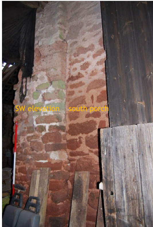
Plate 19. South-east side of south porch of B1, added to SW elevation (from WNW; 2m scales)
