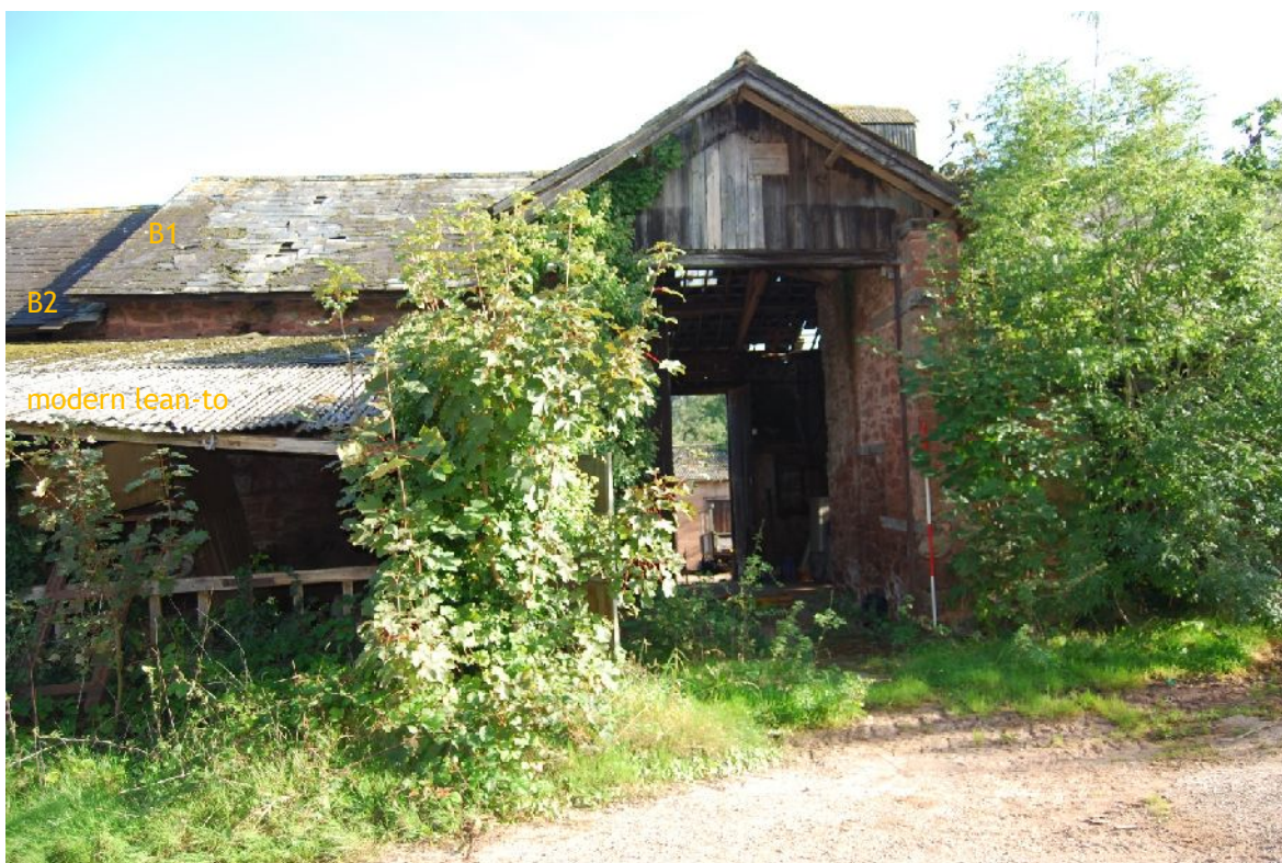
Plate 4. South-west elevation of B1 showing north porch (from WSW; 2m scales)
