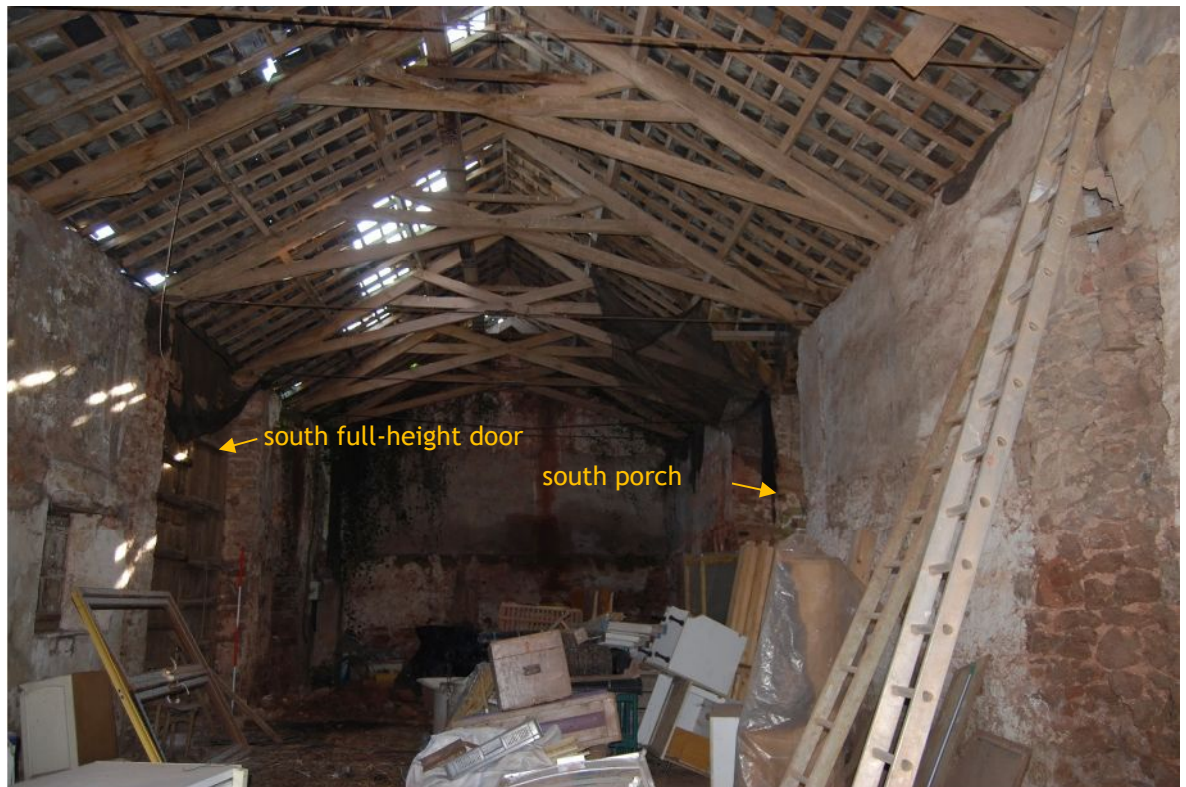
Plate 7. Interior of B1 showing scissor beam trusses (from NNW; 2m scales)
