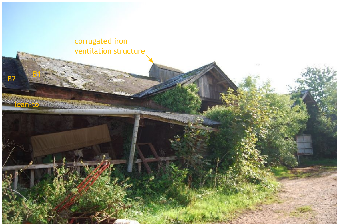
Plate 2. South-west elevation of B1 (from NW; 2m scales)
