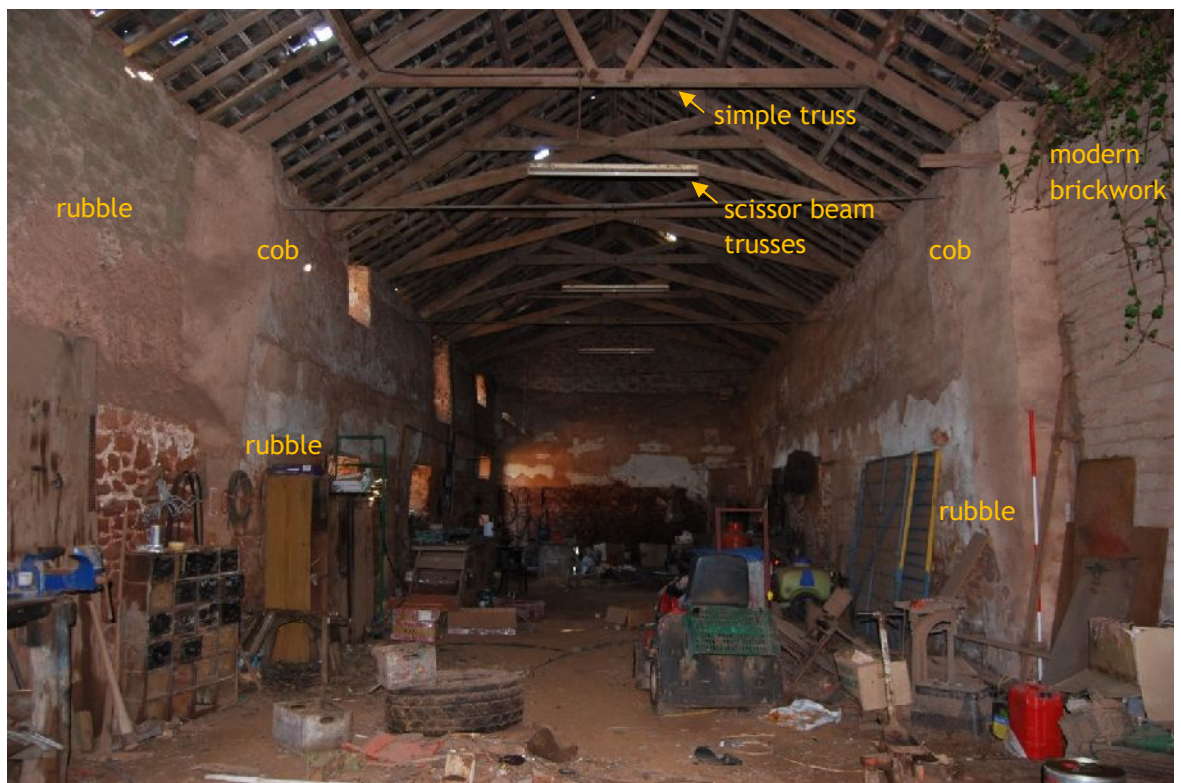
Plate 28. Interior of B2 showing change in build at N end (from NW; 2m scales)
