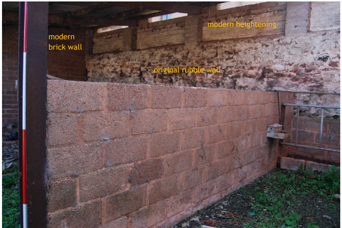
Plate 39. South-west interior elevation of B4 (from NNE; 2m scales)
