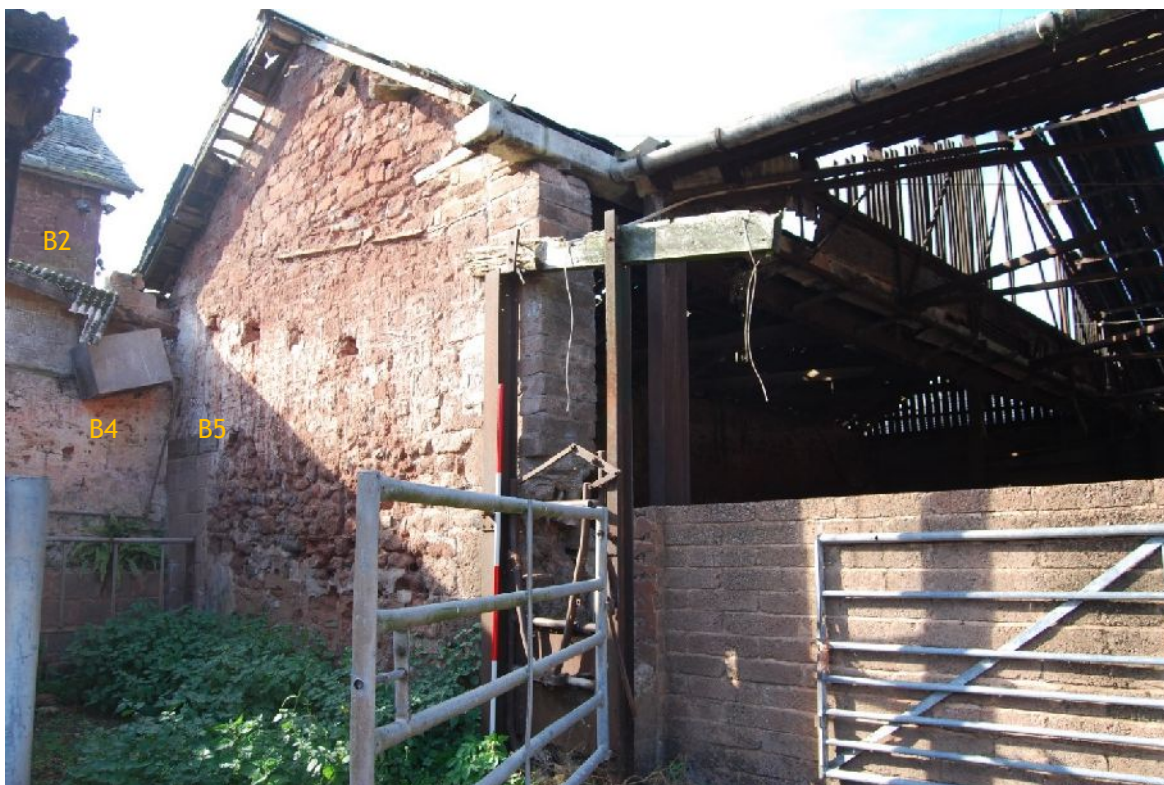
Plate 41. South-east gable of B5 (from ESE; 2m scales)
