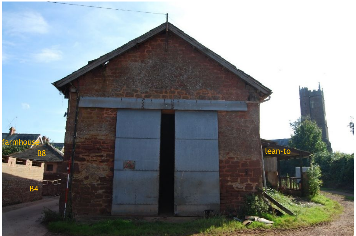
Plate 23. North-west gable of B2 (from NW; 2m scales)
