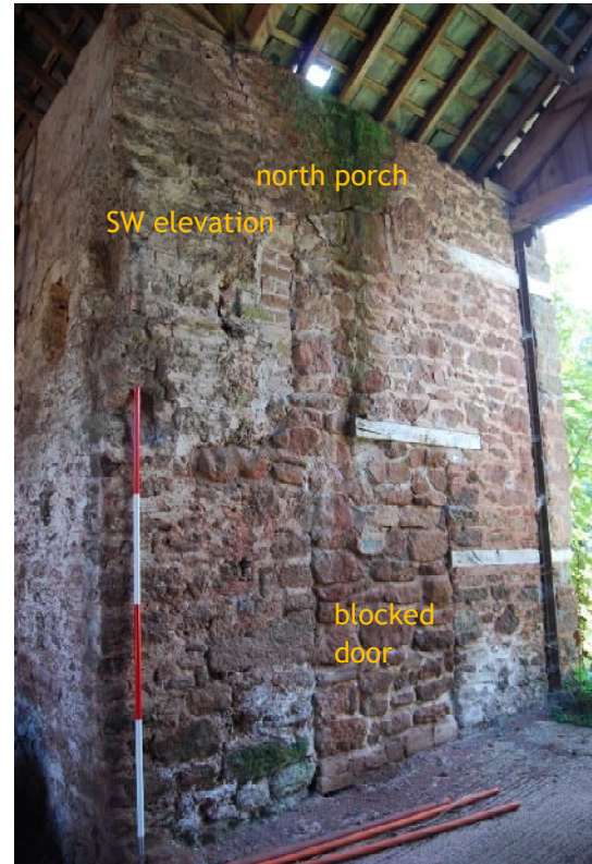
Plate 20. South-east side of north porch of B1, added to SW elevation (from WSE)
