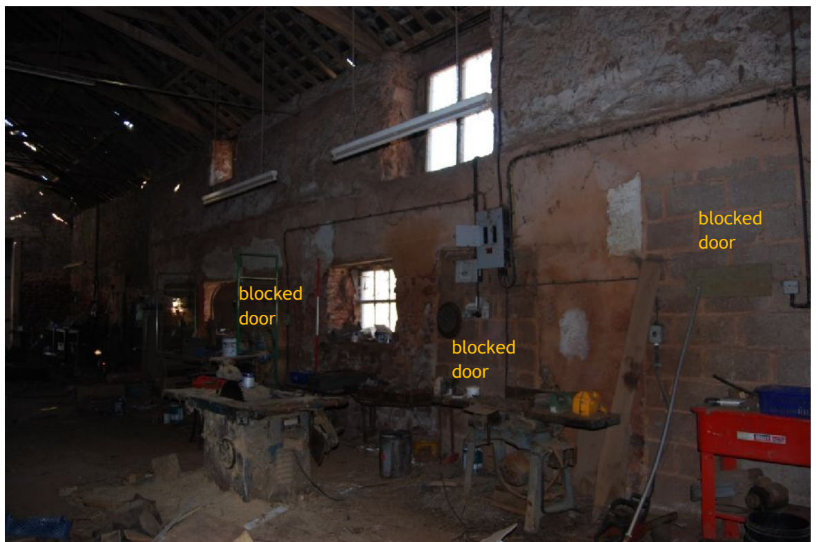
Plate 32. North-east interior elevation of B2 (from S; 2m scales)
