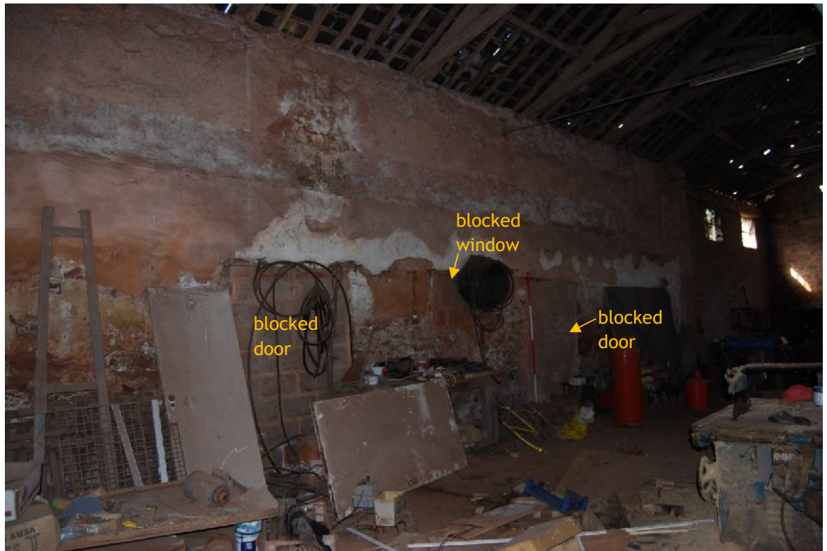
Plate 31. South-west interior elevation of B2 (from SE; 2m scales)
