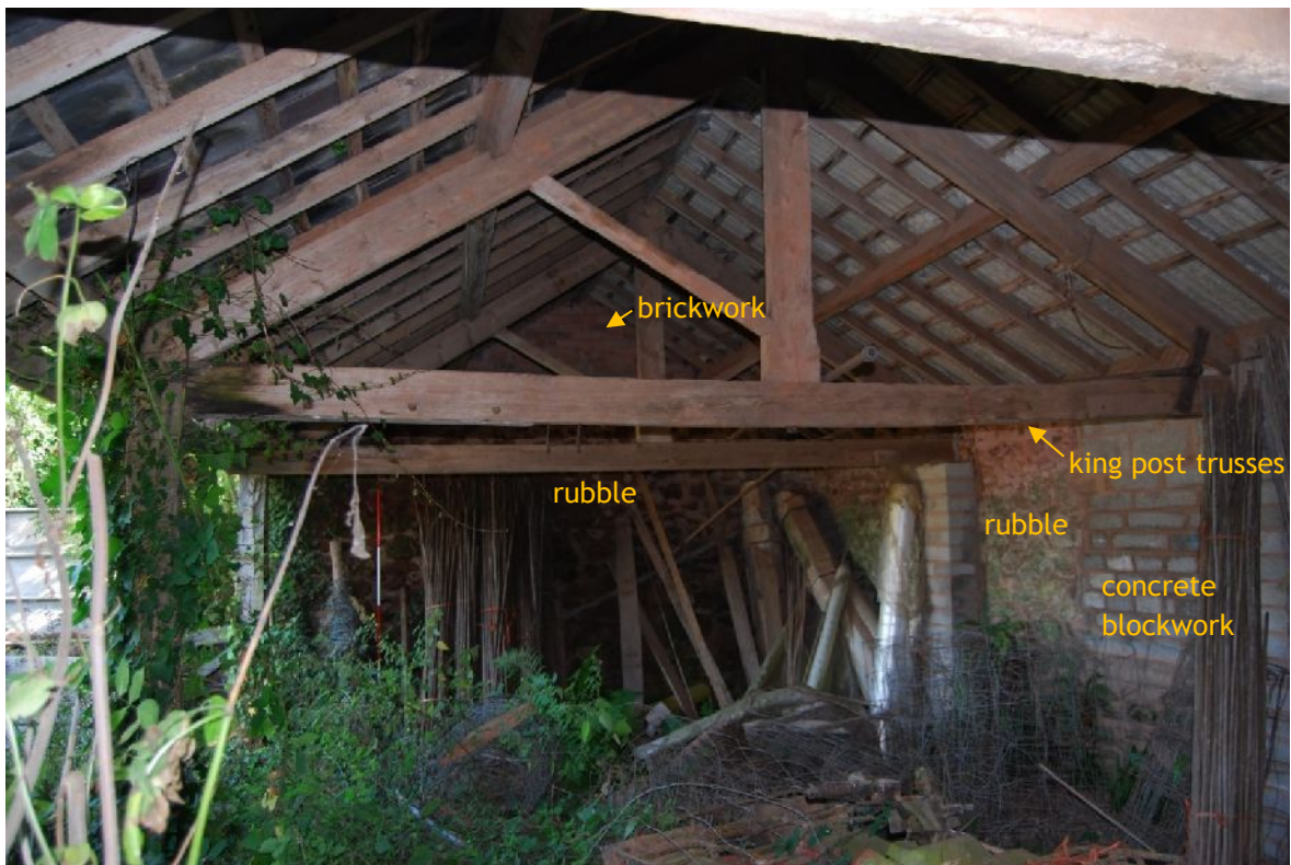
Plate 35. Interior of main part of B3 (from WSW; 2m scales) 0043
