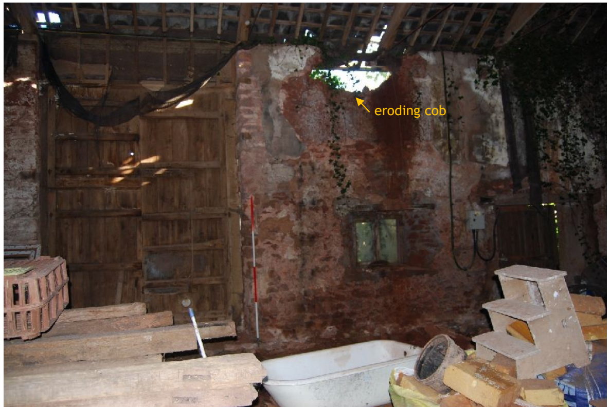
Plate 17. North-east interior elevation of B1 showing south full height door (from SW; 2m scales)
