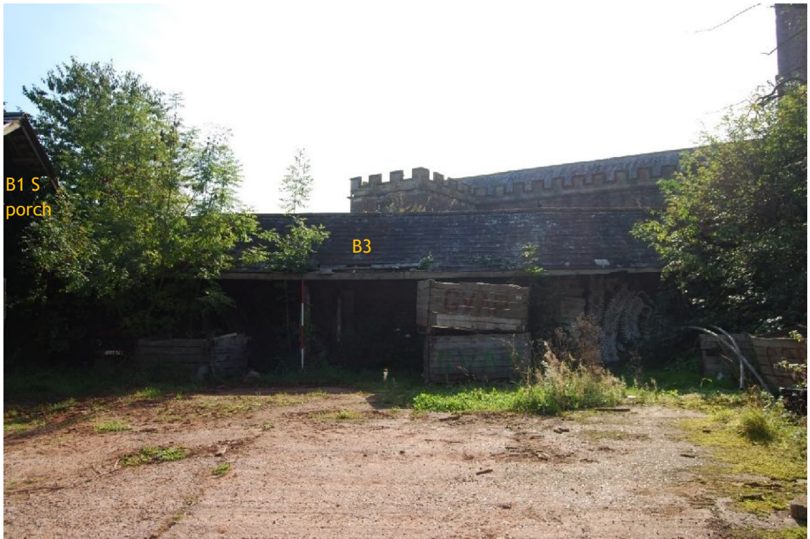
Plate 34. North-north-west side (open-fronted) of B3 (from NNW; 2m scales)
