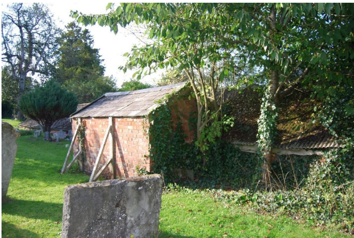
Plate 56. Graveyard outbuilding built on roof of B3 (from ESE)
