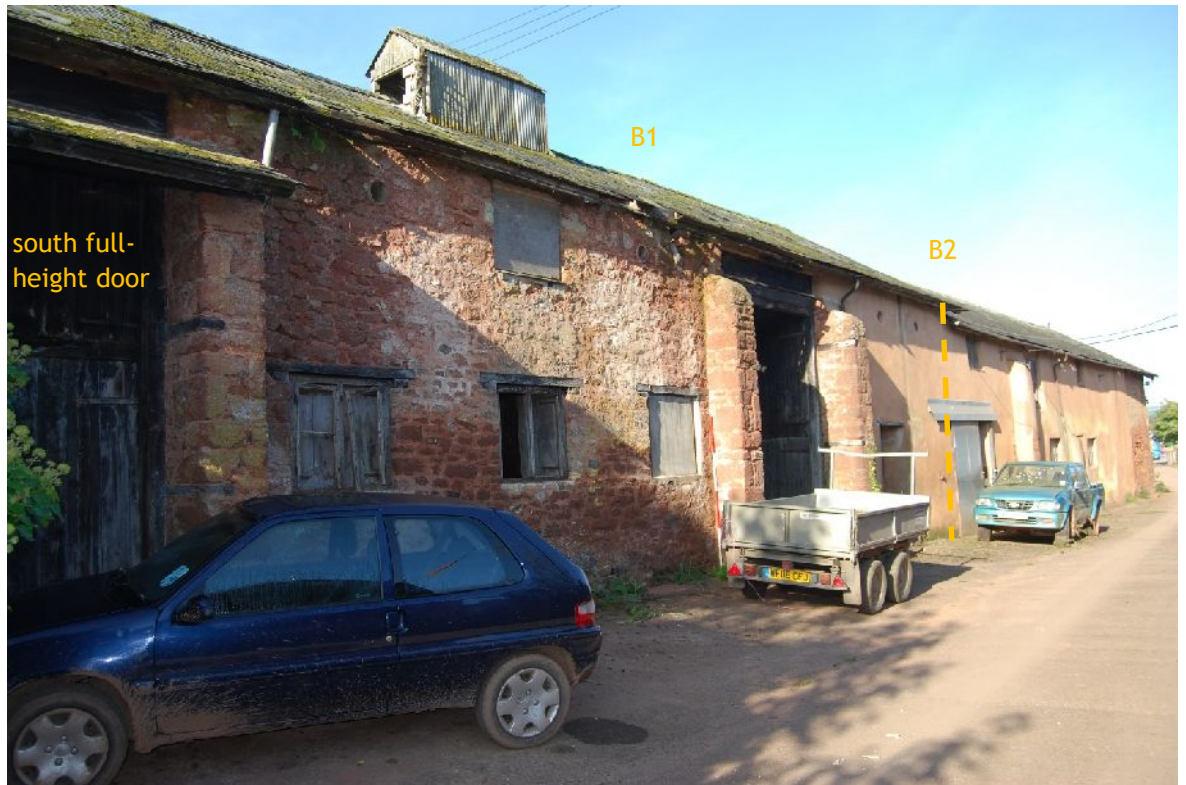
Plate 1. North-east elevation of B1 & B2 (from SE; 2m scales)
