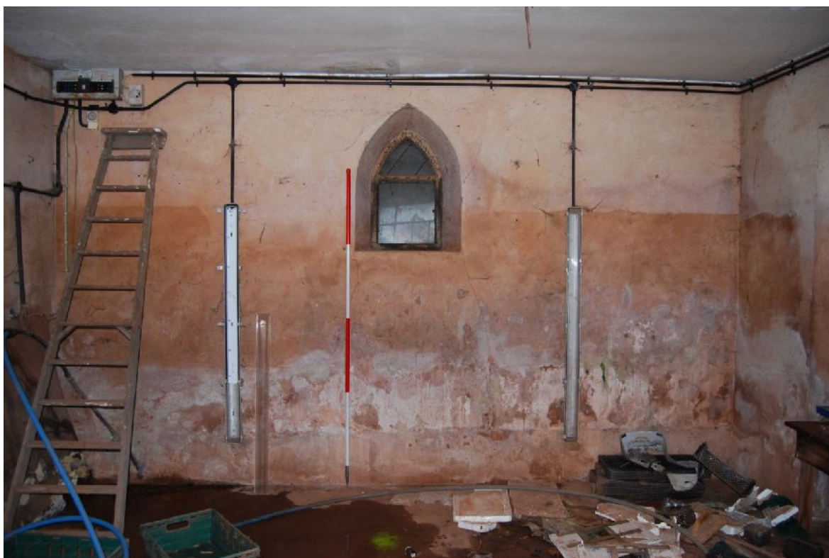
Plate 52. South-east interior elevation of B8 (from NW; 2m scales)
