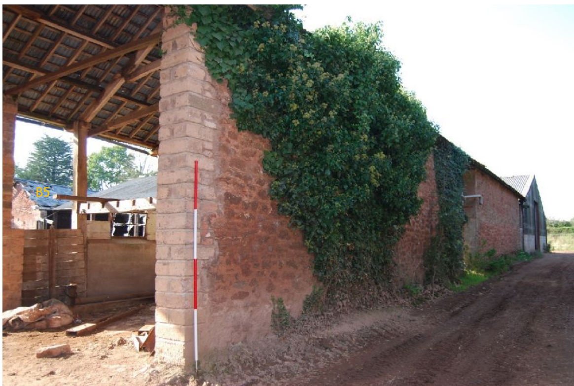
Plate 43. North-east exterior elevation of B6 (from SE; 2m scales)
