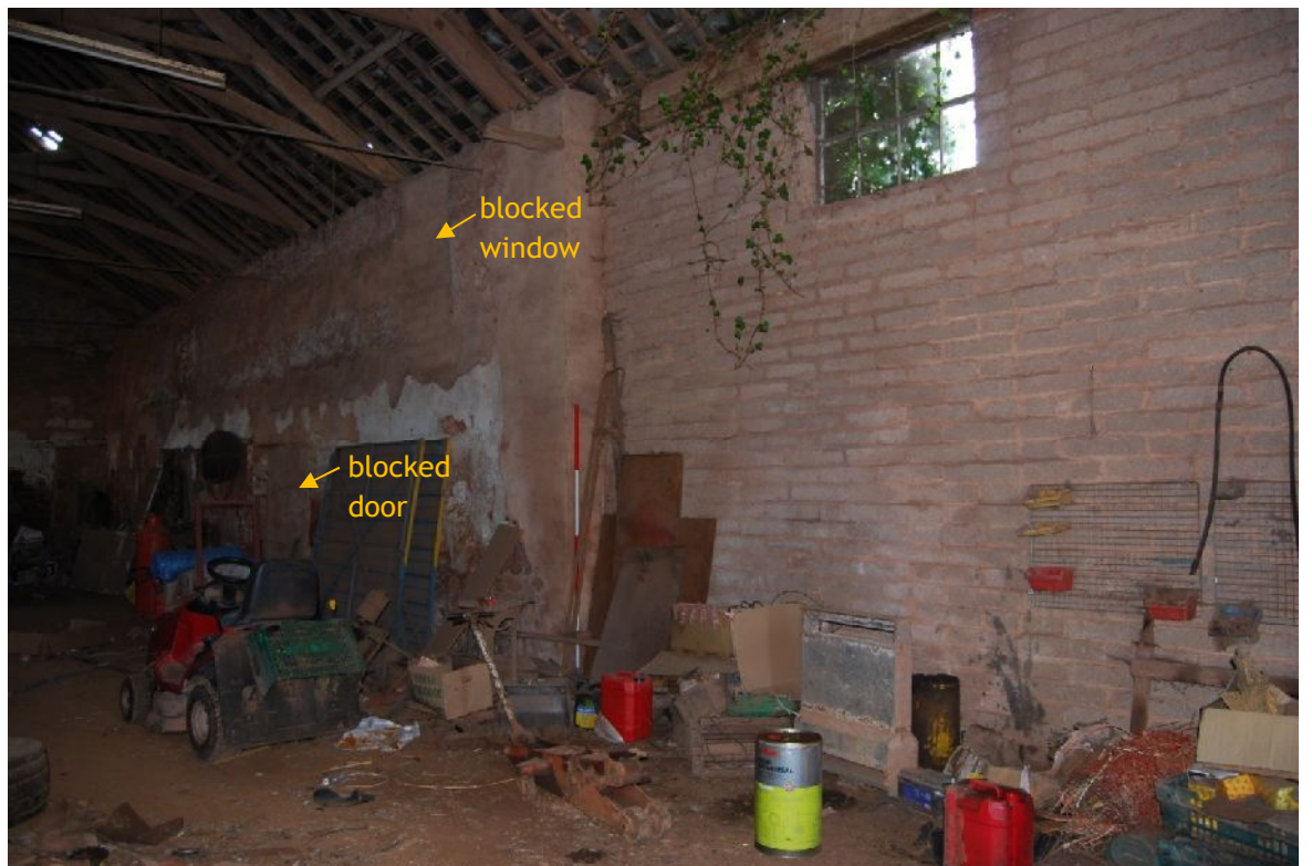
Plate 30. South-west interior elevation of B2 (from N; 2m scales)
