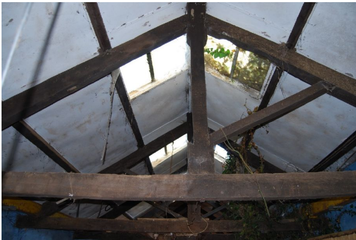
Plate 51. King post truss roof of B7 (from SW; 2m scales)
