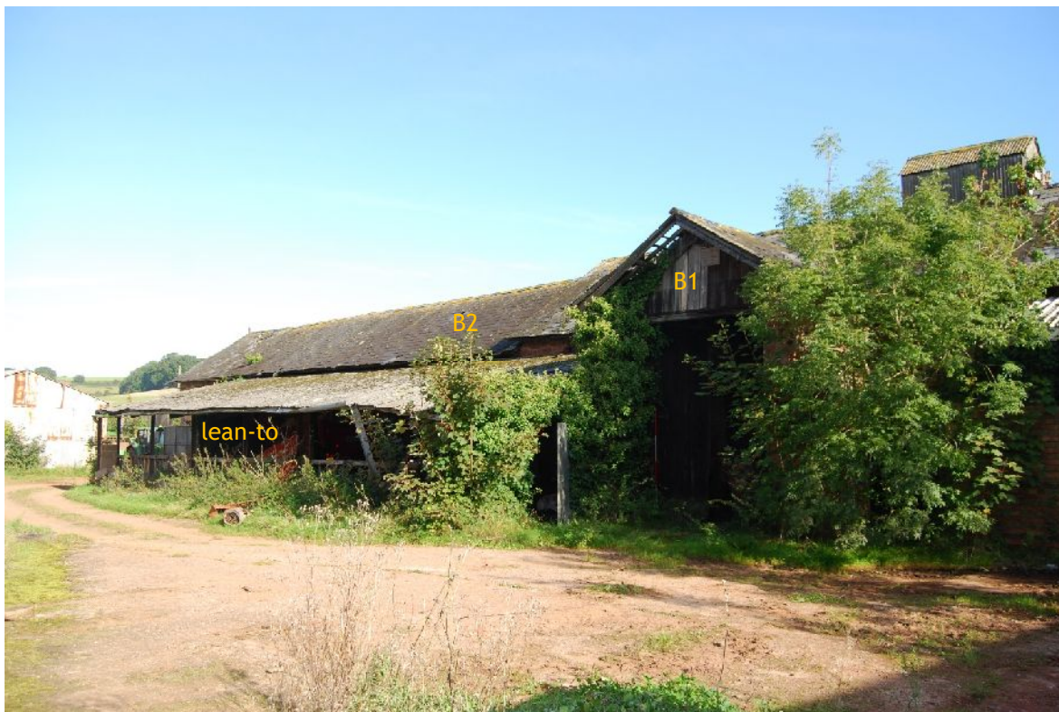
Plate 3. South-west elevation of B1 & B2 (from S; 2m scales)
