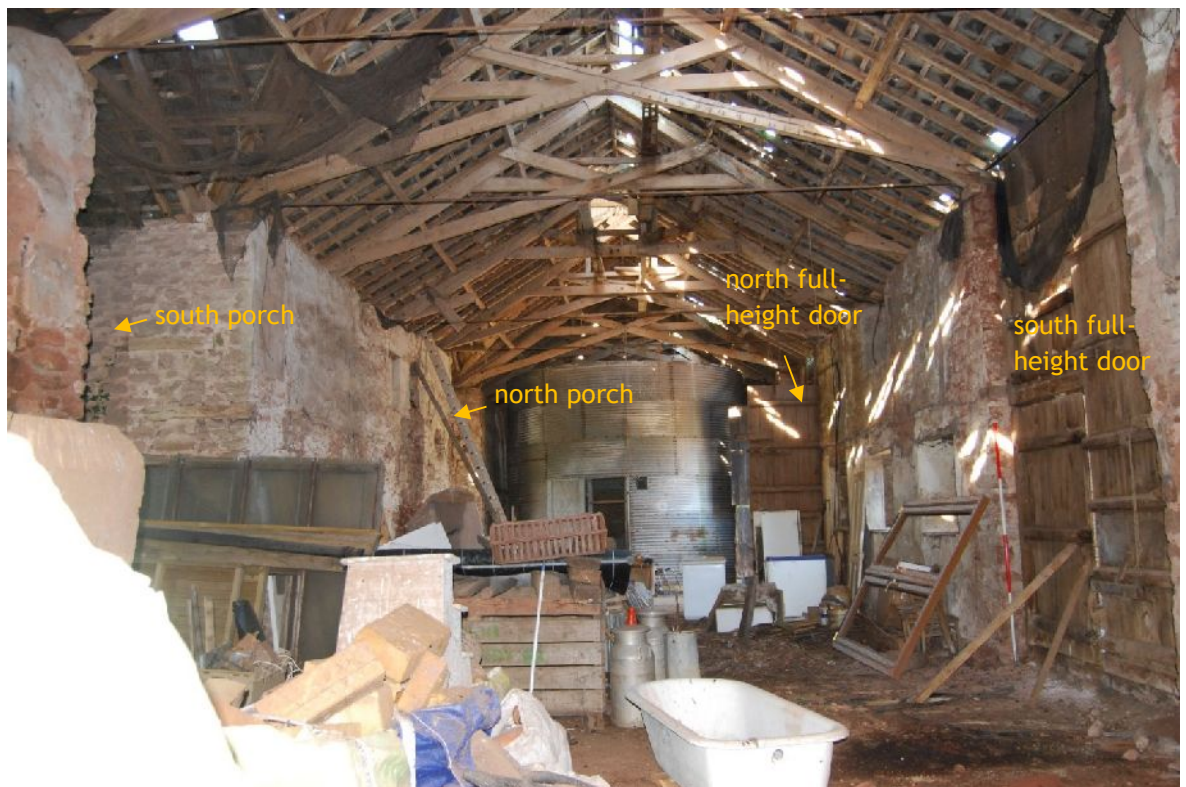
Plate 8. Interior of B1 showing scissor beam trusses (from SSE; 2m scales)
