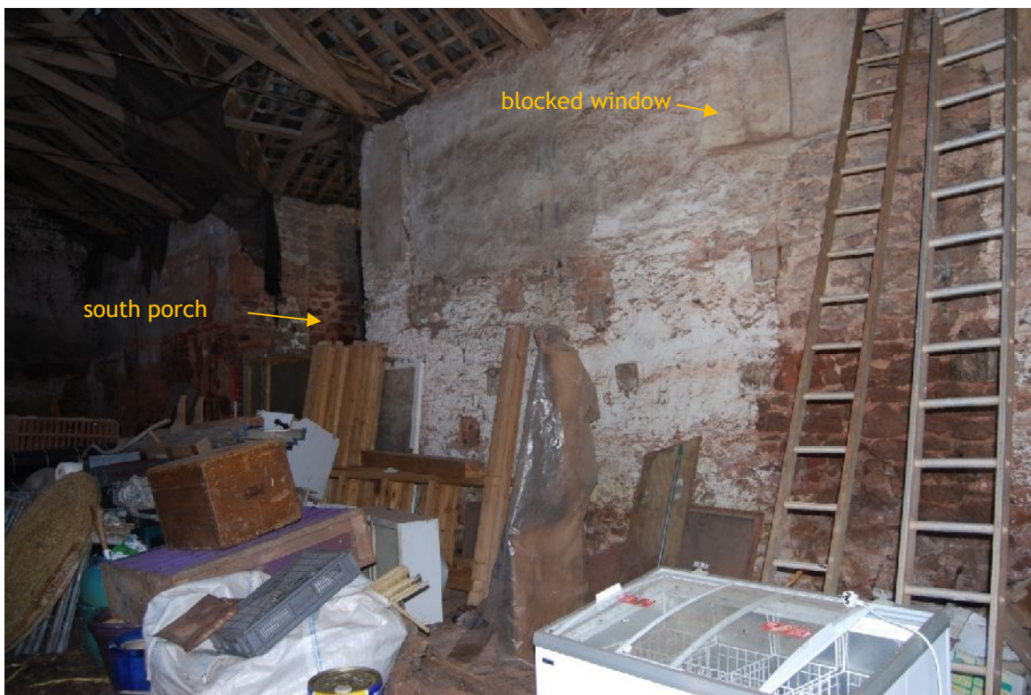
Plate 12. South-west interior elevation of B1 (from N; 2m scales)
