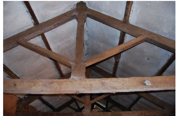
DSC 0099. Roof of B7 (from NE; 2m scales)
