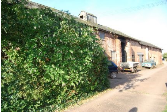
DSC 001. North-east elevation of B1 & B2 (from NE; 2m scales)
