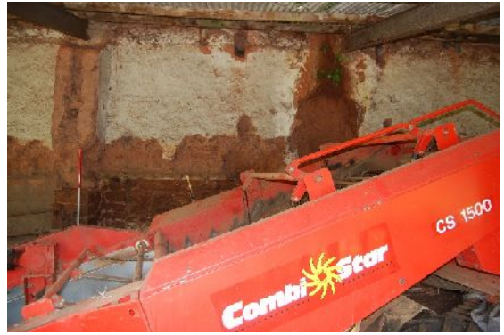
DSC 0026. South-west elevation of B2 (from SW; 2m scales)
