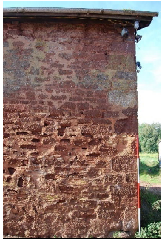
DSC 0018. North-east elevation of B2 (from NE; 2m scales)
