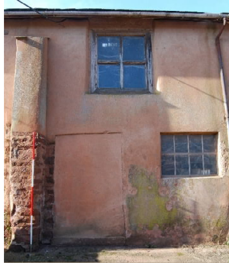
DSC 0012. North-east elevation of B2 (from NE; 2m scales)
