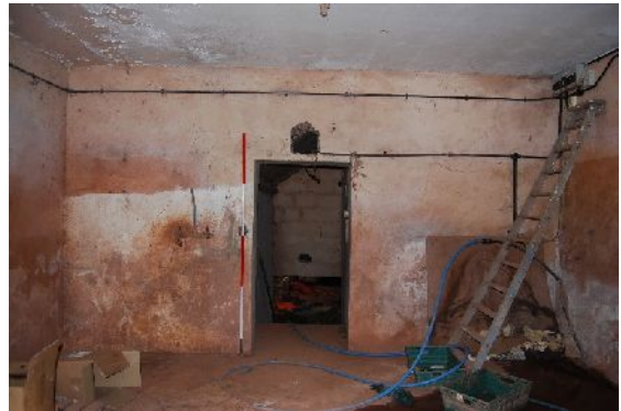
DSC 0092. North-east interior elevation of B8 (from SW; 2m scales)
