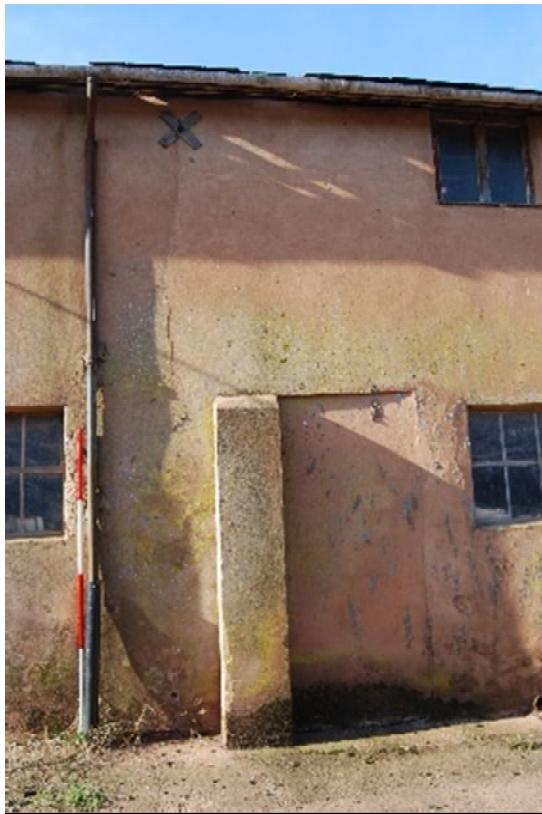
DSC 0013. North-east elevation of B2 (from NE; 2m scales)
