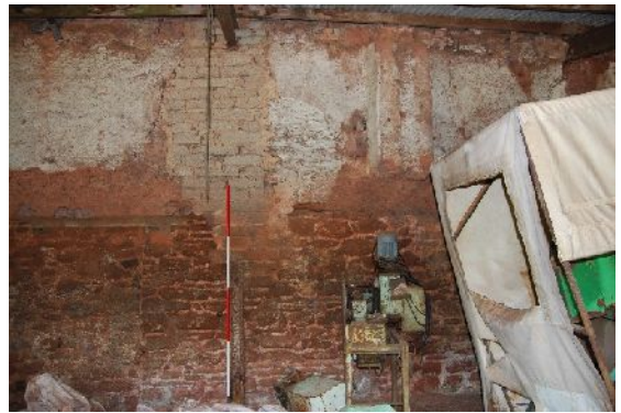
DSC 0029. South-west elevation of B2 (from SW; 2m scales)
