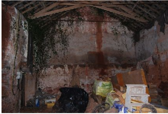
DSC 0063. South-east interior gable end of B1 (from NW; 2m scales)
