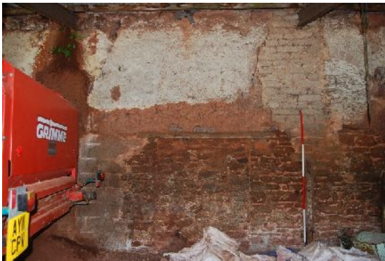
DSC 0027. South-west elevation of B2 (from SW; 2m scales)
