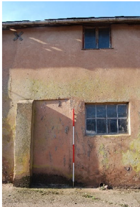
DSC 0014. North-east elevation of B2 (from NE; 2m scales)
