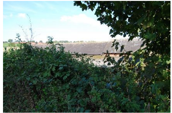
DSC 0121. View of B1 & B2 roofs from graveyard (from SSW)
