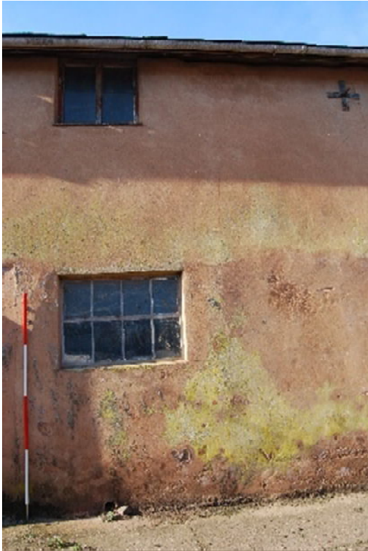
DSC 0015. North-east elevation of B2 (from NE; 2m scales)
