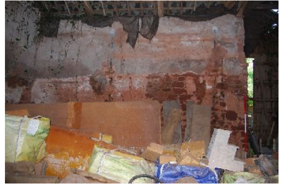
DSC 0052. Interior of southern end of B1 (from NE; 2m scales)
