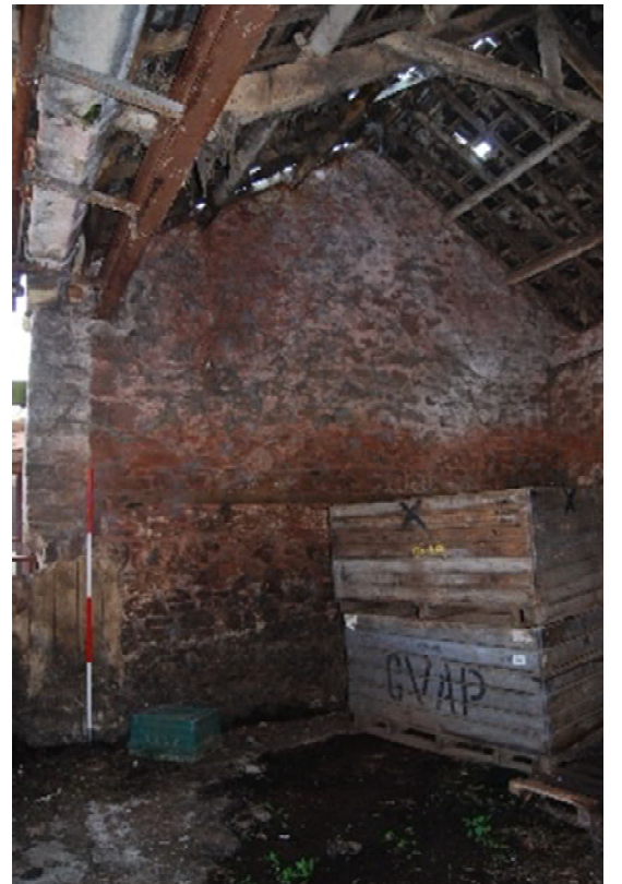
DSC 0102. South-east interior gable elevation of B5 (from N; 2m scales)
