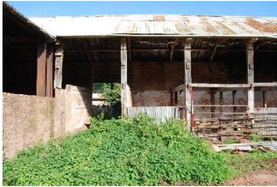
DSC 0108. North-east interior elevation of B6, central (from SW; 2m scales)
