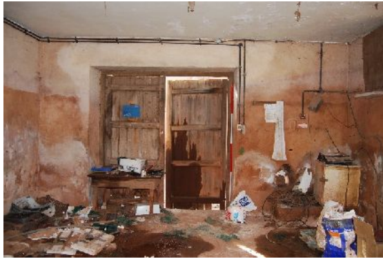
DSC 0094. South-west interior elevation of B8 (from NE; 2m scales)
