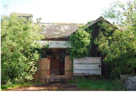
DSC 0037. South-west elevation of B1 showing southern-most full height door (from SW; 2m scales)
