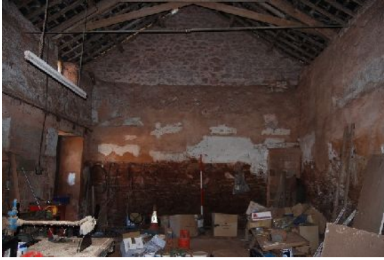
DSC 0077. South-east interior gable elevation of B2 (from NW; 2m scales)
