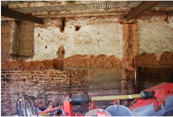
DSC 0025. South-west elevation of B2 (from SW; 2m scales)
