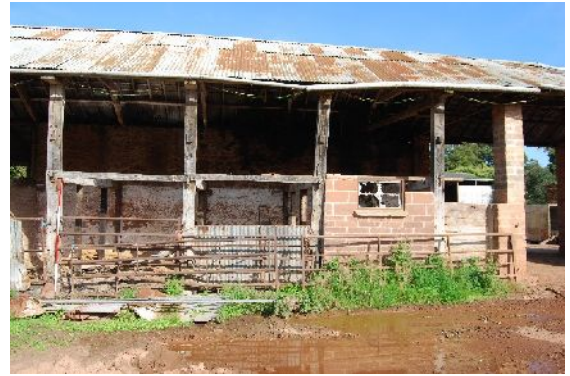
DSC 0109. North-east interior elevation of B6, central (from SW; 2m scales)
