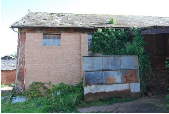
DSC 0020. South-west elevation of B2 (from SW; 2m scales)
