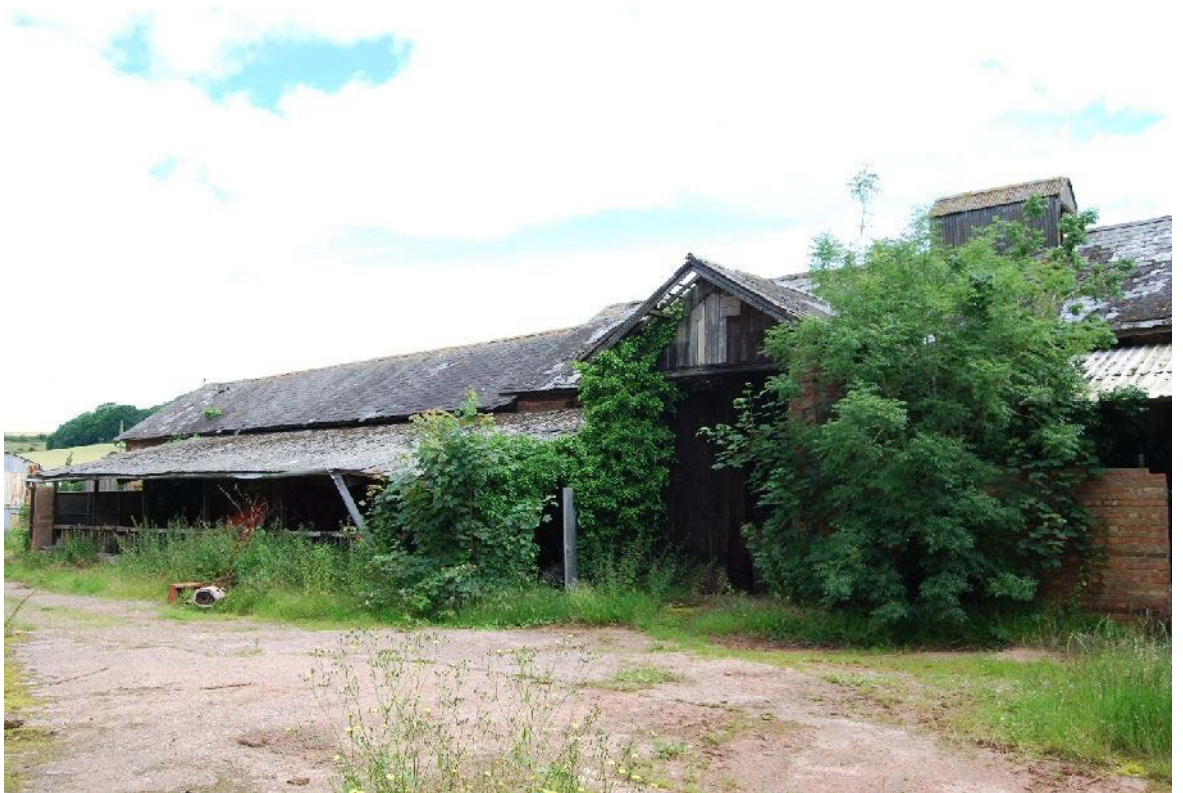
Plate 9. The historic barn on the southern portion of the Site (from SSW), showing the gabled barn entrance and additional sheds along the western wall
