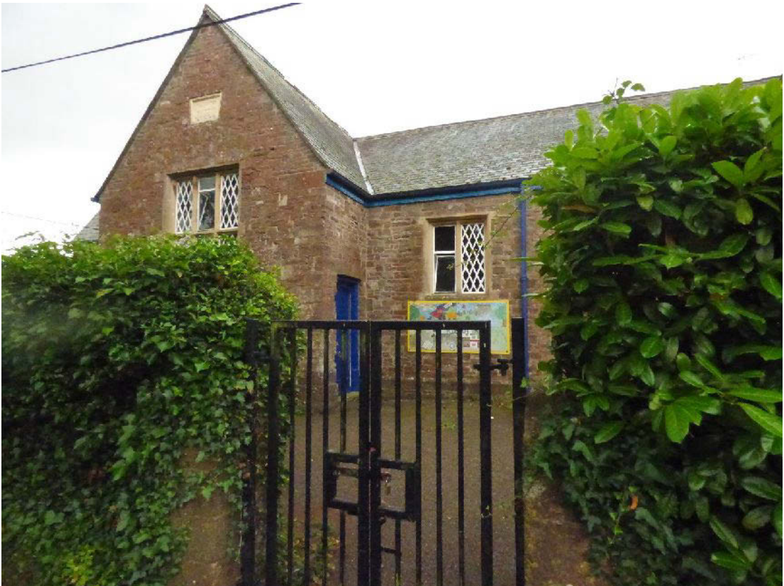
Plate 24. The entrance from Church Path to Grade II Listed Halberton School (No 13) (from N)
