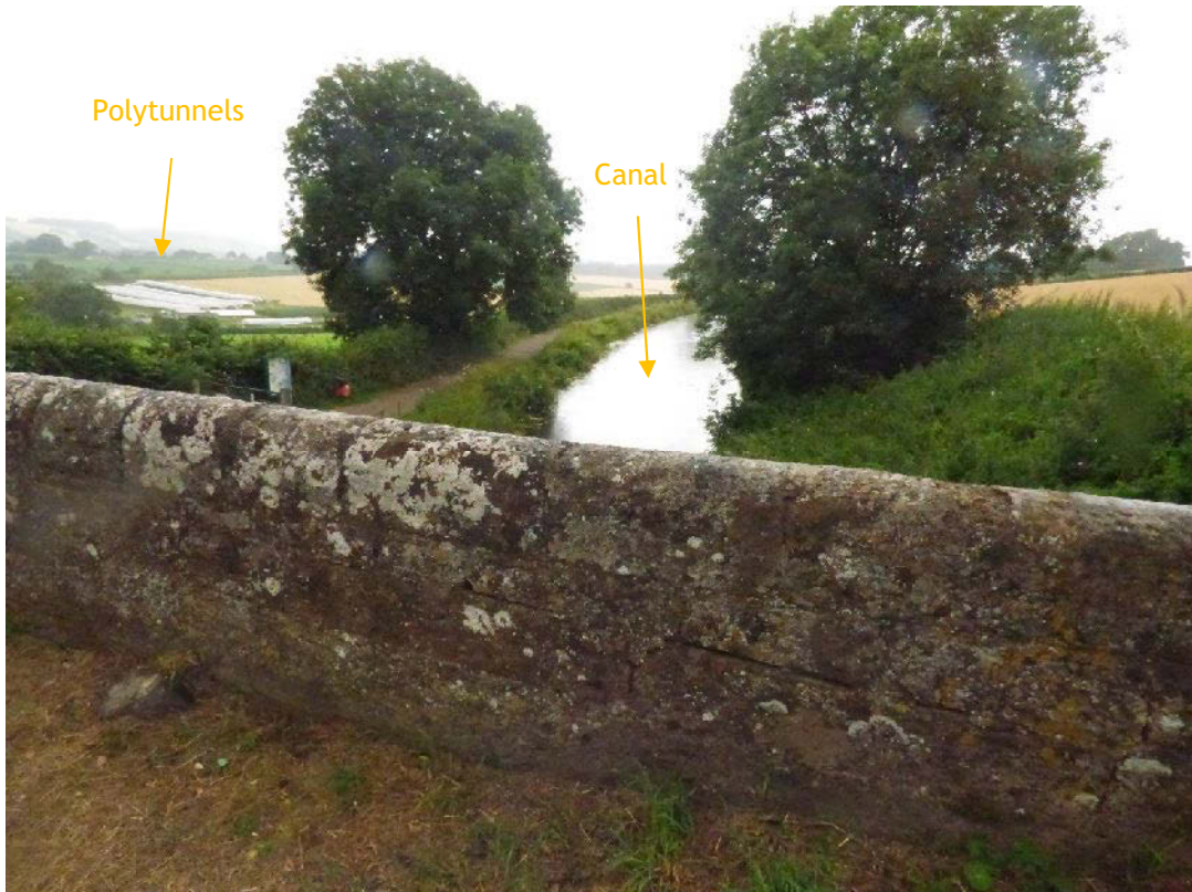
Plate 46. Greenway Bridge (Figure 2 No 46; from SE) and the Great Western Canal
