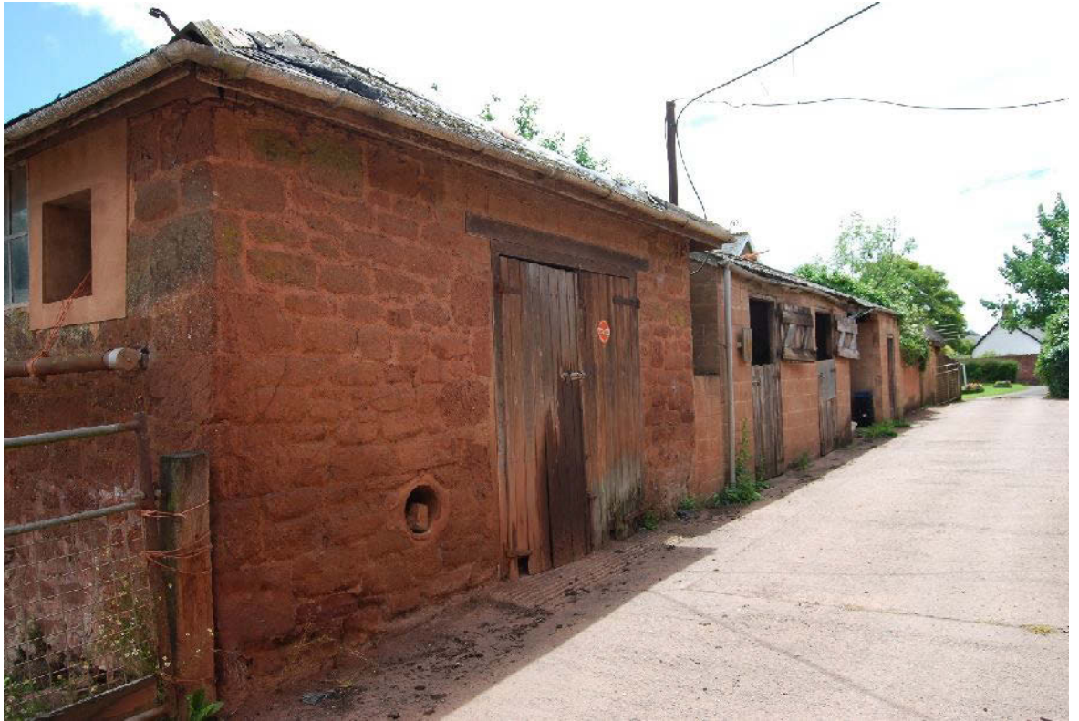
Plate 12. The south-western corner of the 'courtyard' with associated stables and sheds to the south (from NW)
