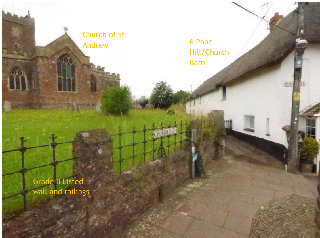
Plate 31. Grade II Listed No 6 Pond Hill/Church Barn (Figure 5 Nos 8 & 9) (from S)
