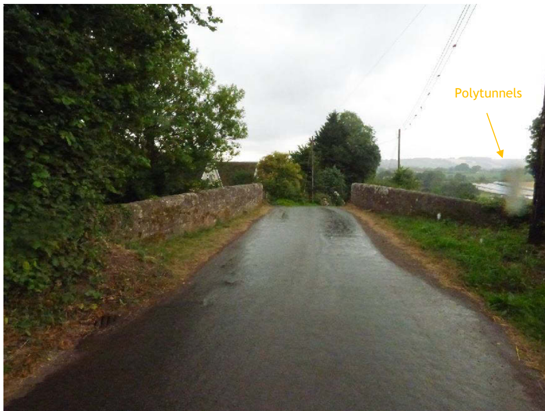
Plate 45. The Greenway Bridge (Figure 5 No 1; from E)
