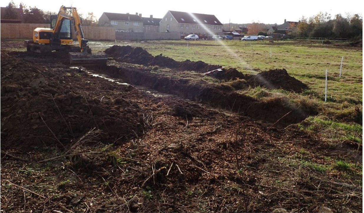
Plate 3: Trench 4 during excavation (no scale)
