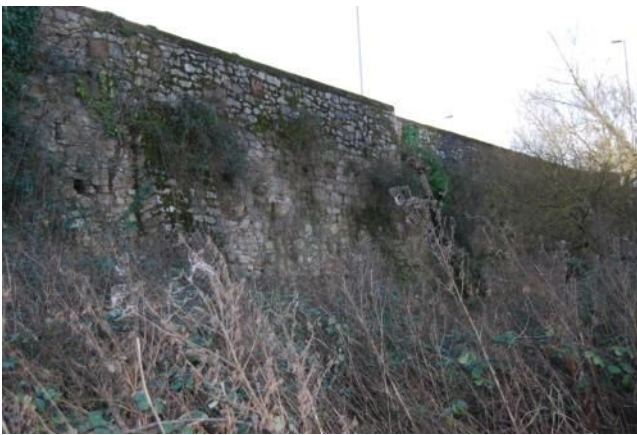
Plate 14. Buttresses at eastern end of upstream elevation (looking S)
