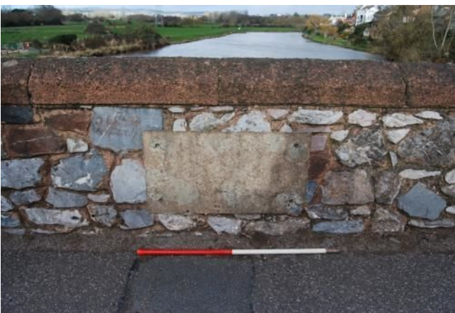
Plate 18. Backing stone for plaque, upstream parapet (looking NW) (1m scale)
