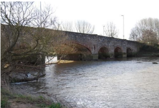
Plate 8. Upstream elevation (looking SW)
