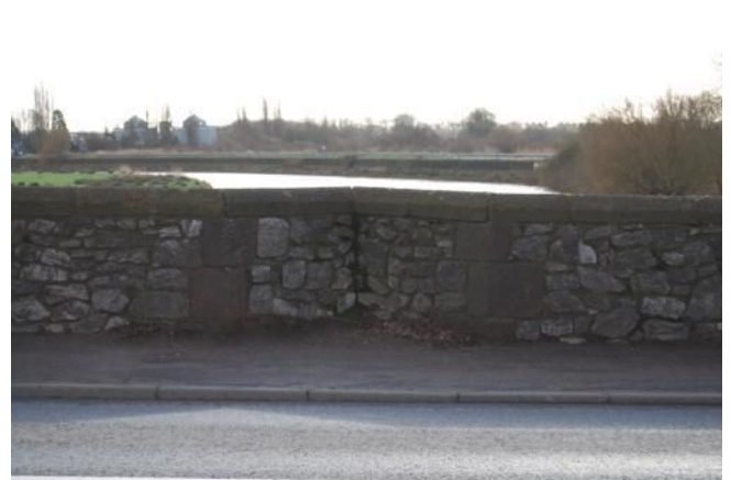
Plate 21. Refuge, downstream parapet (looking SE)
