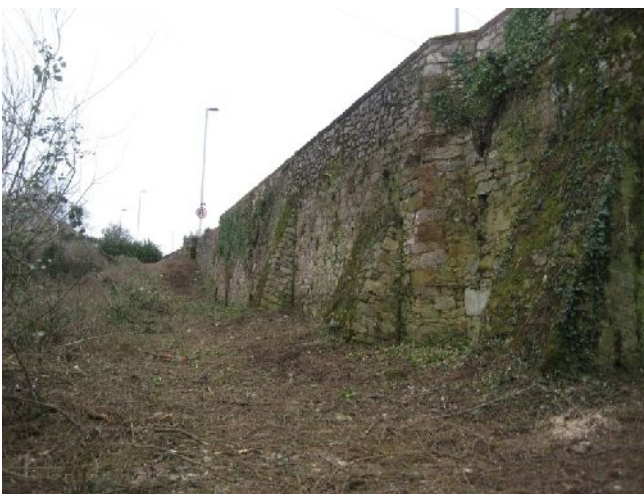
Plate 26. Eastern end of upstream elevation (looking NEE)
