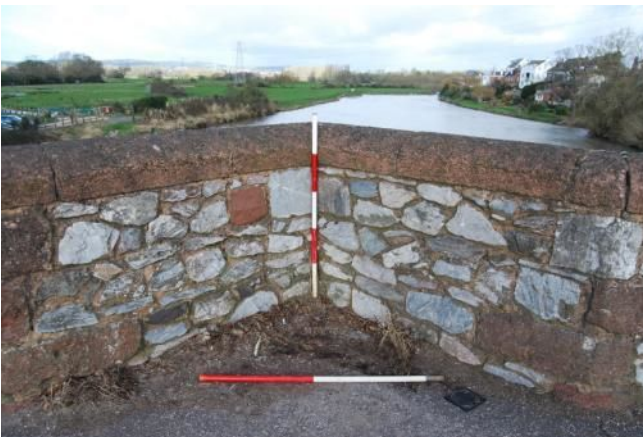
Plate 20. Refuge, upstream parapet (looking NW)
