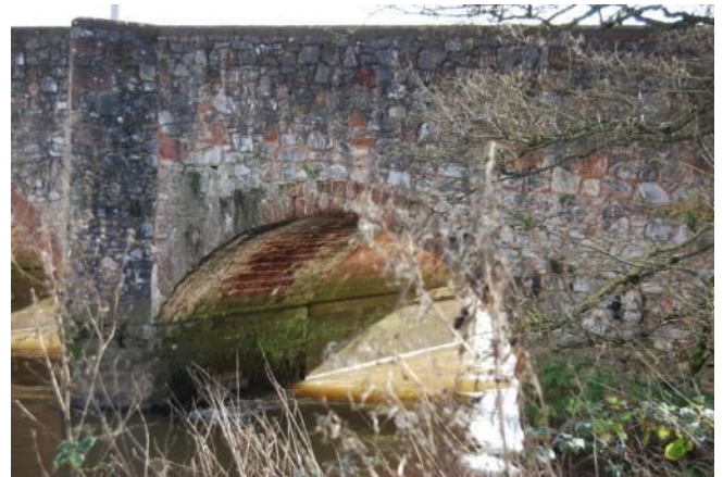
Plate 13. Western arch, upstream elevation (looking SE)
