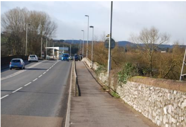
Plate 6. Upstream side of carriageway across bridge (looking SW)
