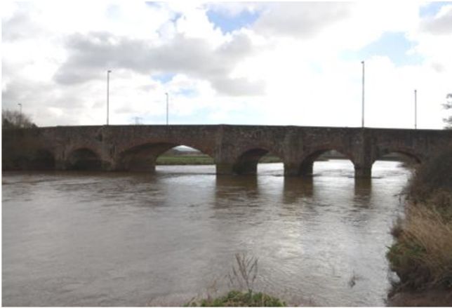
Plate 4. Upstream elevation (looking SE)
