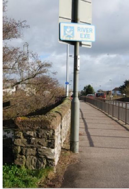
Plate 23. South-west approach to bridge, upstream parapet (looking NE)
