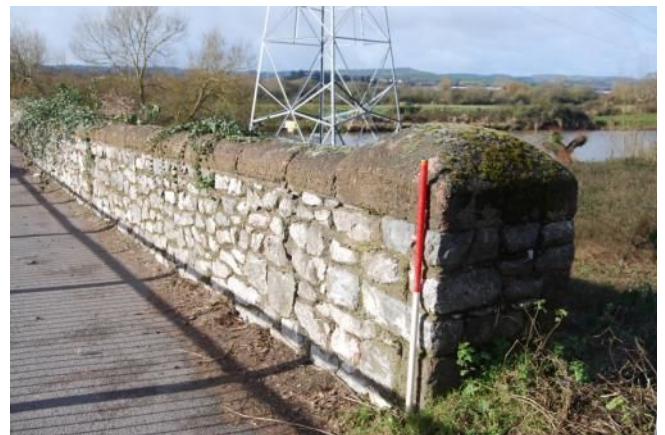
Plate 15. West side of entranceway, upstream parapet (looking W)
