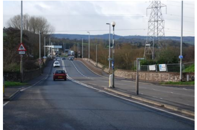
Plate 5. Carriageway across bridge (looking SW)
