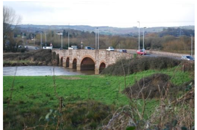
Plate 7. Downstream elevation (looking NWW)
