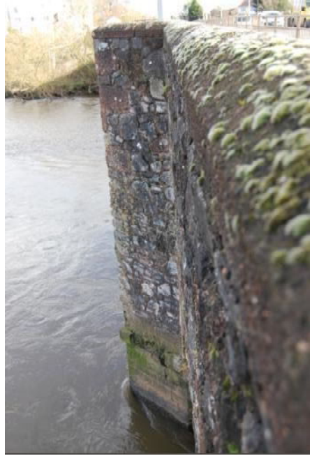
Plate 11. Cutwater Type B, upstream elevation (looking NE)
