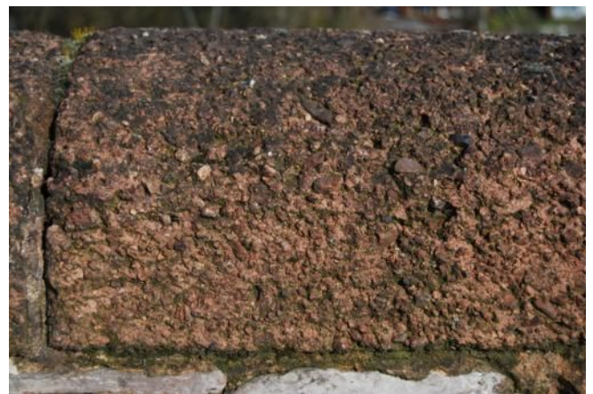
Plate 19. Red cement coping, upstream parapet (looking NW)
