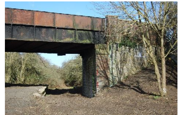
South elevation – east embankment (from S)
