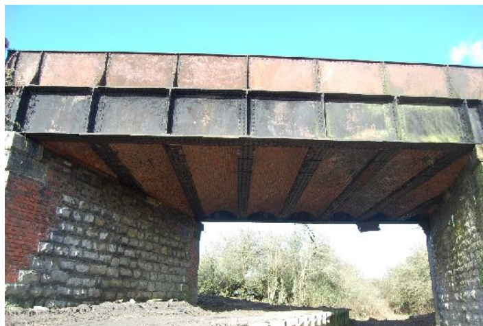
Plate 16. Underside & parapet, looking NW
