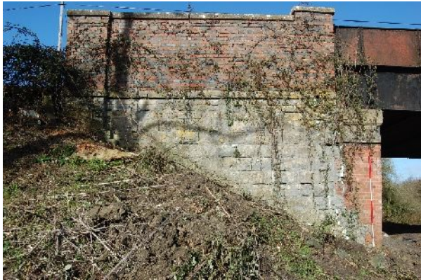
South elevation – west embankment (from SSE)
