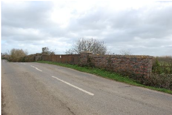
South parapet of bridge (from SW)
