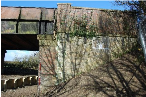
South elevation – east embankment (from SSE)
