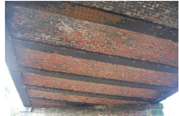
Underside of bridge (from NNE)
