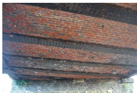
Plate 18. Underside, looking NE
