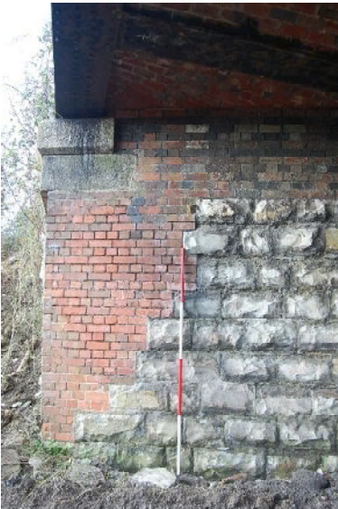
West abutment - south end (from NNE)
