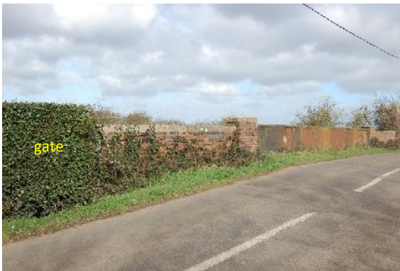
Plate 6. North side of bridge parapet from road, looking N
