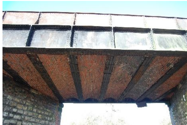
Underside of bridge (from SSE)
