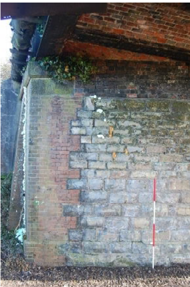
East abutment - north end (from SSW)
