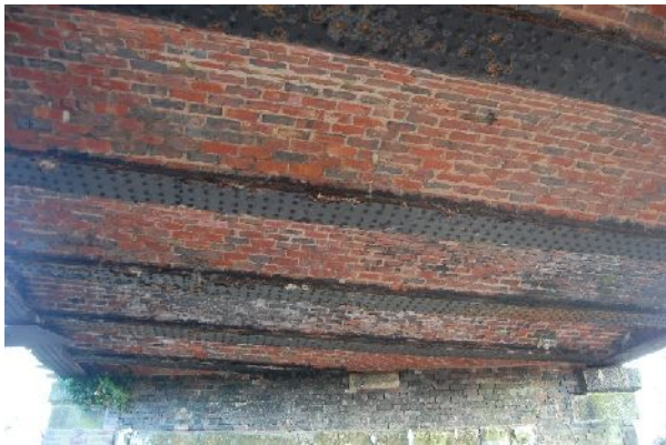
Underside of bridge (from SSW)
