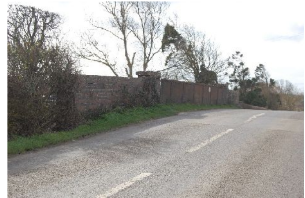
South parapet of bridge (from NNE)
