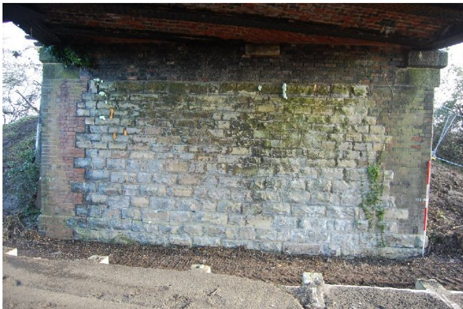
Plate 15. East abutment & platform, looking NE (2m scale)
