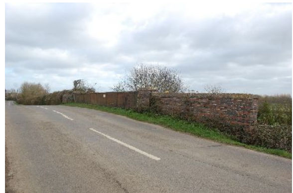
Plate 7. South side of bridge parapet from road, looking ENE
