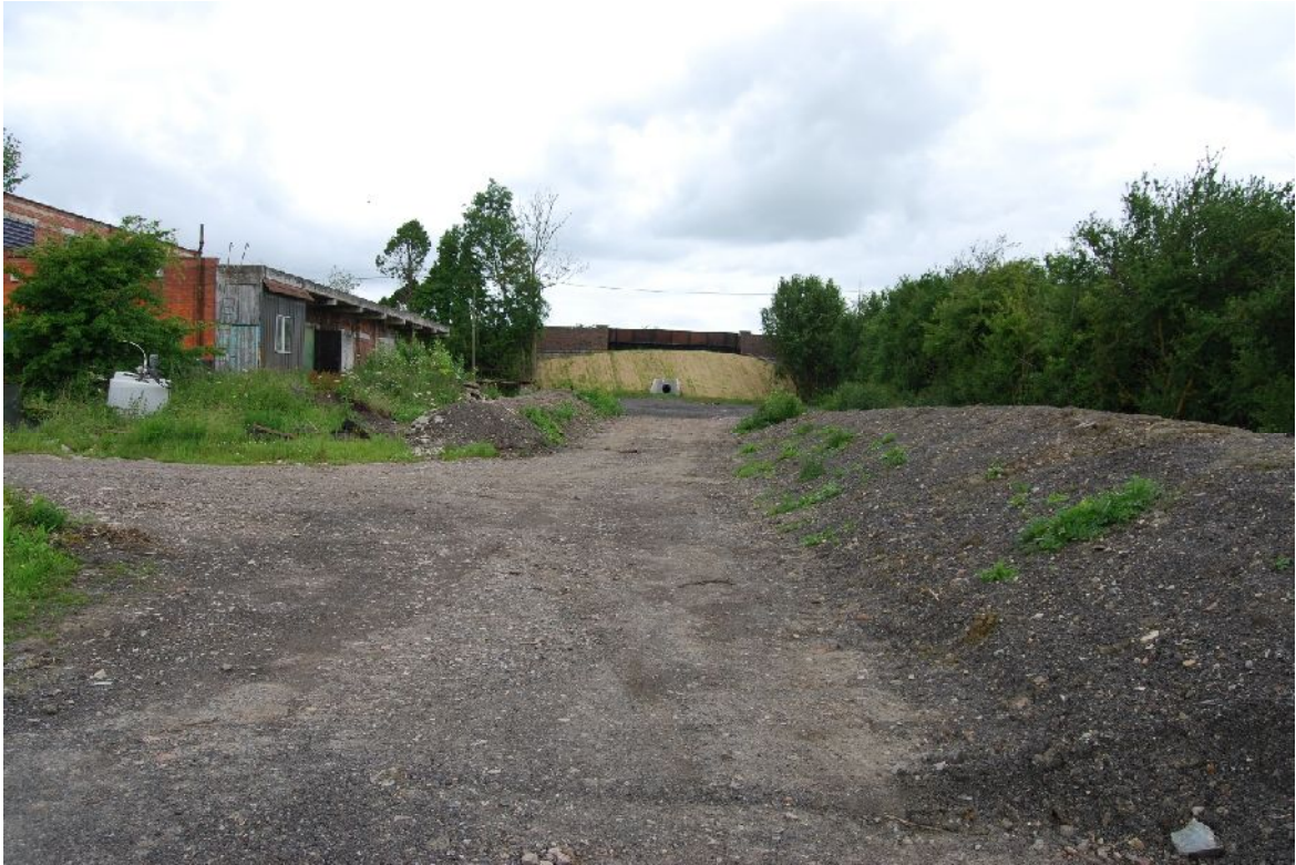
Plate 23. South elevation following infilling with former Nestle siding, looking NW
