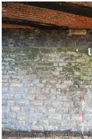
East abutment – central (from SSW)
