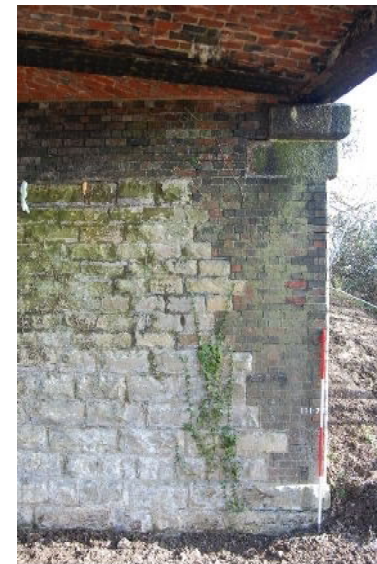
East abutment - south end (note benchmark next to scale) (from SSW)
