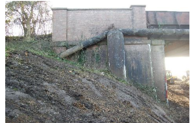
North elevation – east embankment (from NNW)
