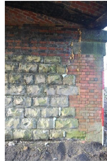
West abutment - north end (from NNE)
