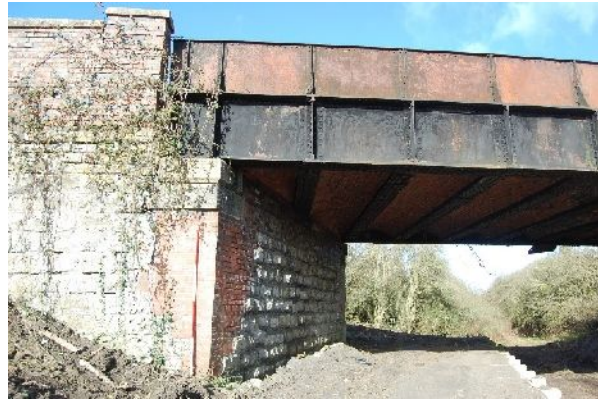
South elevation – west embankment & bridge (from SSE)
