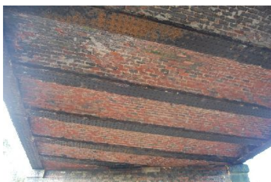
Plate 17. Underside, looking SW
