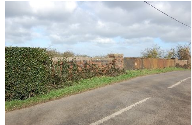
North parapet of bridge (from S)
