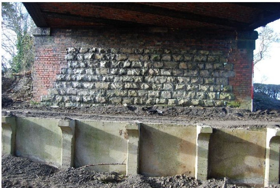
Plate 14. West abutment & platform, looking SW (2m scale)
