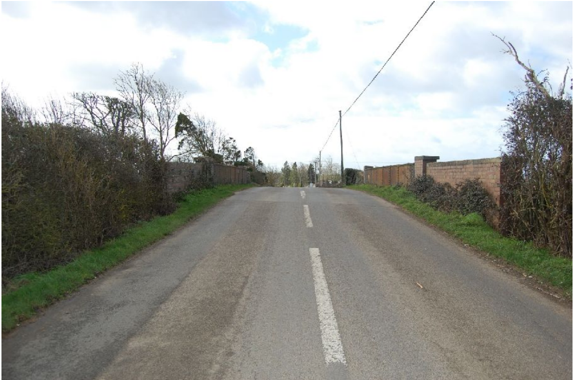
Plate 5. View along road above bridge, looking SW
