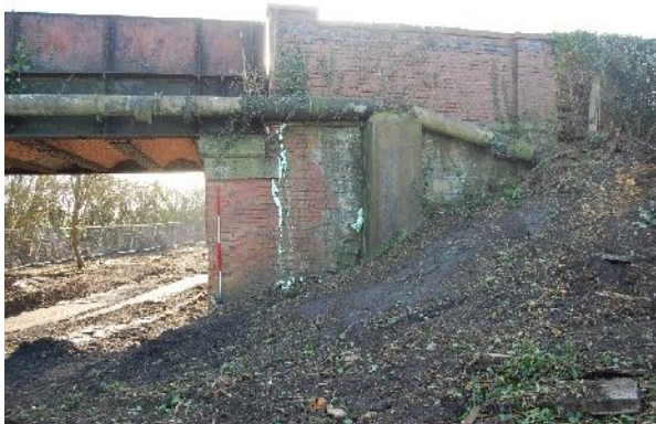
North elevation – west embankment (from NNW)
