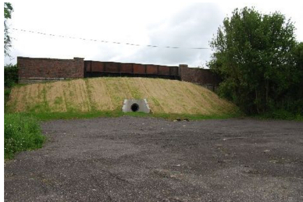
Completion shot of south elevation (from S)
