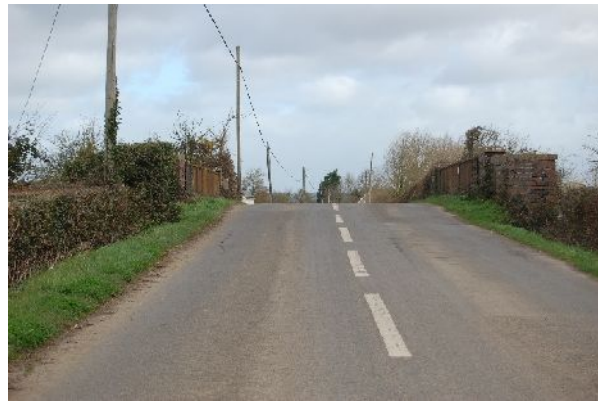
Road over bridge (from SSW)
