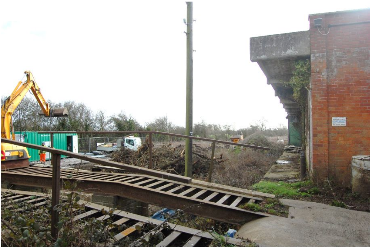
Plate 20. Former Nestlé building with platform, siding & loading ramp, looking SE
