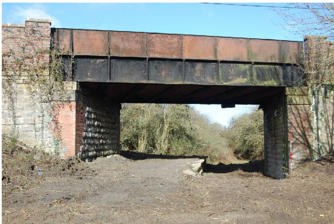
Plate 4. South elevation, looking NW (2m scale)
