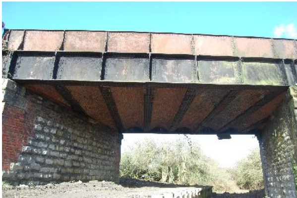
Underside of bridge (from SSE)
