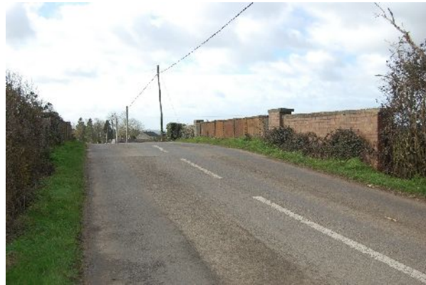
North parapet of bridge (from NE)
