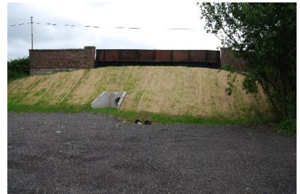
Completion shot of south elevation (from SE)
