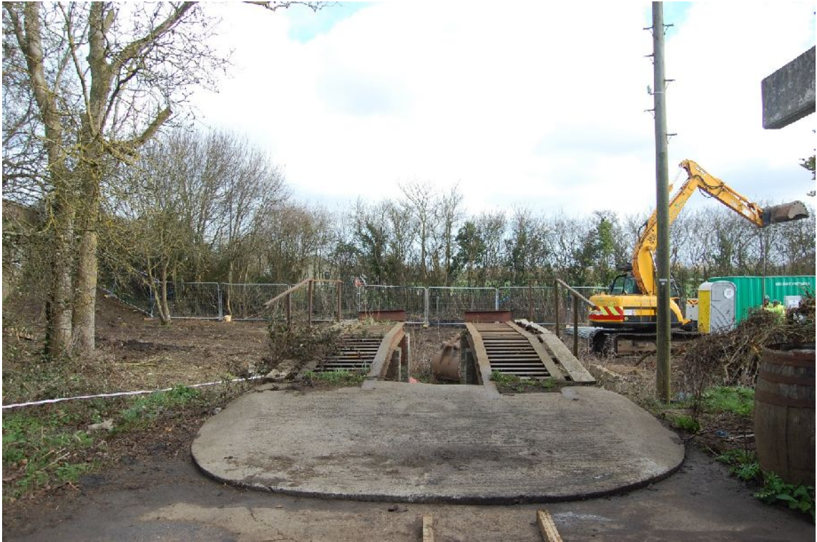
Plate 21. Former Nestle loading ramp, looking ENE
