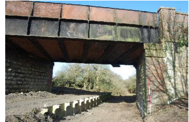
South elevation – east embankment & bridge (from SSE)
