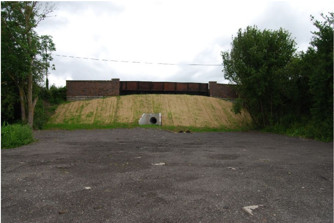
Plate 24. South elevation following infilling, looking NW
