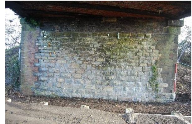
East abutment wall & platform edge (benchmark next to scale) (from SSW)
