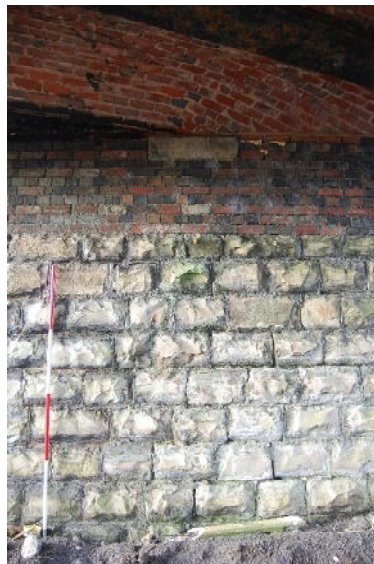
West abutment – central (from NNE)
