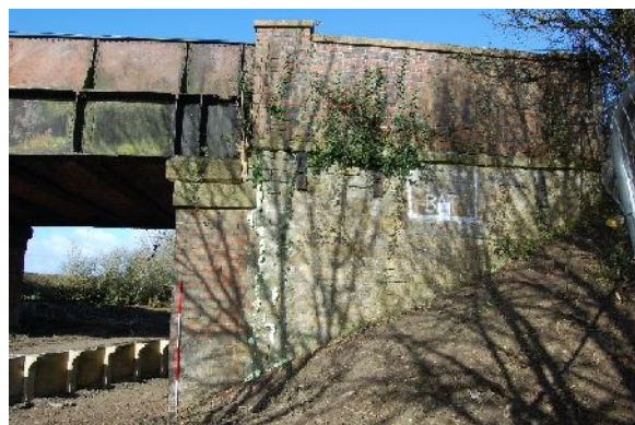
Plate 13. East side of south elevation, looking NW (2m scale)
