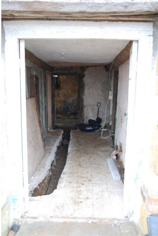
Plate 2. Test trench in cross-passage from NE (no scale) (Profile 1)
