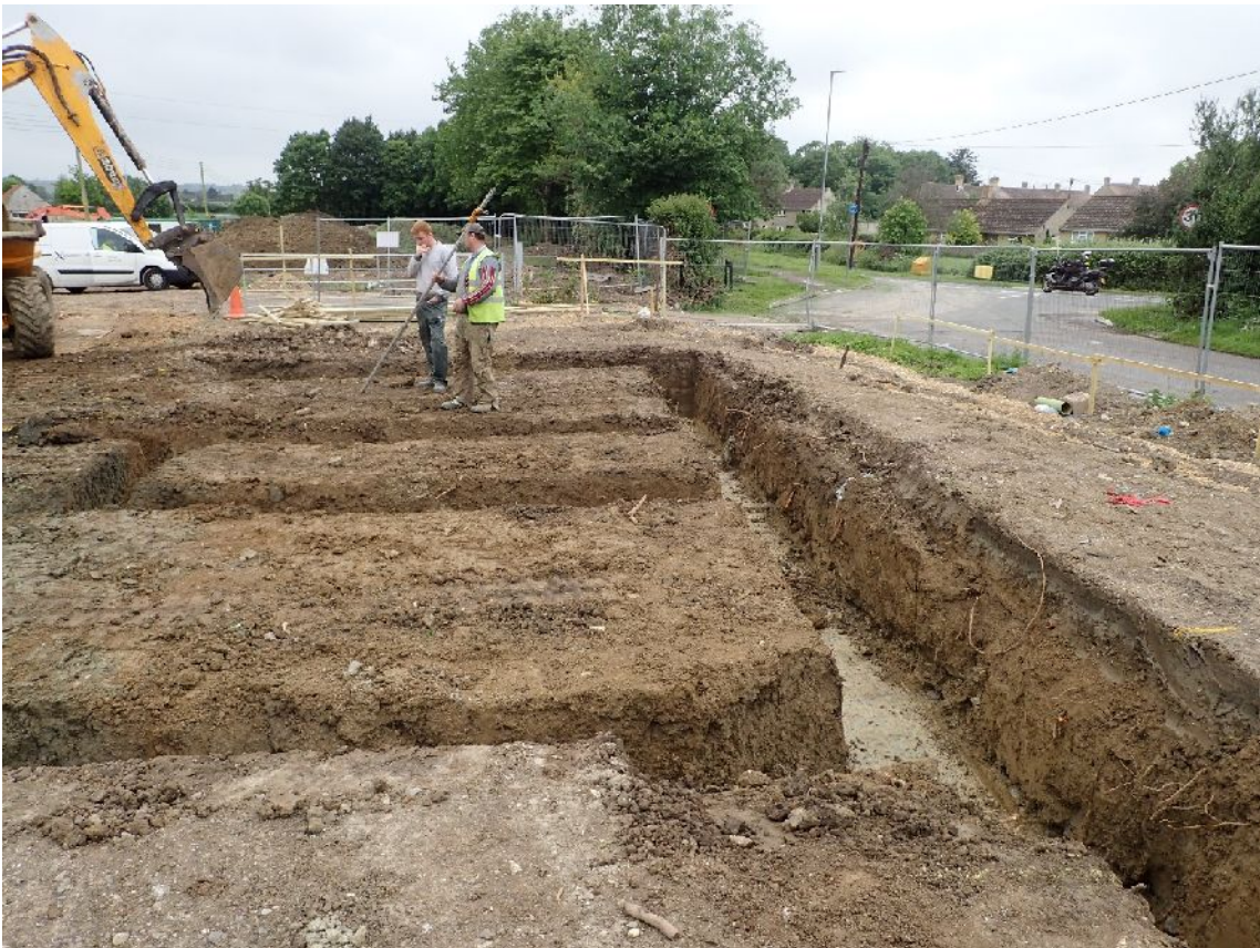
Plate 2. Working shot: excavation of foundation trenches (from N, no scale)
