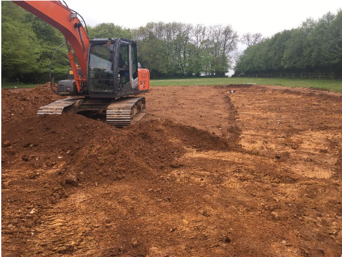
Plate 1. Working shot during removal of topsoil
