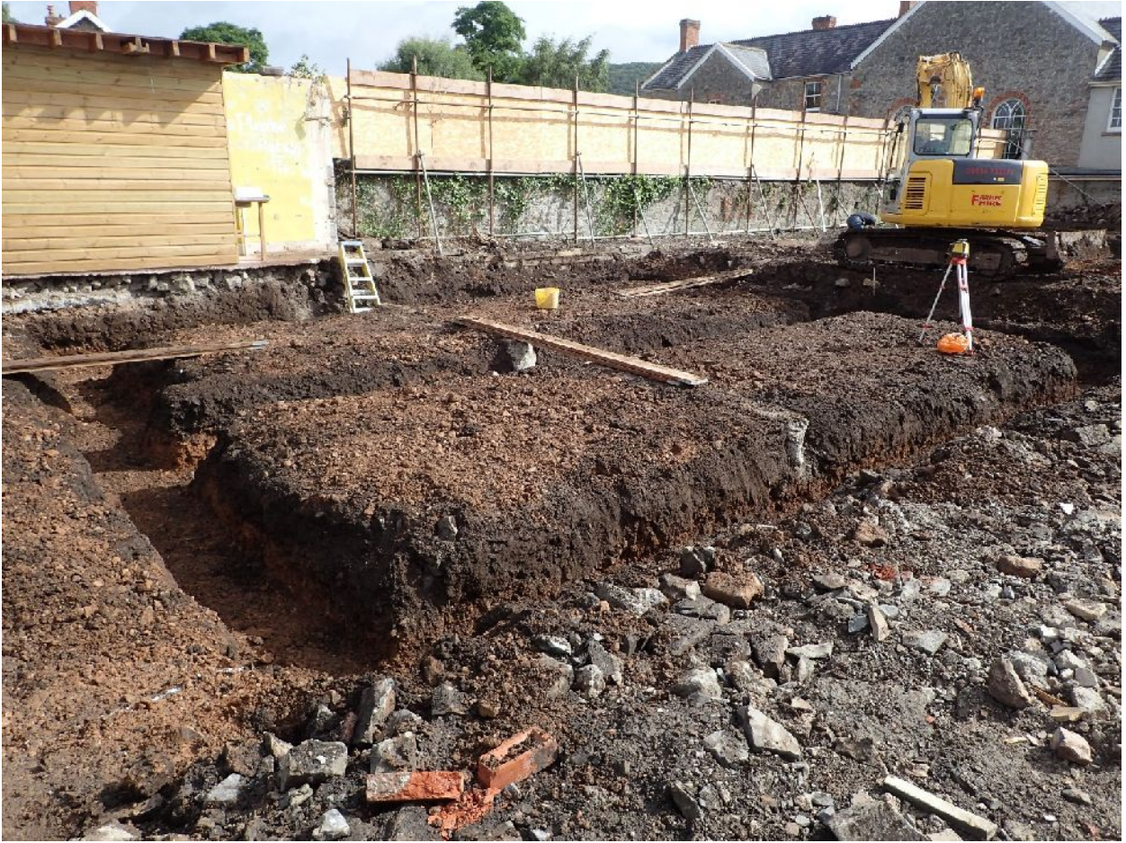
Plate 1. Excavated footings (facing NE)
