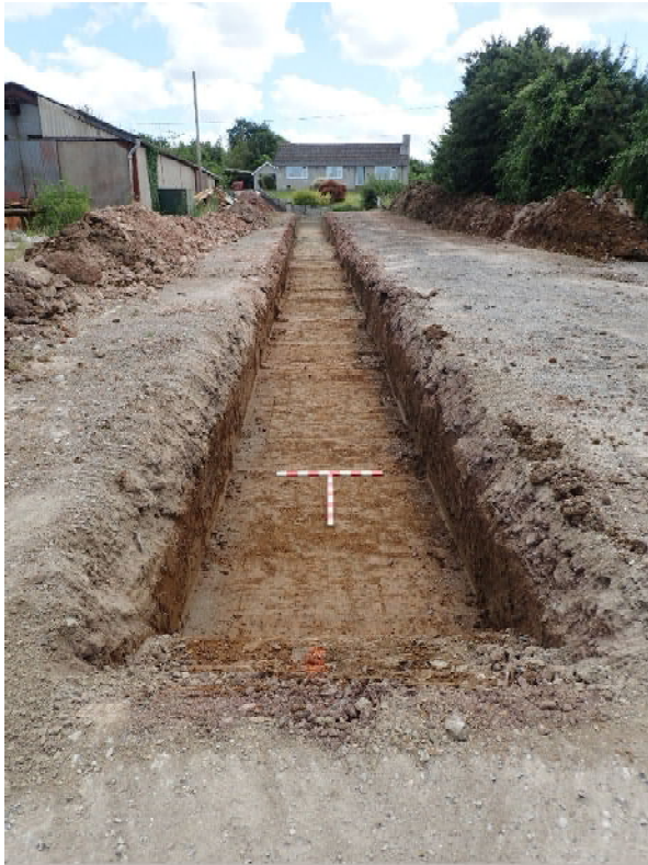
Plate 1. Trench 1 excavated (from NNE, 2 x 1m scales)
