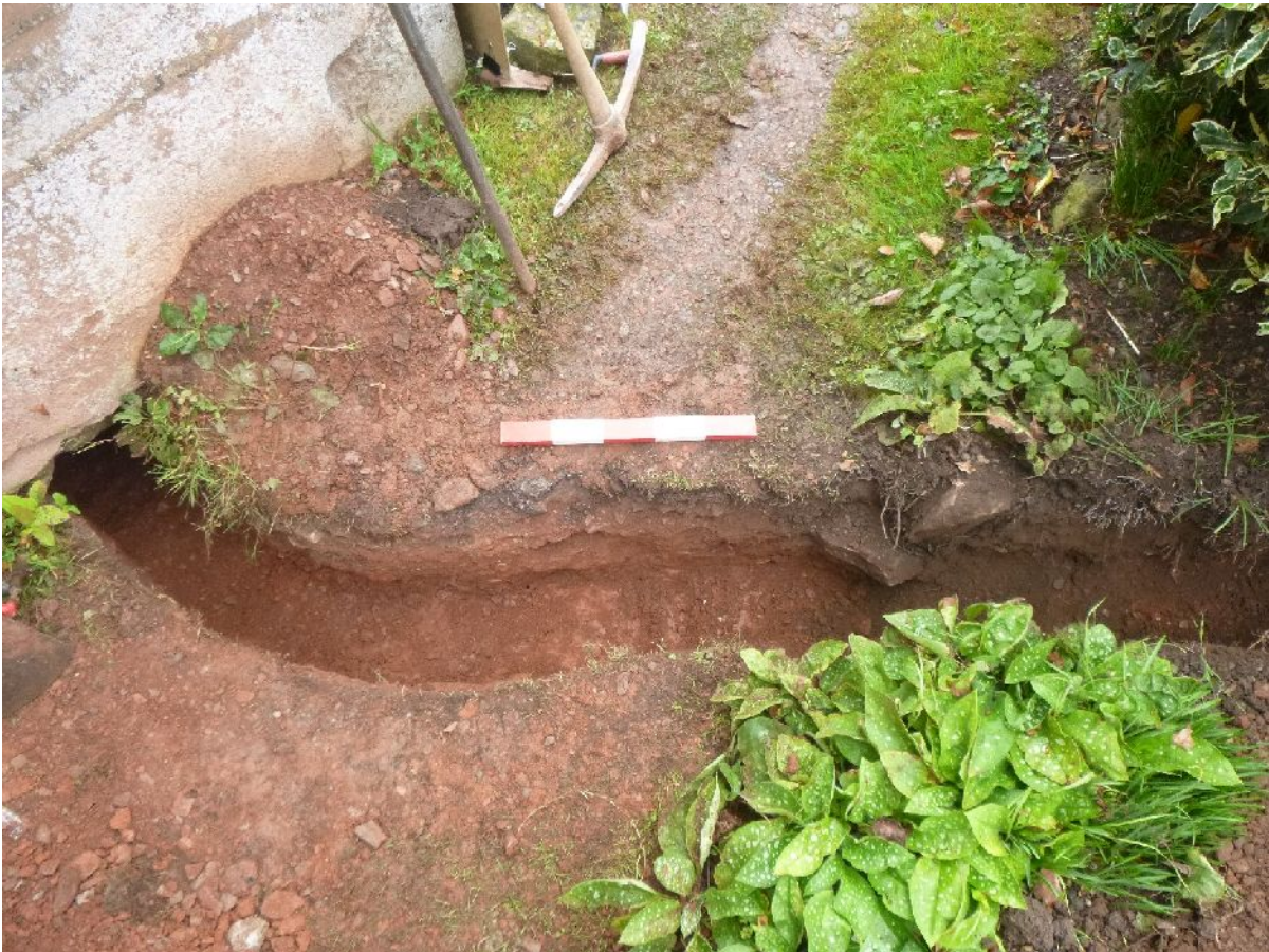
Plate 3. Exterior pipe trench (facing S; 0.50m scale)
