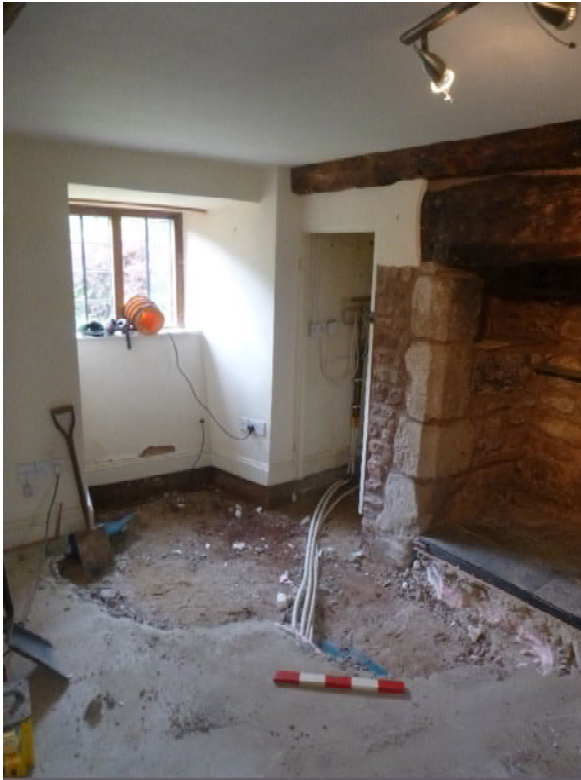
Plate 1. Interior works (facing SW; 0.50m scale)
