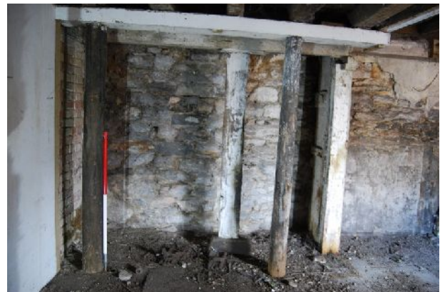
Plate 19. Wall A ground – rubble walling (from N)
