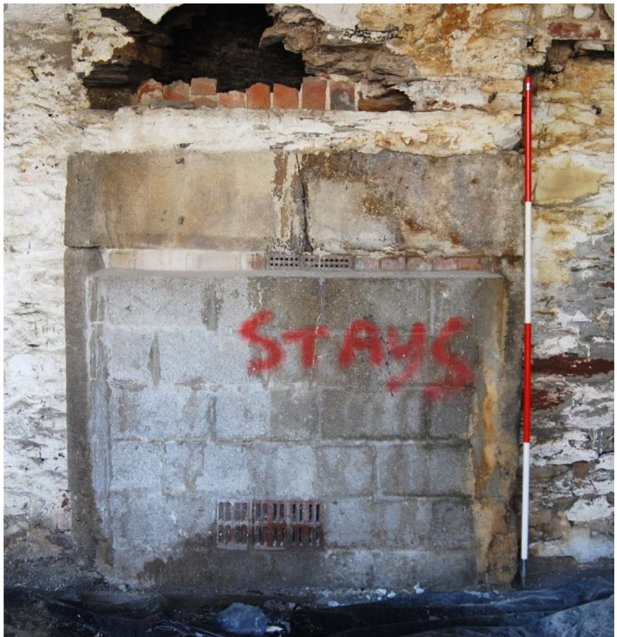
Plate 3. B1 Wall A - late 16 th to mid-17 th century fireplace (from N)
