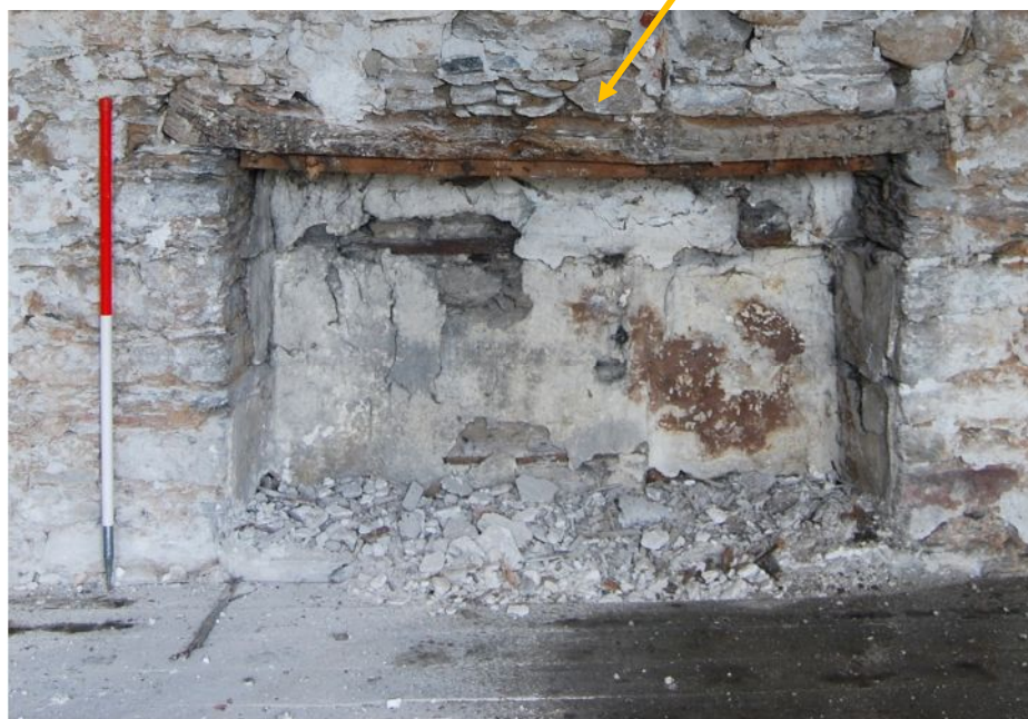
Plate 9. B1 Wall A first floor – blocked window
