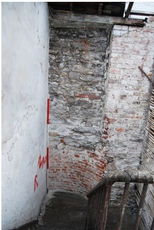
Plate 11. B1 Wall from second floor – stair turret (from N)
