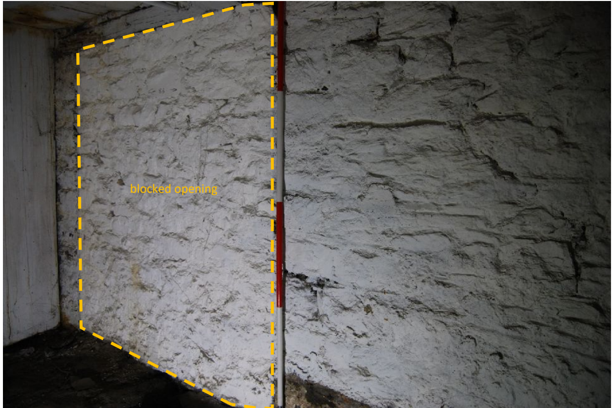
Plate 20. B2 east wall – rubble walling with blocked opening (from SW)
