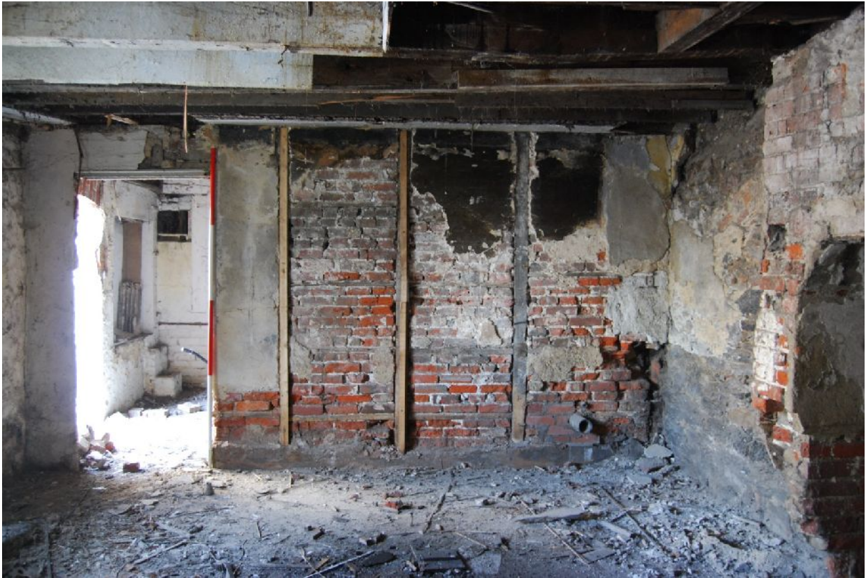
Plate 17. B2 ground – brick partition between rooms (from W)
