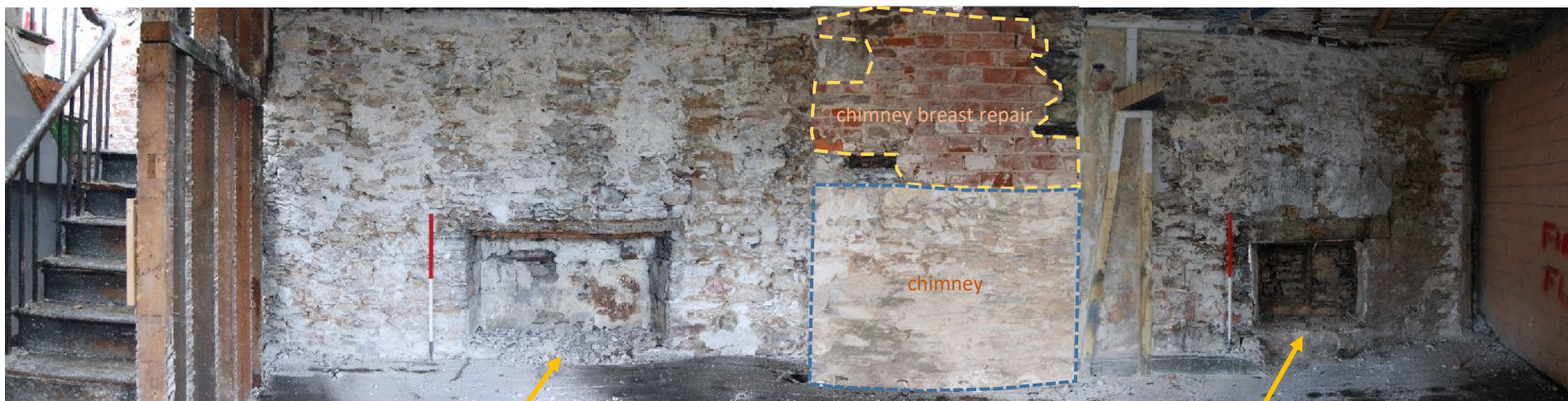
Plate 8. B1 Wall A first floor
