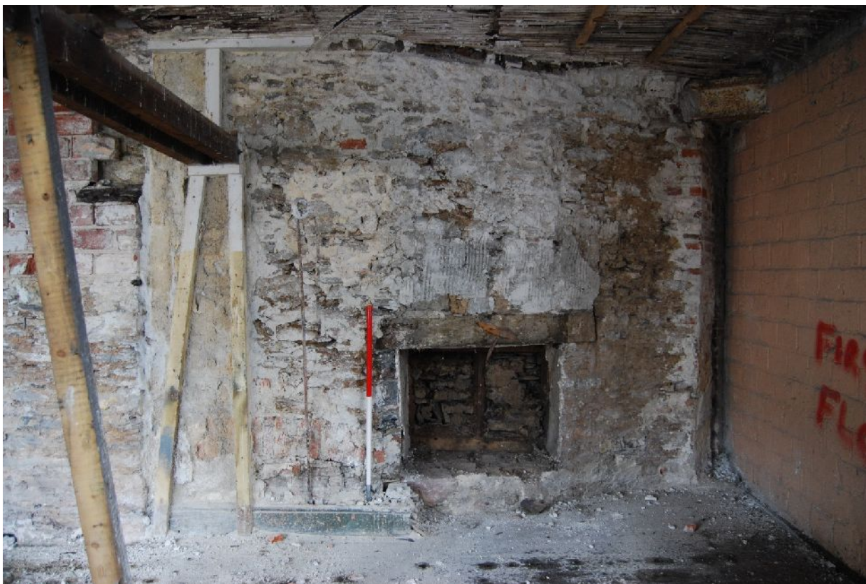
Plate 12. B1 Wall A first floor – west end (from N)
