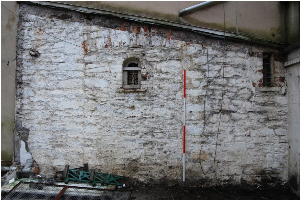
Plate 21. No. 98 east wall – blocked opening & two 17 th / 18 th century windows (from W)
