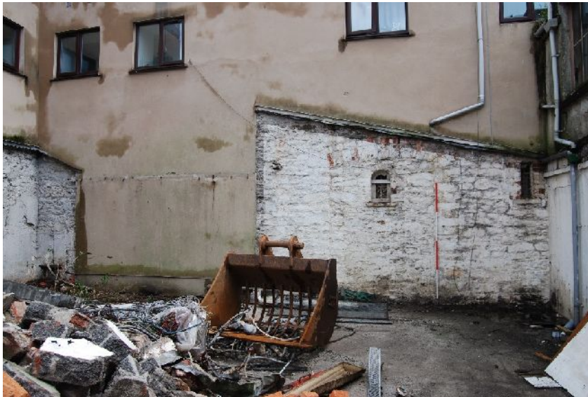
Plate 22. No. 98 east wall below Dolphin House with western return (from W)
