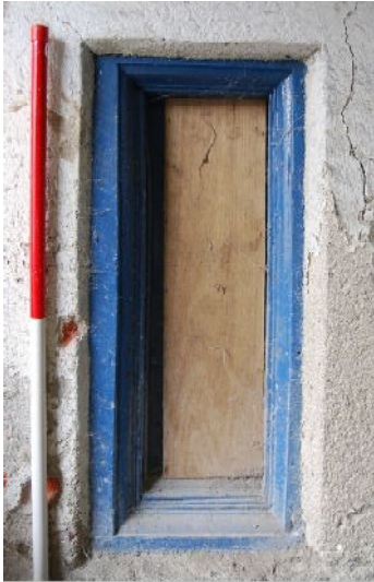
Plate 2. B1 north wall - 17 th century window (from N)
