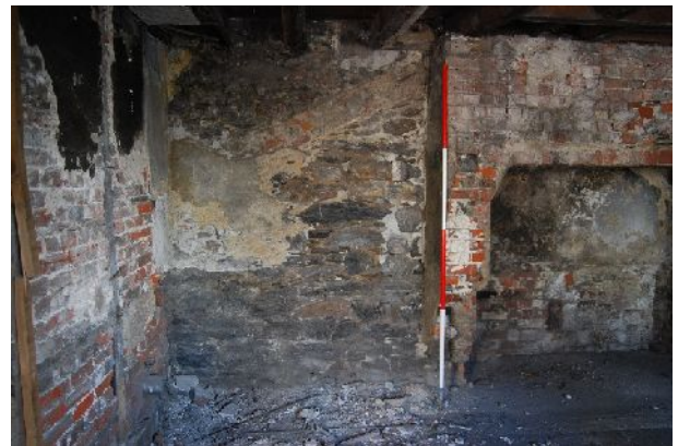
Plate 16. B2 Wall A ground – brick flue to east of fireplace (from N)
