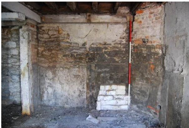
Plate 18. Wall A ground – rubble walling & stove setting across corner (from N)
