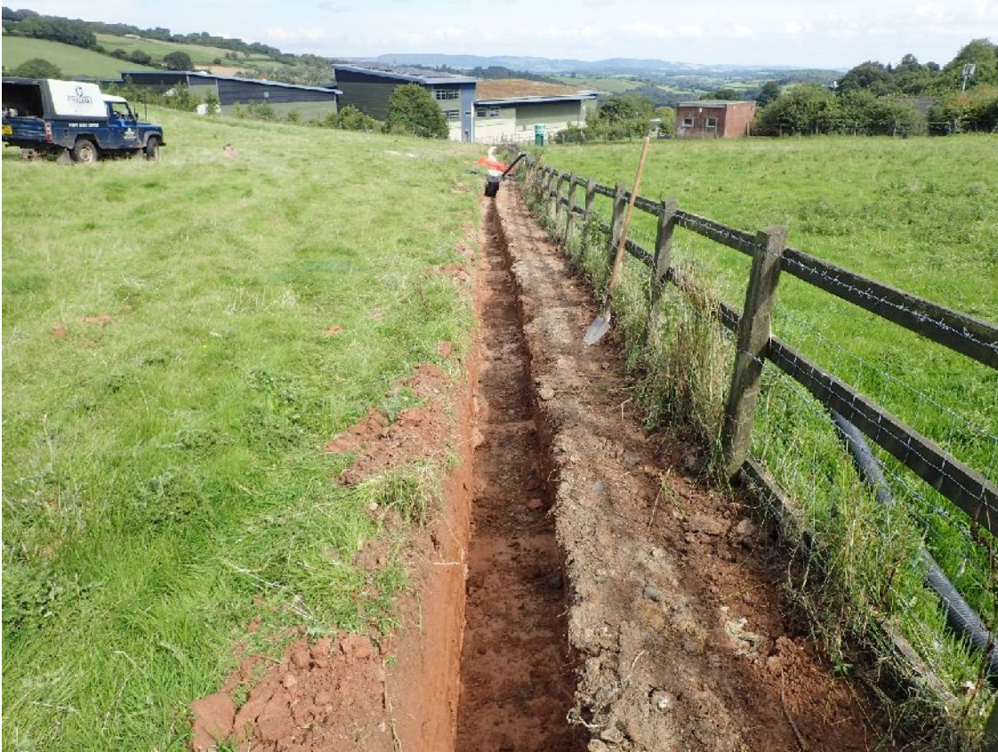
Plate 1. Land drain (facing NE)
