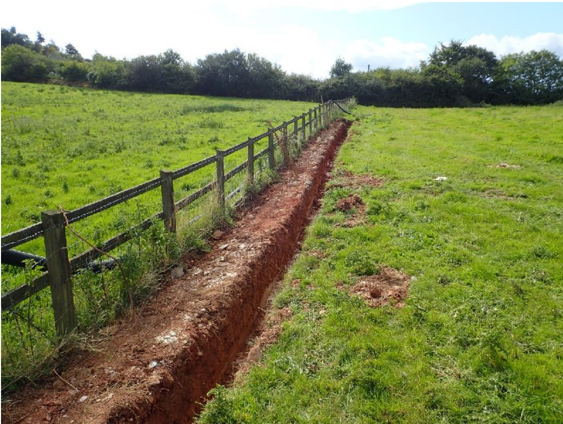
Plate 2. Land drain (facing SW)
