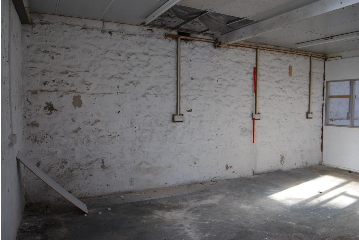
Figure 25. Ground floor of building A (2m scale, looking SW)
