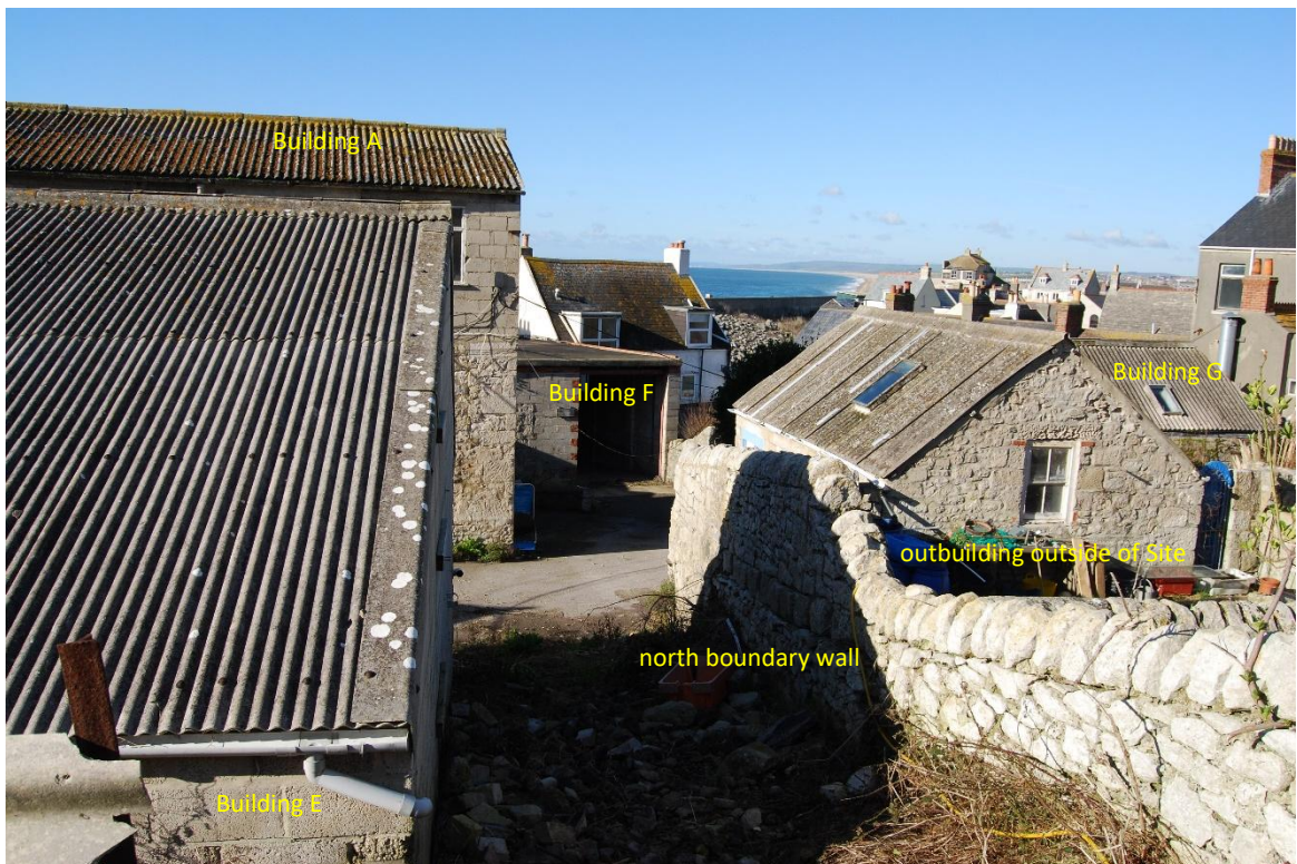
Figure 17. Stone boundary wall along north side of Site (looking W)
