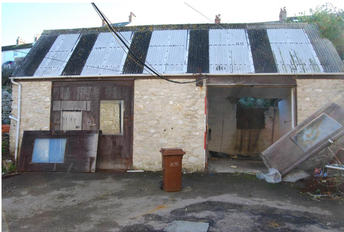
Figure 28. Building E (2m scale, looking E)
