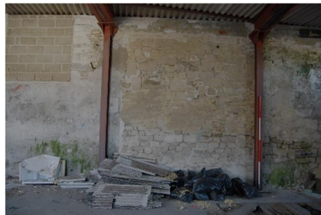
Building F – south wall
