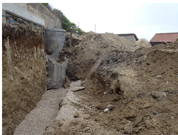
Figure 34. Deep piling alongside E boundary wall (looking S)
