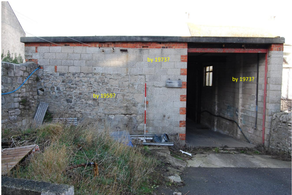
Figure 14. East end of Building F opening onto yard with extended mid-C20 north wall & east wall (2m scale, looking W)
