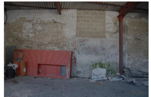
Building F – south wall
