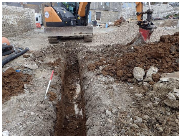
Figure 32. Excavation of trench (1m scale, looking N)
