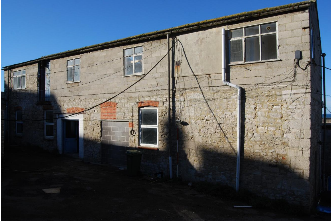
Figure 21. East elevation of building A (2m scale, looking WSW)
