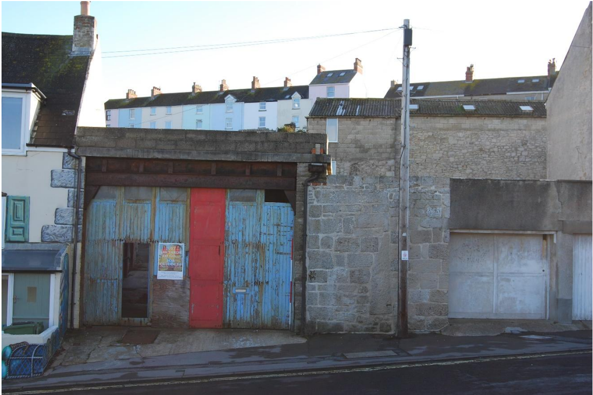
Figure 11. Access to Site from Brandy Row (2m scale, looking E)
