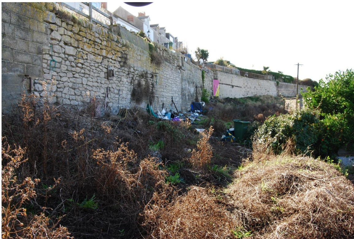
Figure 18. East retaining wall (looking S)
