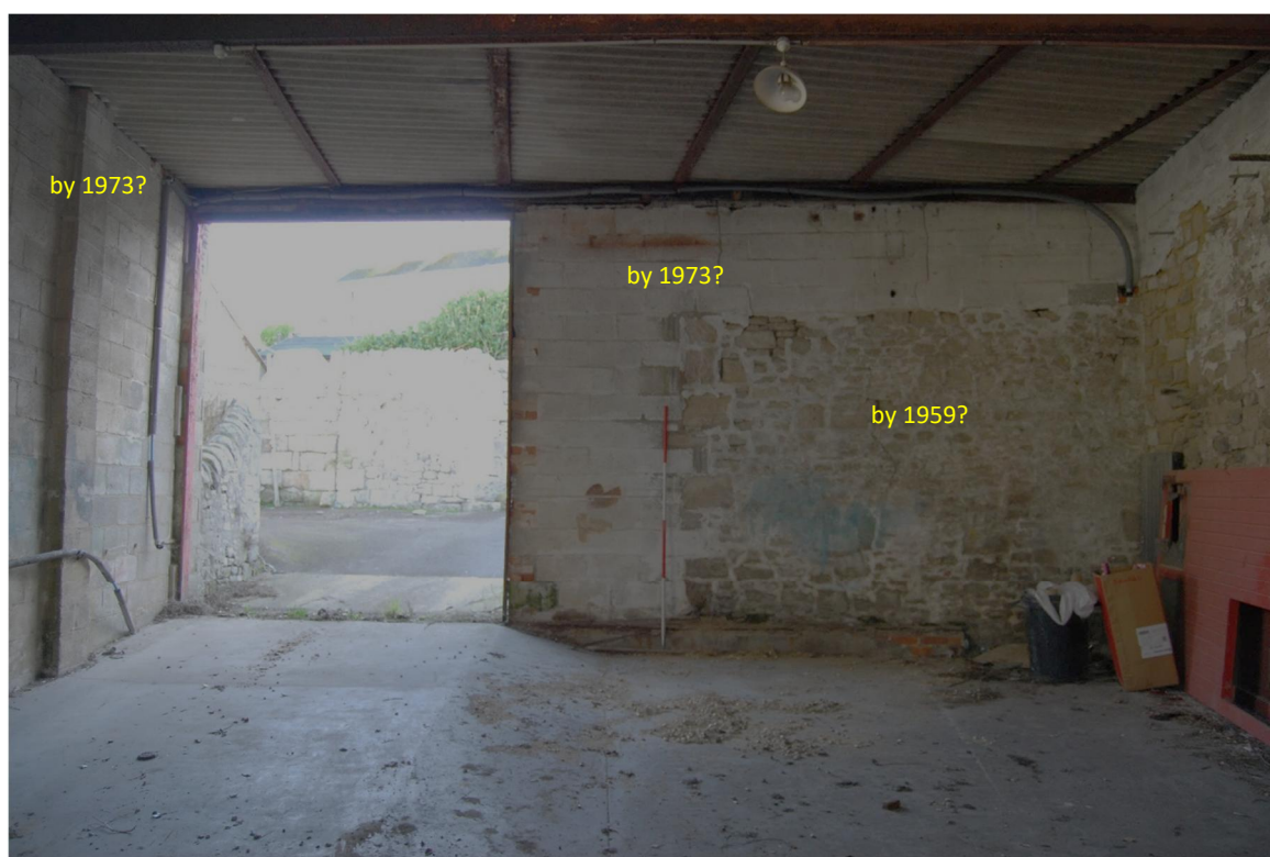
Figure 13. Building F with extended mid-C20 north wall & east wall (2m scale, looking E)
