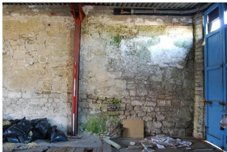
Building F – south wall
