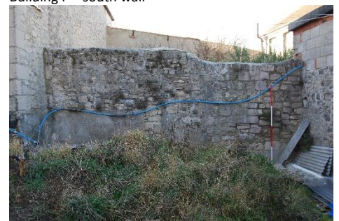
Boundary between building F & building A (looking S)
