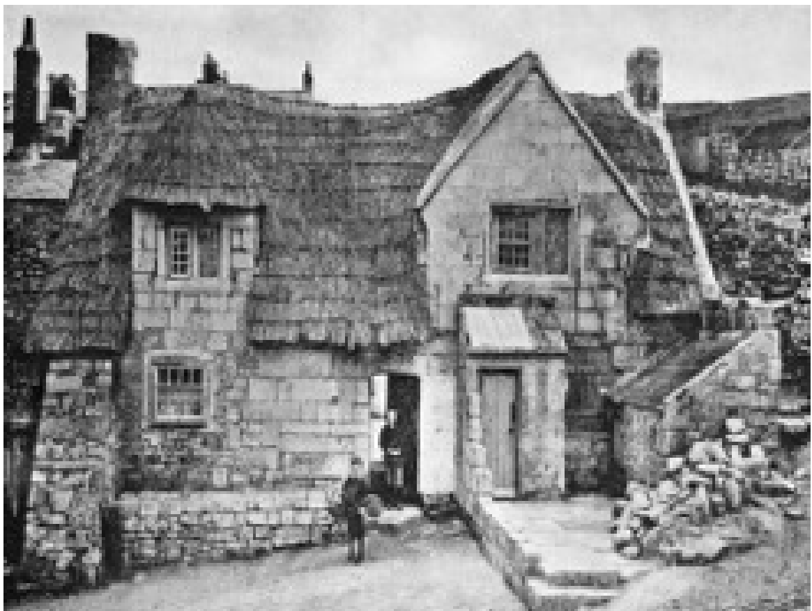
Figure 4. Photograph showing cottage with thatched dormer & buttress near south end of Brandy Row
