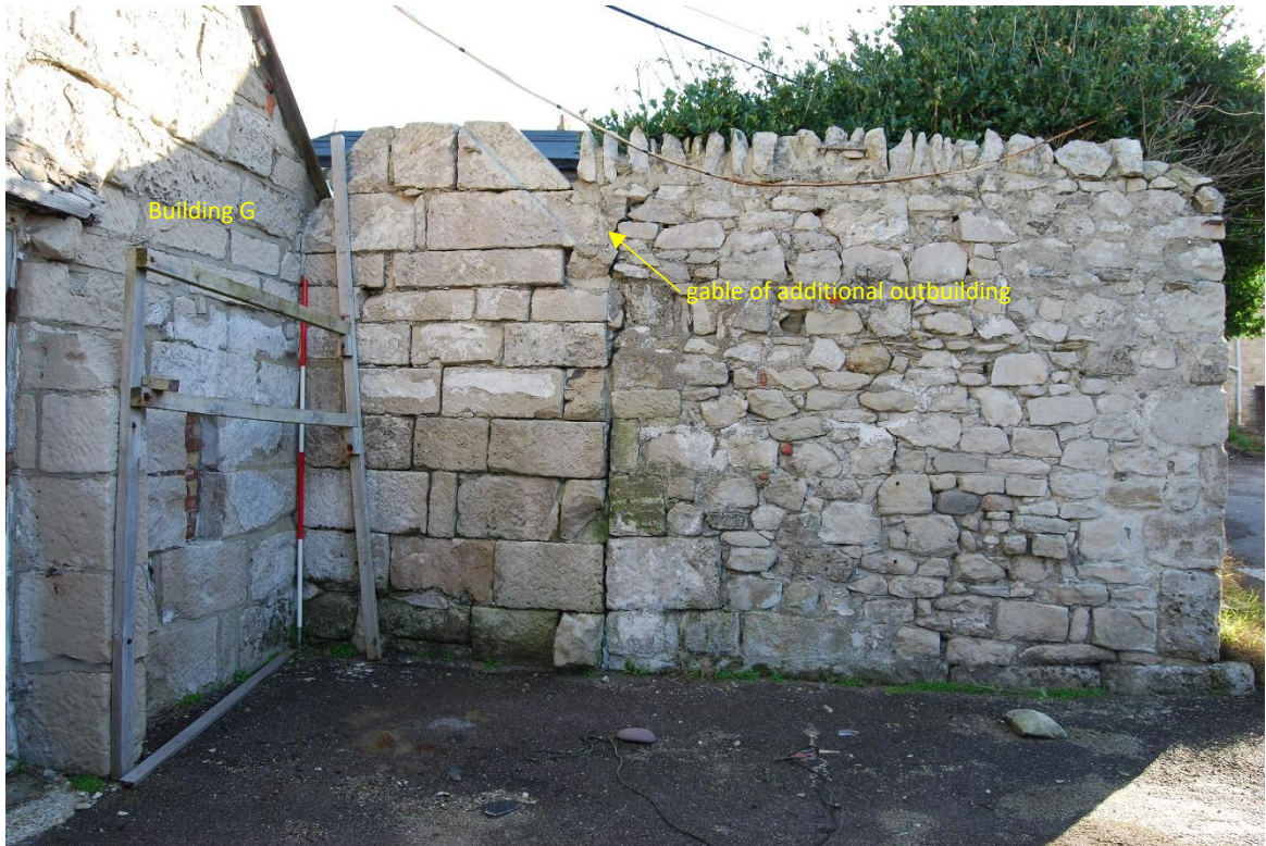
Figure 16. Building G with additional building to S (2m scale, looking E)
