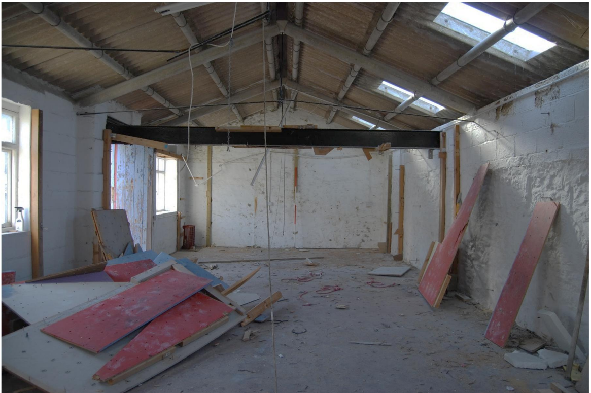
Figure 22. Upper storey of building A (2m scale, looking S)
