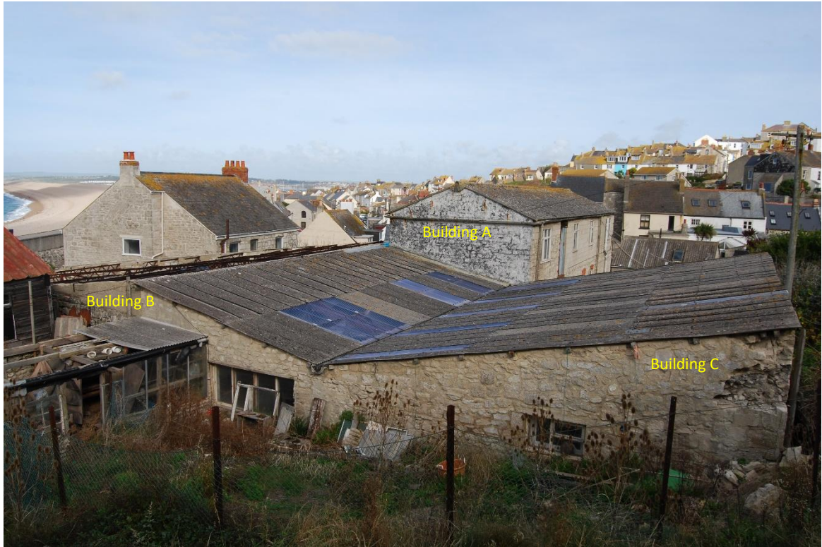
Figure 9. General view of buildings from S side of Site (looking N)
