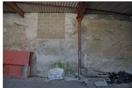
Building F – south wall
