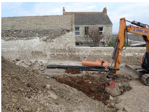
Figure 31. Excavation of trench (looking W)
