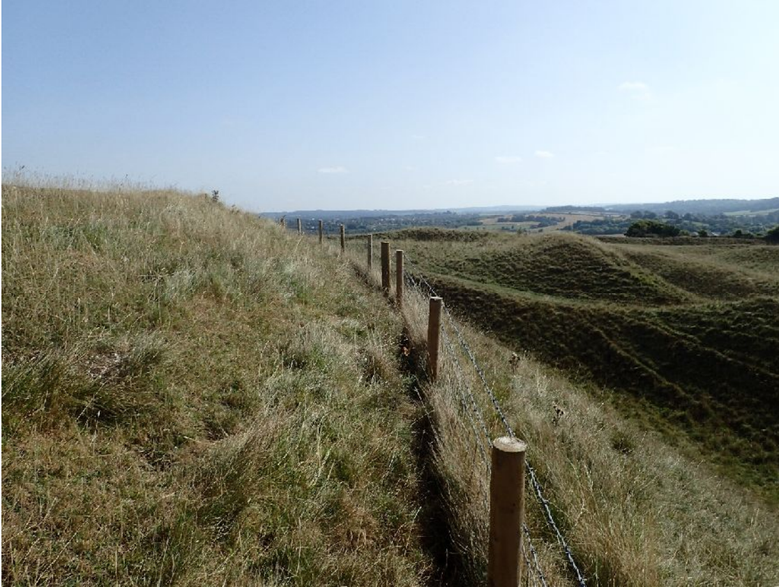
Plate 1. Replacement fence on same alignment as original (facing E)
