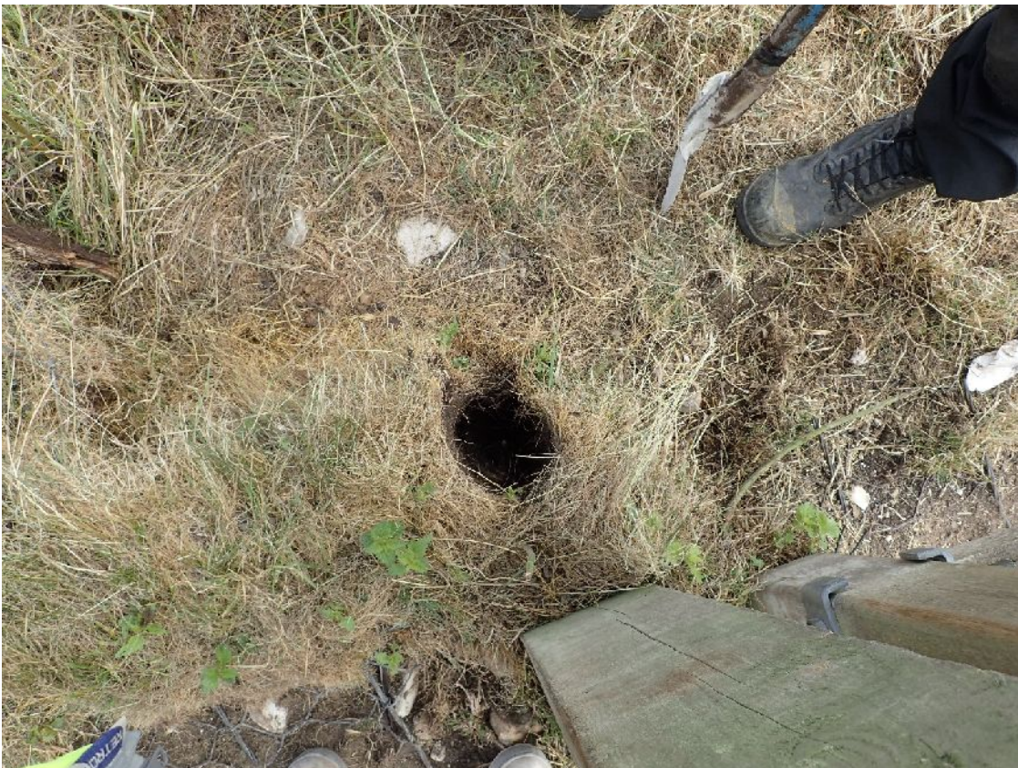
Plate 2. Post-hole after withdrawing existing post (vertical view)
