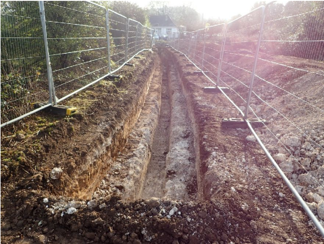
Plate 2. Pipe trench (facing NW)
