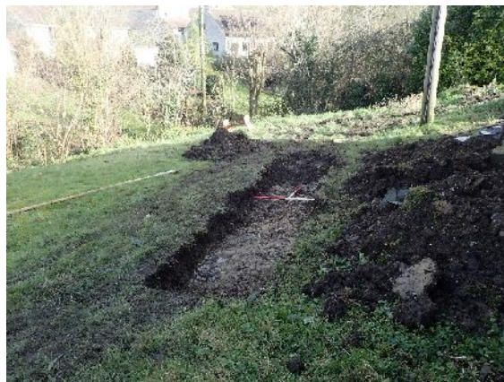
Plate 2. Excavated trench (from SW; 2 x 1m scales)
