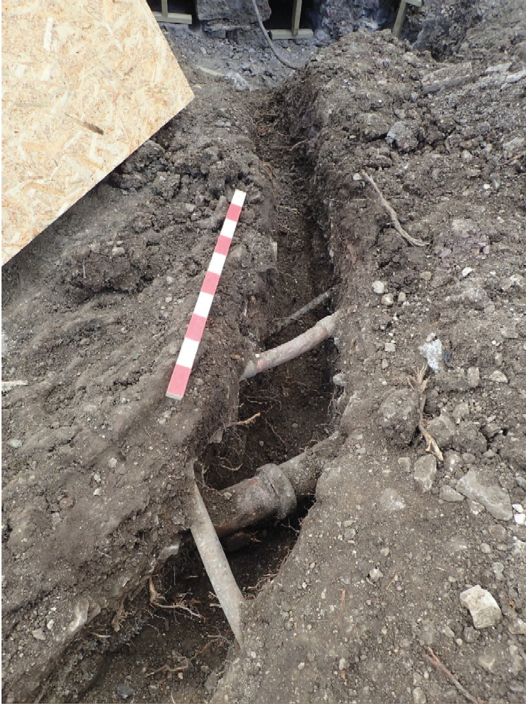
Plate 1. Electric cable trench (facing W; 1m scale)
