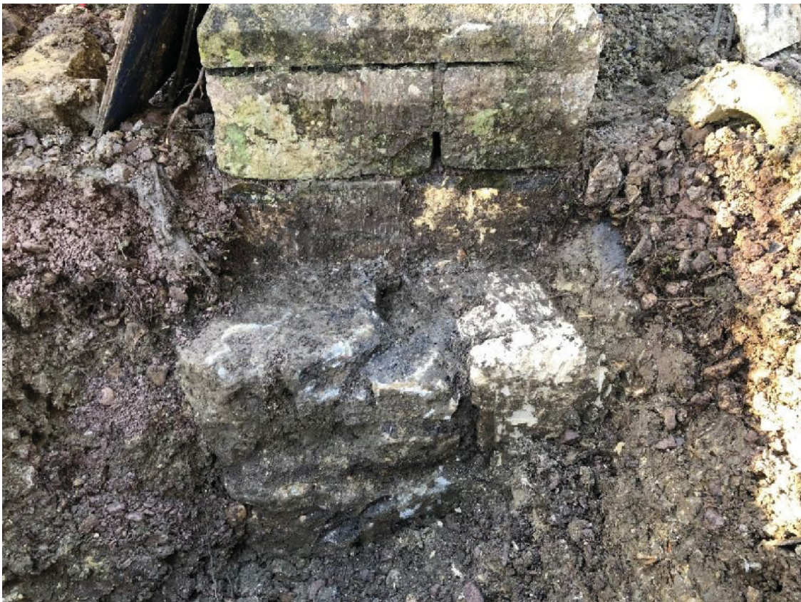
Plate 3. North-east corner buttress with projecting foundation (facing SW)
